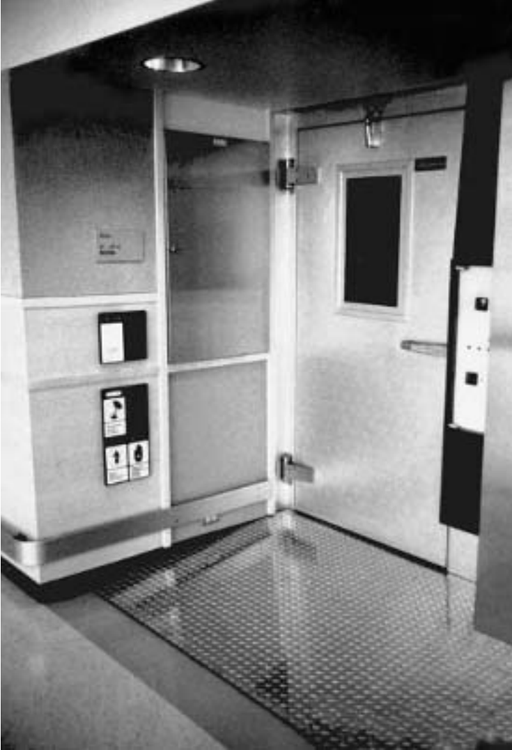
▲ Entry into a modular cold room.
