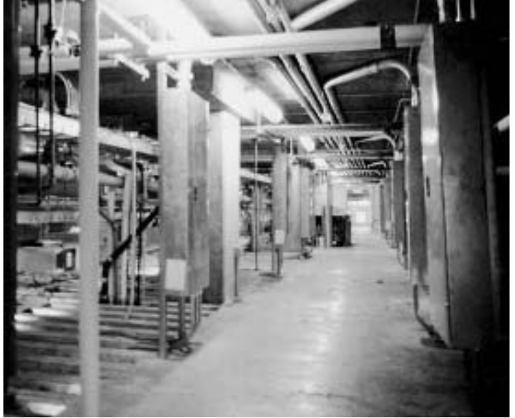
▲ Partial Interstitial space. NIH Building 40, Bethesda, Maryland. HLM, architect.
