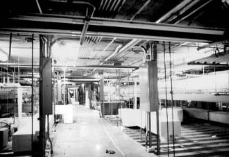
◀ Partial interstitial space. NIH Building 40, Bethesda, Maryland. HLM, architect. Courtesy NIH.
