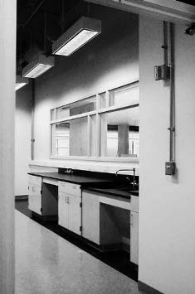
▲ Location of light fixtures in relation to casework. Manufacturing Related Disciplines Complex, Phase II, Georgia Institute of Technology, Atlanta. Perkins & Will, architect.
