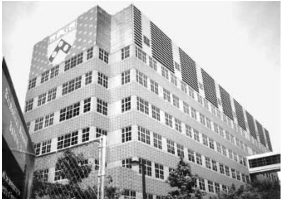
▶ Clinical Research Building, University of Pennsylvania, designed and constructed more than 10 years after Thomas Laboratories at Princeton. Venturi Scott Brown with Payette & Associates, Inc., architect.
