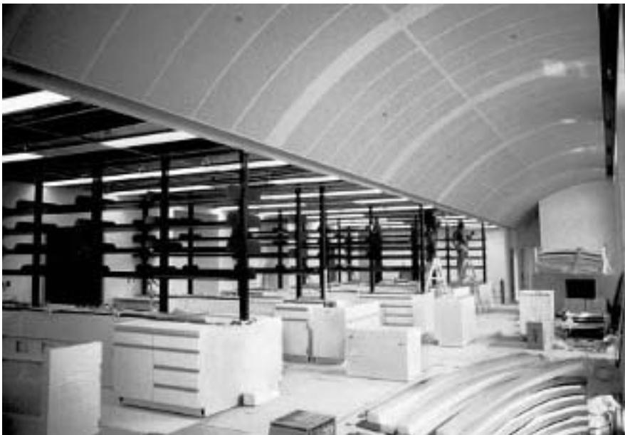
▲ Partial Interstitial space. NIH Building 40, Bethesda, Maryland. HLM, architect.
