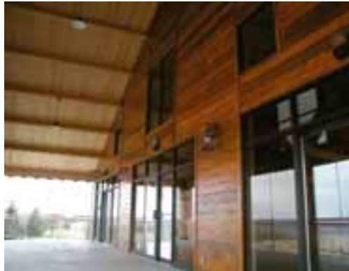
Figure 22 Wide overhang shelters the verandah
