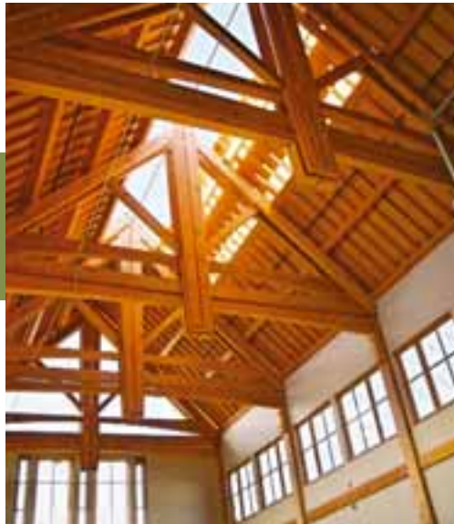
Figure 30 Bright, open roof structure in the main entry
