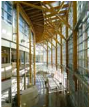
Figure 33 Glulam structure provides a bright, roomy atmosphere for the main public corridor
