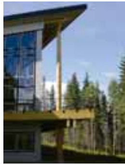
Figure 8 Exterior, north side
