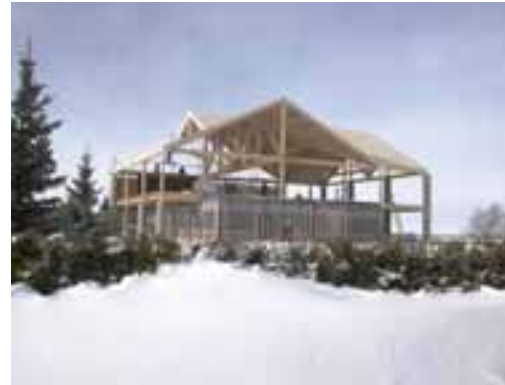
Figure 23 Structural frame during construction
