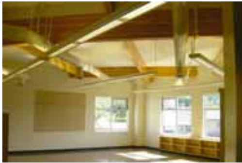
Figure 18 Typical classroom (before furnishing) showing roof structure and views to the exterior
