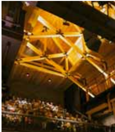
Figure 13 Auditorium roof structure
