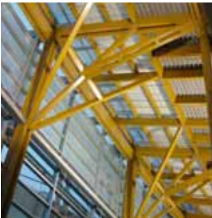
Figure 34 Detail of the glulam roof trusses and struts
