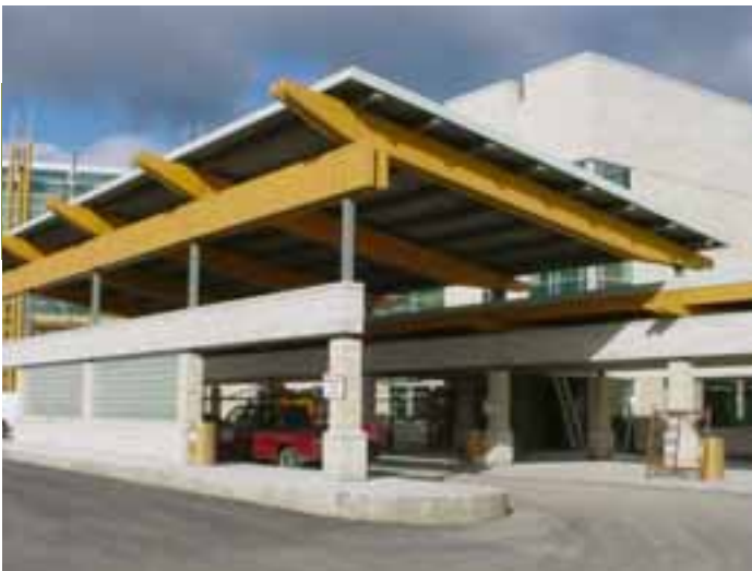
Figure 36 Glulam entrance canopy
