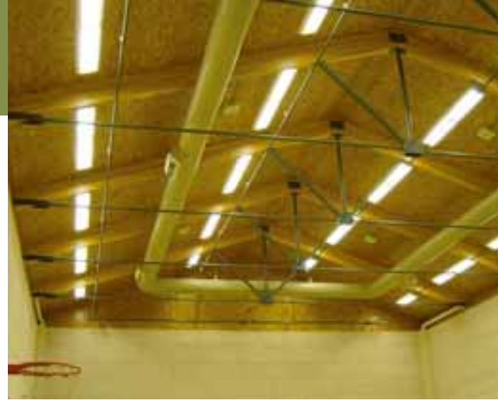
Figure 20 View of the glulam-tied roof, lighting and ventilation
