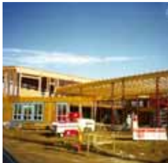
Figure 26 Wood structure during construction
