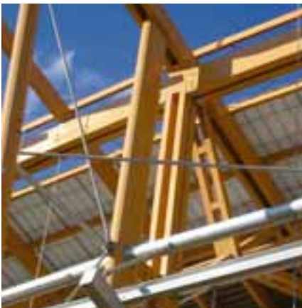
Figure 35 Timber connectors and tie rods
