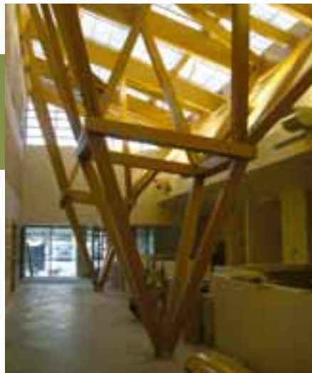
Figure 37 Glulam support structures in the cancer treatment centre
