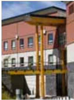
Figure 7 Main entry bridge
