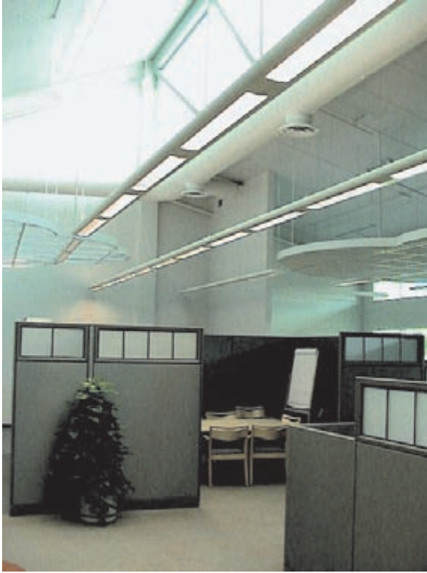
Figure 3-3. A sensor measures the amount of natural light coming in and adjusts overhead fluorescent lights accordingly.
