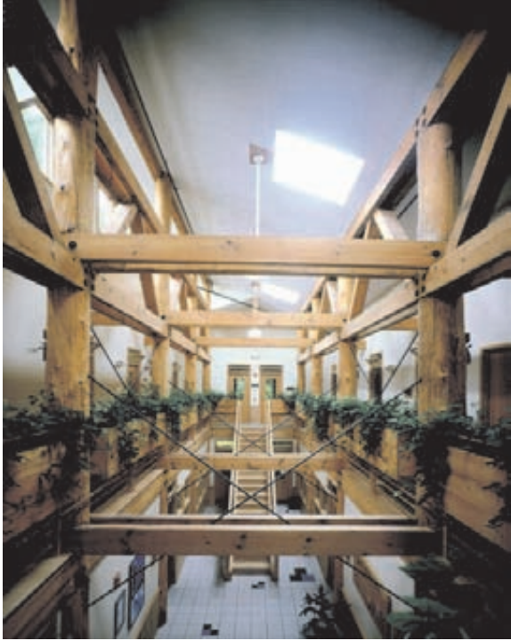
Figure 3-22. North-facing skylights illuminate the French Wing's corridor.
