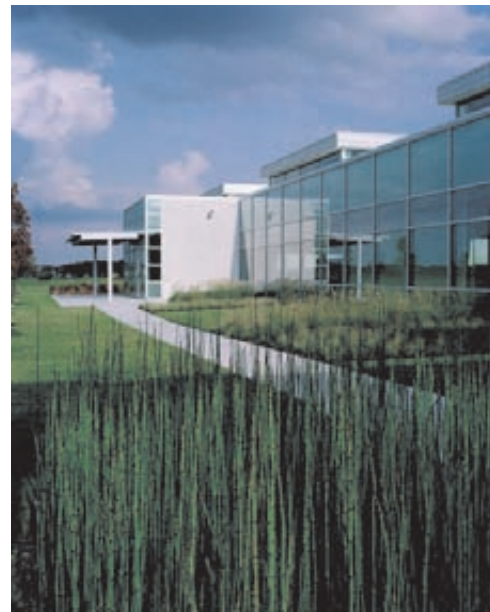
Figure 3-9. Native plants, a low planting density, and a weather-monitoring device were installed to help reduce demand for landscape irrigation.
