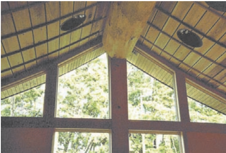
Figure 3-17. Skylights and windows provide an aggregate of twice the already stringent Oregon code standards for energy efficiency.
