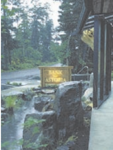
Figure 3-14. Water from the roof is discharged through a scupper into a landscaping pond for storage and settling before the water is reabsorbed into sandfill below.
