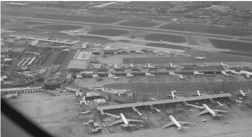
Figure 7-7 Pier system at London Heathrow Airport (Photo: A. Kazda)
