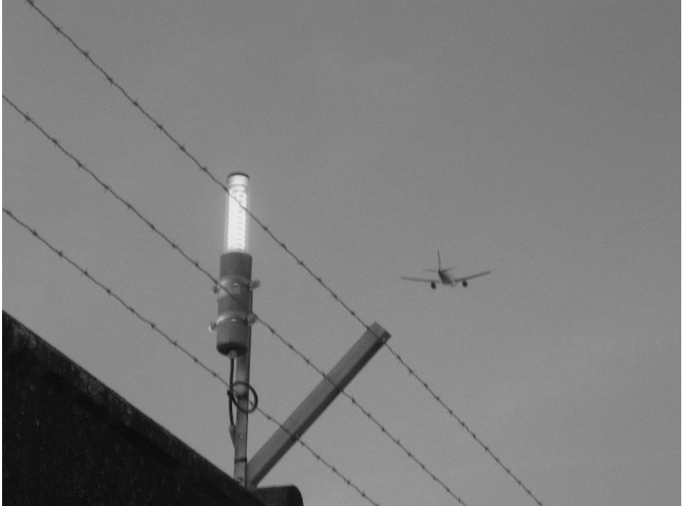
Figure 15-22 Low intensity neon obstacle light, (Photo: M. Ma'aš)
