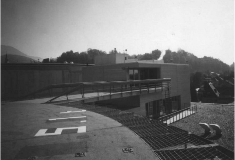
Figure 18-8 Electrically heated pavement - emergency heliport on the roof of the regional hospital at Salzburg, (Photo: A. Kazda)
