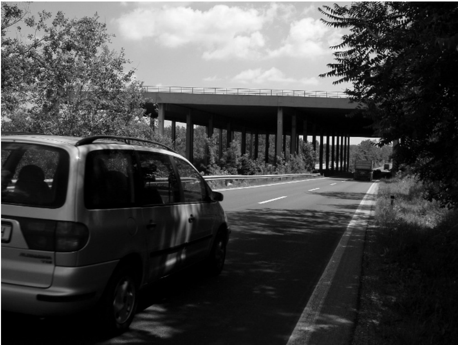
Figure 5-2 Large constructions are sometimes necessary to guarantee runway strip dimensions – Vienna Airport (Photo: A. Kazda)
