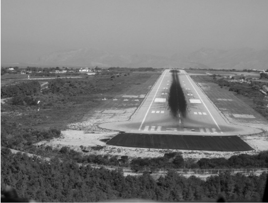
Figure 4-15 Turn pad at the runway end
