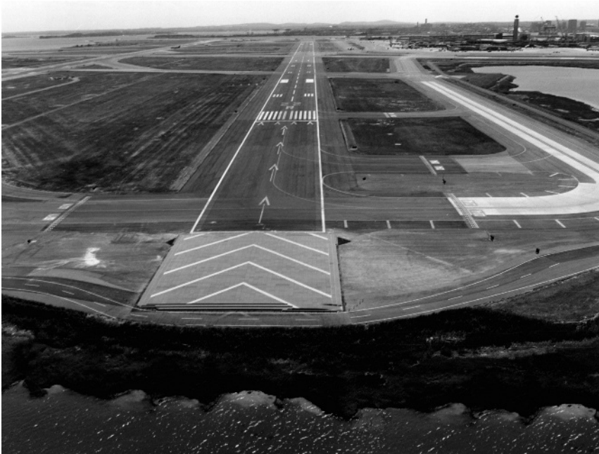
Figure 5-5 EMAS installation at Boston Logan Airport, courtesy ESCO ZODIAC Company (Photo: David J. Heald, C.M.)
