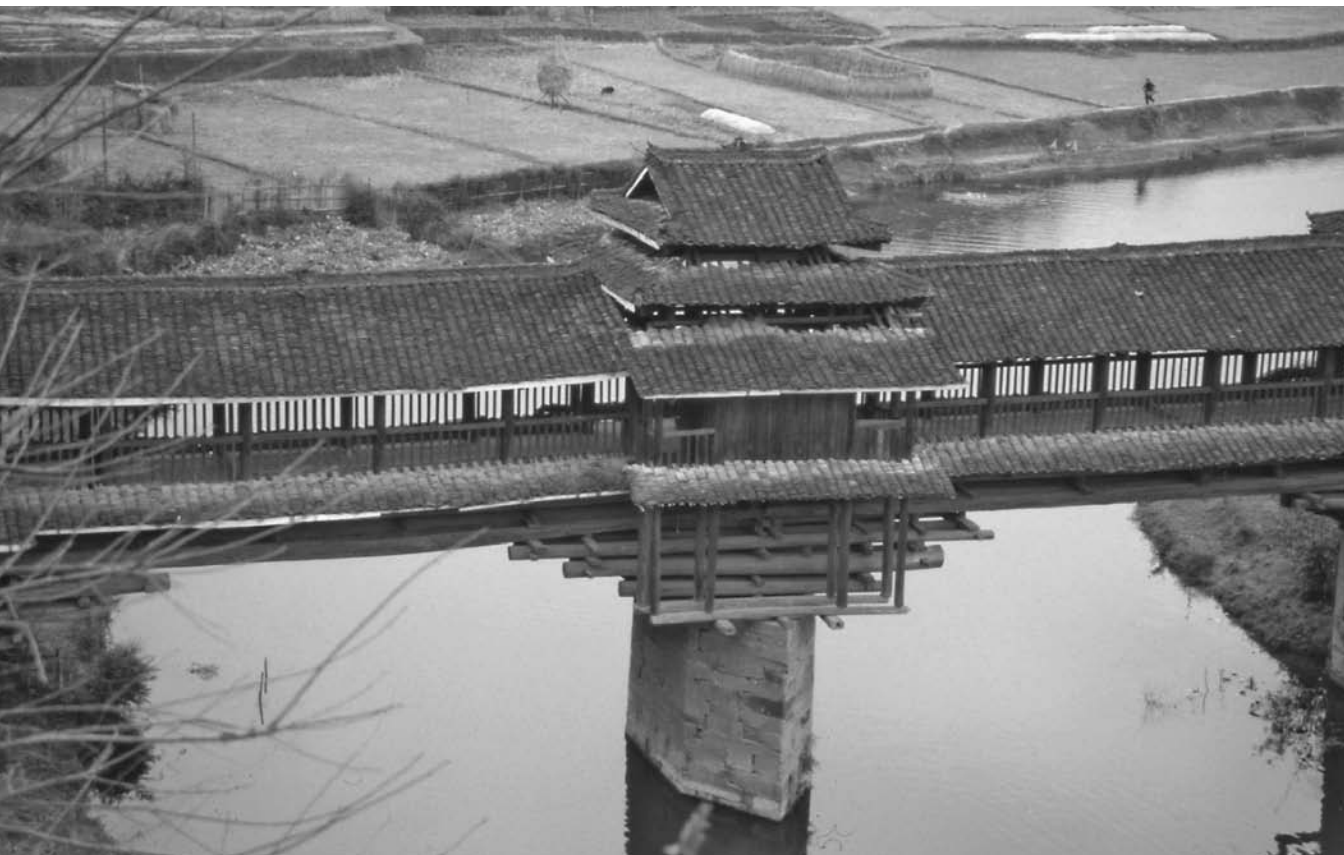
Figure 2.57 A close view of the Pingyan wind-and-rain bridge in Ma'an village, Sanjiang region, Guangxi province. Source: Photograph by Xing Ruan, 1992.
