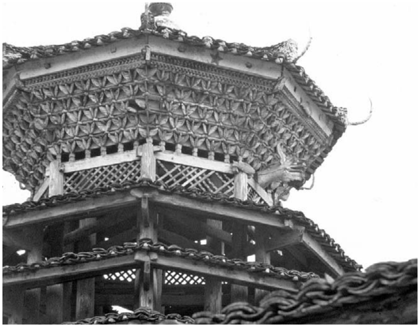
Figure 3.15 The top drum pavilion of the Xindi village drum tower is supported by dougong . Congjiang region of Guizhou province. Source: Photograph by Xing Ruan, 1993.
