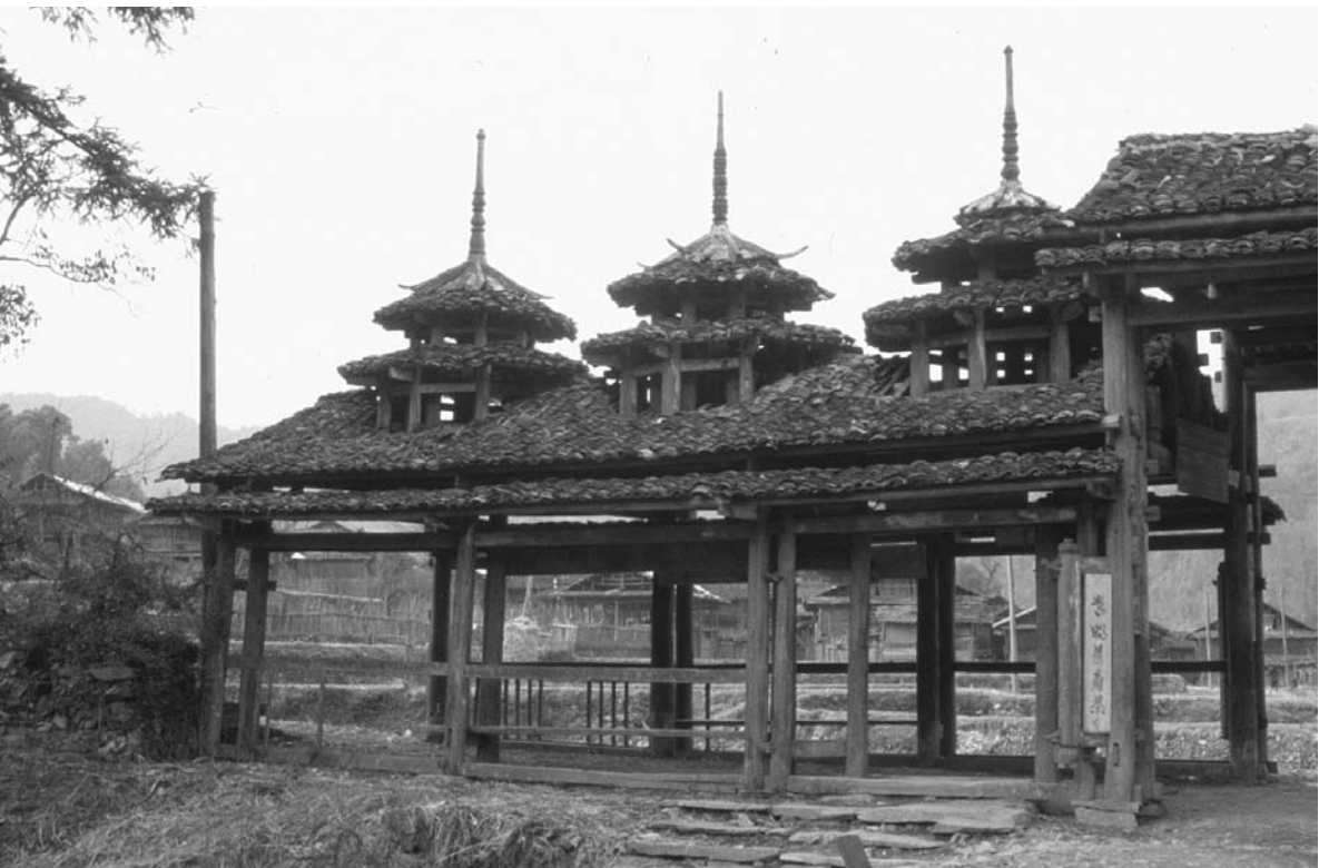
Figure 2.28 The Xindi village gate of the Congjiang region is a combination of gate, roadside pavilion, and wind-and-rain bridge. Source: Photograph by Xing Ruan, 1993.
