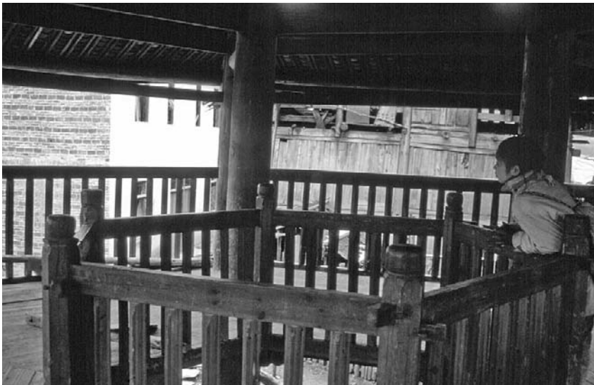
Figure 3.25 a and b In Heli village of the Sanjiang region, Guangxi province, the inhabited level of one drum tower ( top ) is elevated above the ground ( bottom ). Source: Photograph by Xing Ruan, 1992.
