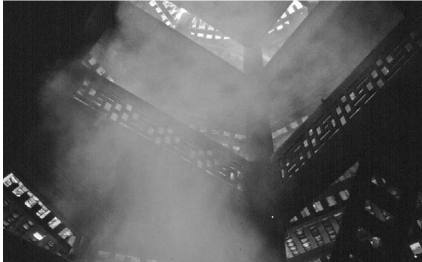
Figure 5.1 Smoke from the fire pit in the Zengchong drum tower accelerates the ageing of the timber frame. Congjiang region, Guizhou province. Source: Photograph by Xing Ruan, 1993.
