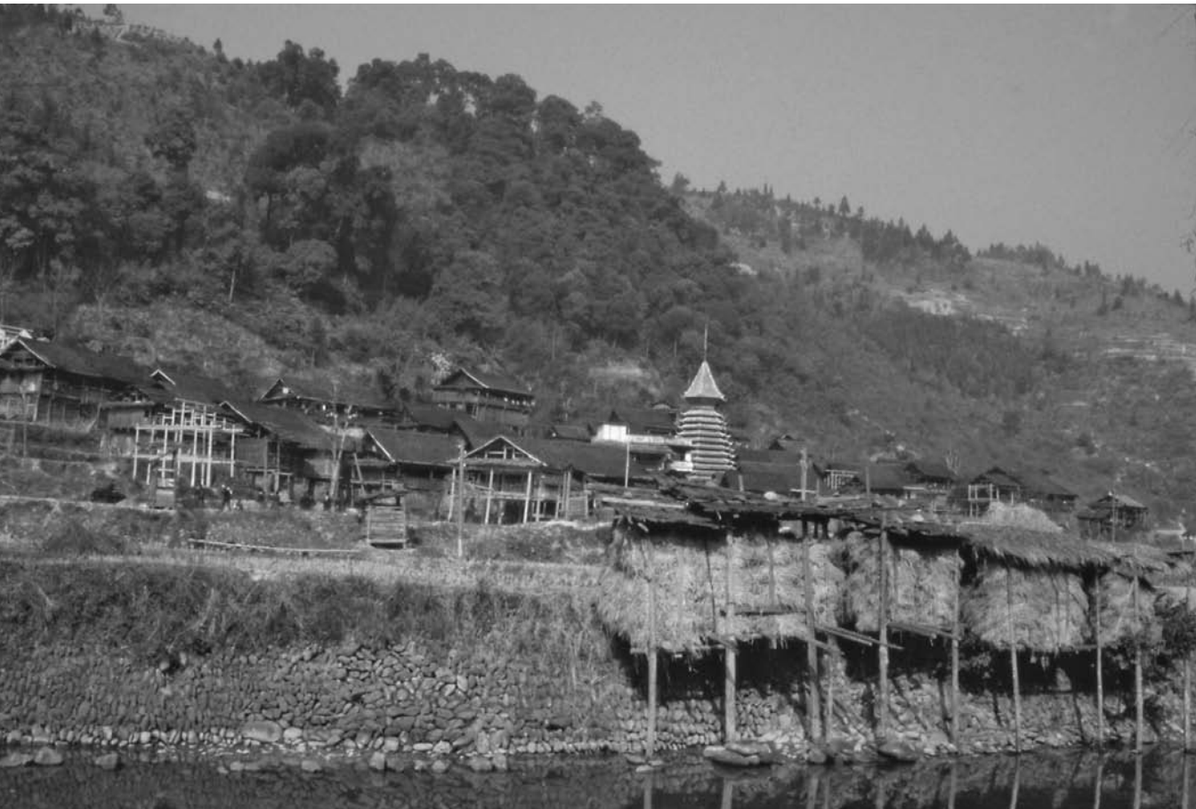
Figure 2.43 In Gaozeng village of the Congjiang region, pile-built granaries are grouped and separated from the village. Source: Photograph by Xing Ruan, 1993.
