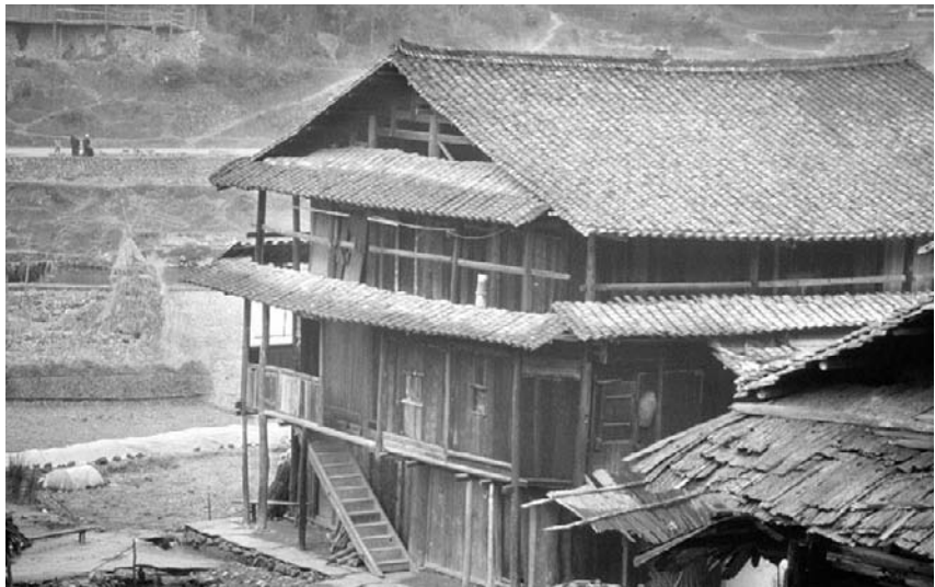
Figure 3.8 House in Ma'an village in the Sanjiang region, Guangxi province. The roof is typical of the gable-and-hip form across the whole Dong region. Source: Photograph by Xing Ruan, 1992.
