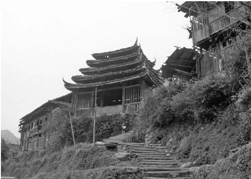
Figure 2.16 The drum tower of Zaimao village in the Sanjiang region, Guangxi province, a combination of gate and drum tower, stands at the village's edge. Source: Photograph by Xing Ruan, 1992.
