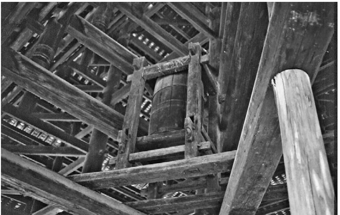
Figure 3.33 Since there is no top pavilion, the drum of the Mapang drum tower is placed on the main structural framework. Source: Photograph by Xing Ruan, 1992.
