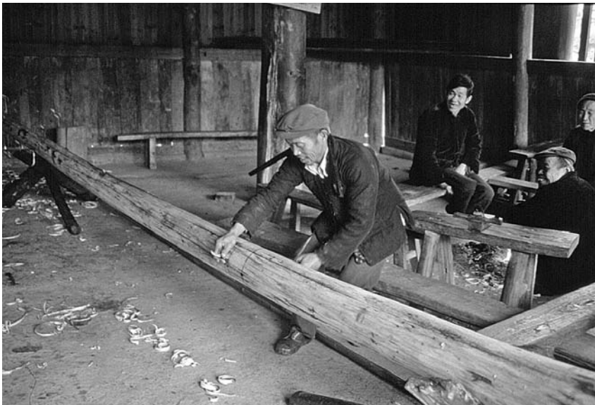
Figure 3.43 Tree trunks being worked into columns on stands. Ma’an village, Sanjiang region, Guangxi province. Source: Photograph by Xing Ruan, 1992.
