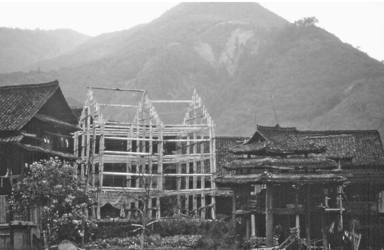
Figure 4.31 A new Dong house frame against the background of weathered houses in Pingyan village, Sanjiang region, Guangxi province. Source: Photograph by Xing Ruan, 1993.
