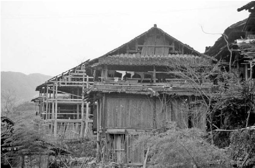
Figure 2.45 A house in Ma'an village of the Sanjiang region. Some frameworks of the house are left unfilled for drying rice paddies. Source: Photograph by Xing Ruan, 1989.
