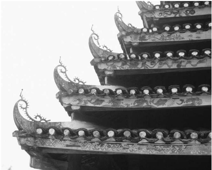
Figure 3.11a and b Many drum tower eaves are curved with distinctive snake or dragon features. Dong drum towers from ( top ) Zengchong village, Congjiang region in Guizhou province; ( bottom ) Mapang village, Sanjiang region in Guangxi province. Source: Photographs by Xing Ruan, 1993 and 1992.
