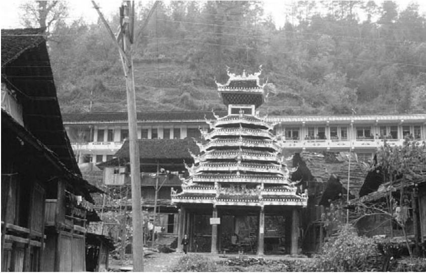
Figure 3.18 One of the five drum towers located in the central area of Zhaoxin village in the Liping region, Guizhou province. This is the only flat, gable-and-hip roof among the five drum towers, which is claimed to symbolically roof the “cabin” of the whole village “boat.” Two birds stand on the roof ridge. Source: Photograph by Xing Ruan, 1993.
