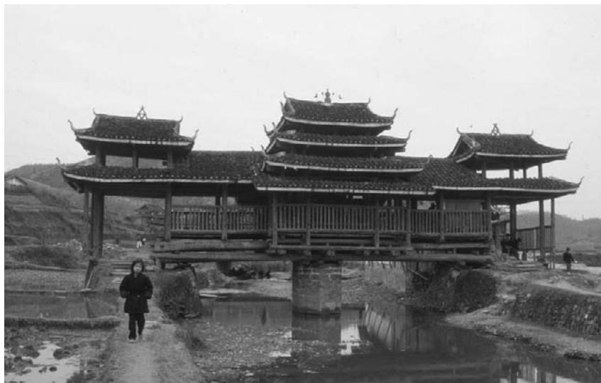
Figure 1.11 The Ouyang bridge in Heli village, Sanjiang region of Guangxi province, is a large-scale elaborate structure but spans only a small stream. Source: Photograph by Xing Ruan, 1992.
