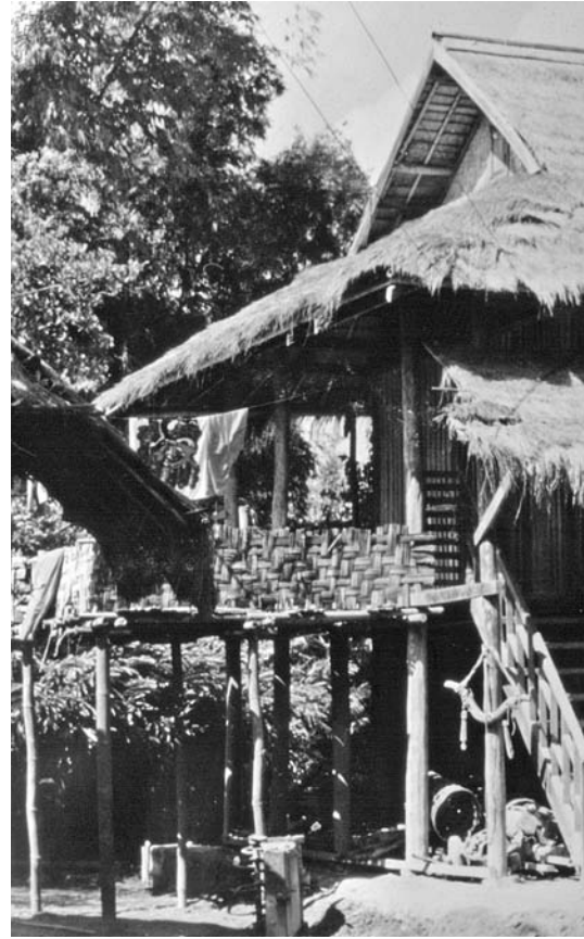
Figure 4.11 A gable-and-hip roof, pile-built Dai house in Ruili, Dehong region, Yunnan province. Source: Photograph by Xing Ruan, 1986.
