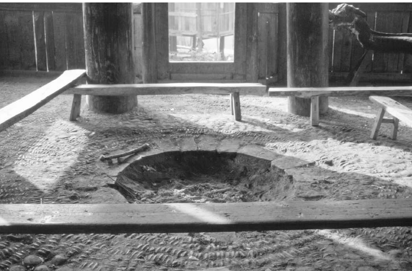
Figure 1.15 The interior of the lower pavilion in the Gaozeng drum tower, Congjiang region in Guizhou province, showing the central fire pit and long benches around it. Source: Photograph by Xing Ruan, 1993.
