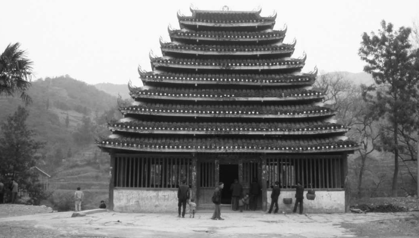
Figure 3.32 Front elevation of the Mapang drum tower, which has no pavilion loft. Sanjiang region in Guizhou province. Source: Photograph by Xing Ruan, 1992.
