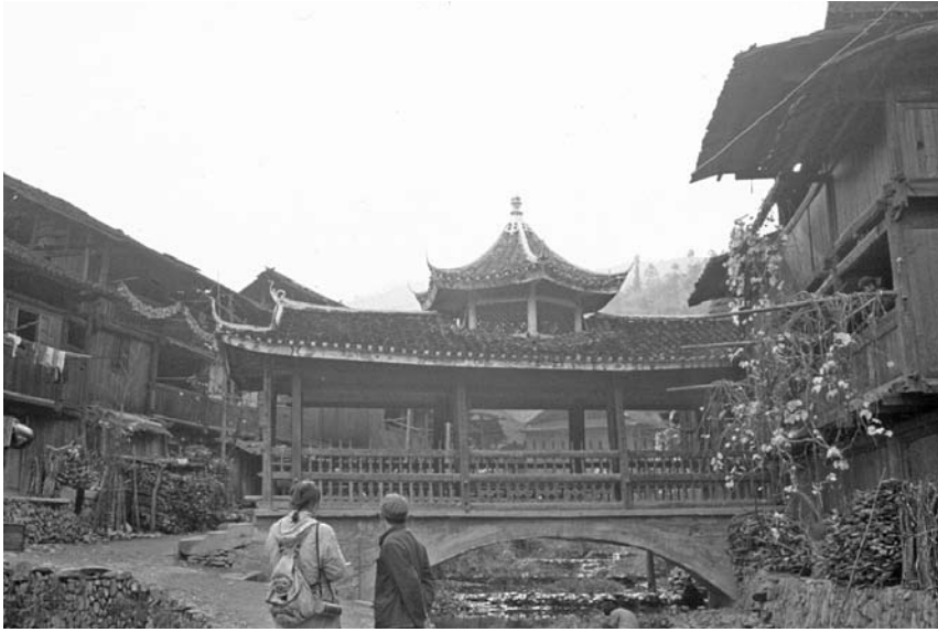
Figure 2.33 One of the wind-and-rain bridges in Zhaoxin village of the Liping region, Guizhou province, is in the center of the settlement, perhaps to bridge the “dragon’s veins.” Source: Photograph by Xing Ruan, 1993.
