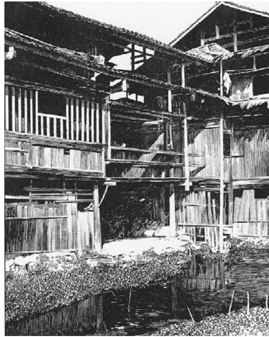
Figure 2.48 Dong houses are sometimes connected through overbridging. Mapang village of the Sanjiang region, Guangxi province. Source: Li Changjie et al. (1990, 385).
