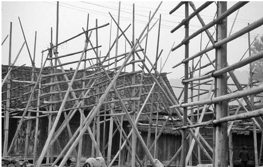
Figure 2.41 The heliang , the freestanding timber framework for drying rice paddies, in Binmei village of the Congjiang region, Guizhou province. Source: Photograph by Xing Ruan, 1993.
