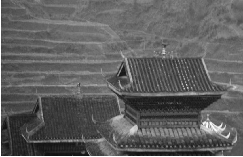
Figure 3.30 The top pavilion loft of the Baxie drum tower is a gable-and-hip roof. Baxie village, Sanjiang region, Guangxi province. Source: Photograph by Xing Ruan, 1989.
