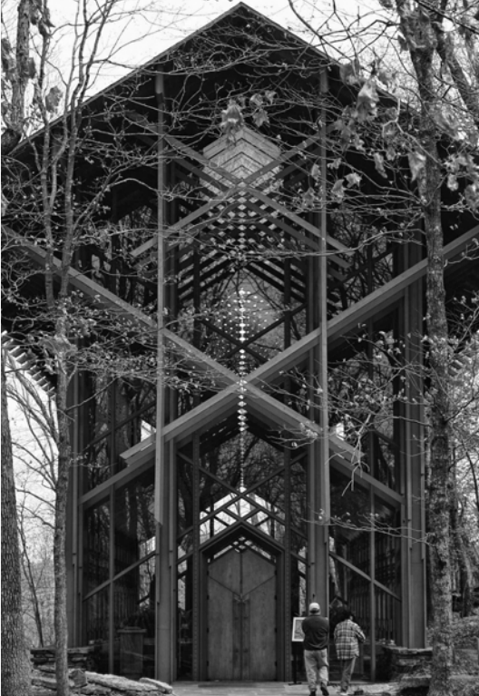
FIGURE 4.1 Photograph of the entry to Thornycrown Chapel, including interior cross bracing, Eureka Springs, Arkansas, United States (1979–1980). Architect: E. Fay Jones.
