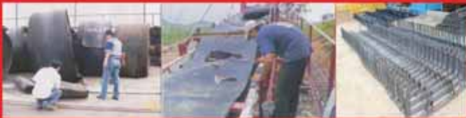
Conveyor Belt Joining
