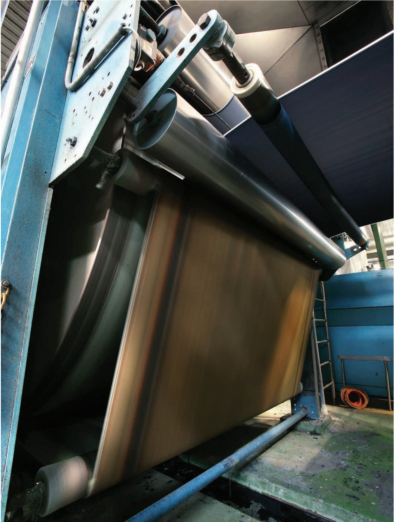
Sanforizing range. Exit Rubber belt section
