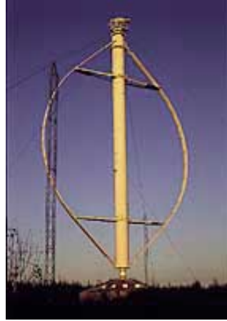
Fig.1.2 Vertical axis wind turbine
