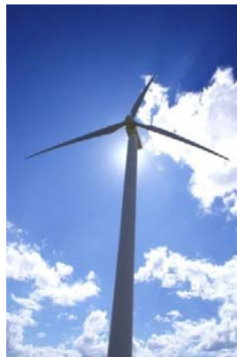
Fig.1.1 Horizontal axis wind turbine
