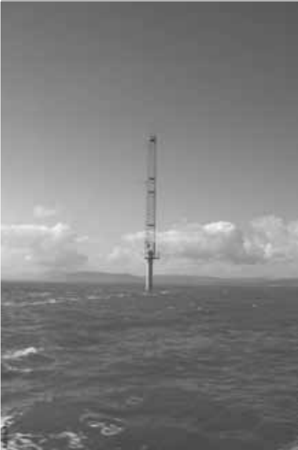
Figure I.5.1: An offshore meteorological mast
