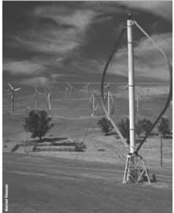
Figure I.3.3: Darrieus type vertical axis wind turbine
