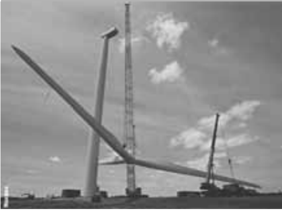
Figure I.3.27: Erection of Nordex wind turbines
