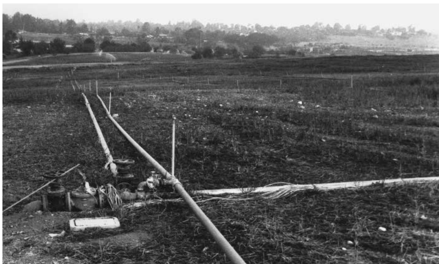
Figure 5-38 Completed landfill with irrigation system.
