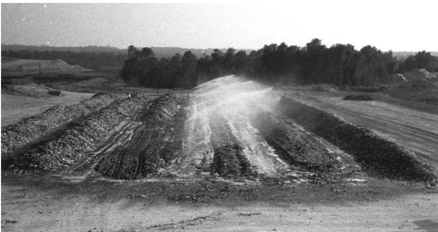
Figure 5-20 Overview of windrow composting operation.
