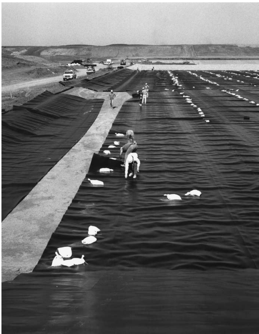
Figure 5-28 Placement of geomembrane liner in area-type landfill.
