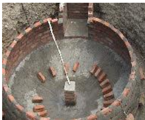
Fig.-3: Deenbandhu in-situ model under construction
