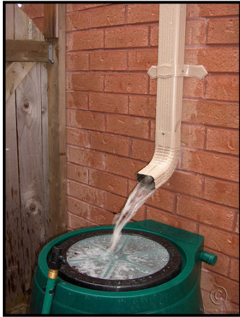
Figure. 4 Rainwater collection (through downpipes and sieves)
