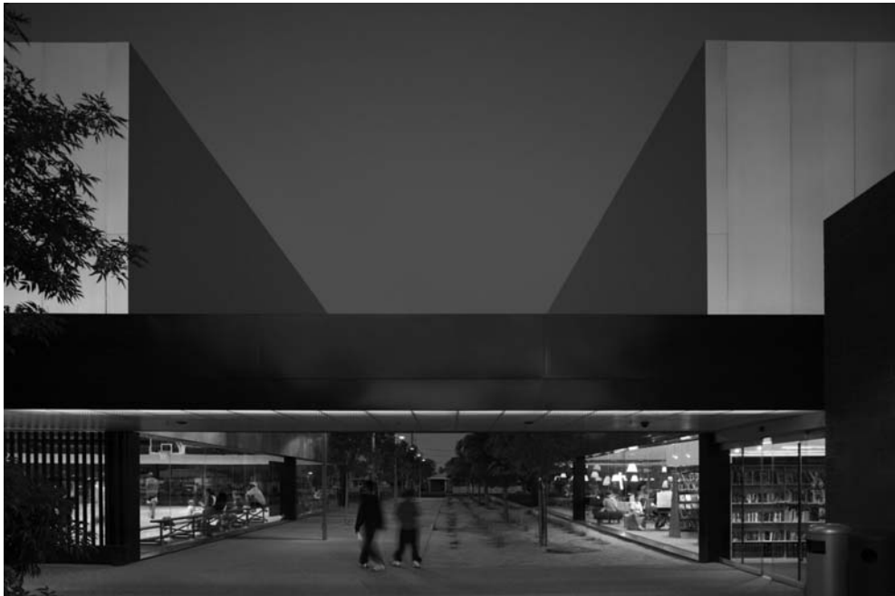
Figure 44.1 Palo Verde Library and Maryvale Community Center in Phoenix, AZ, 2006, designed by Gould Evans & Wendell Burnette Architects. Source: Bill Timmerman – used by permission.
