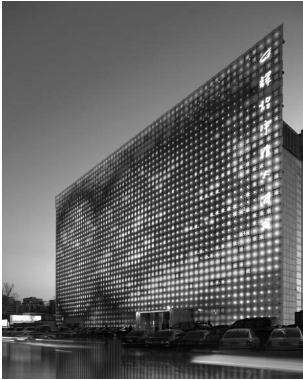
Figure 34.8 The GreenPix Zero Energy Wall in Beijing. Source: ©Simone Giostra & Partners/Arup/Ruogu – used by permission.
