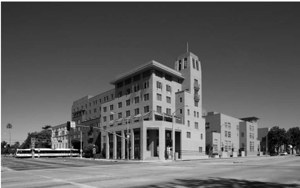
Figure 49.3 Del Mar Station, Pasadena, CA. Source: Moule & Polyzoides, 2006 – used by permission. Note: The fabric of buildings surrounding a transit station should be configured in block-appropriate massing that supports a pedestrian-friendly public realm.
