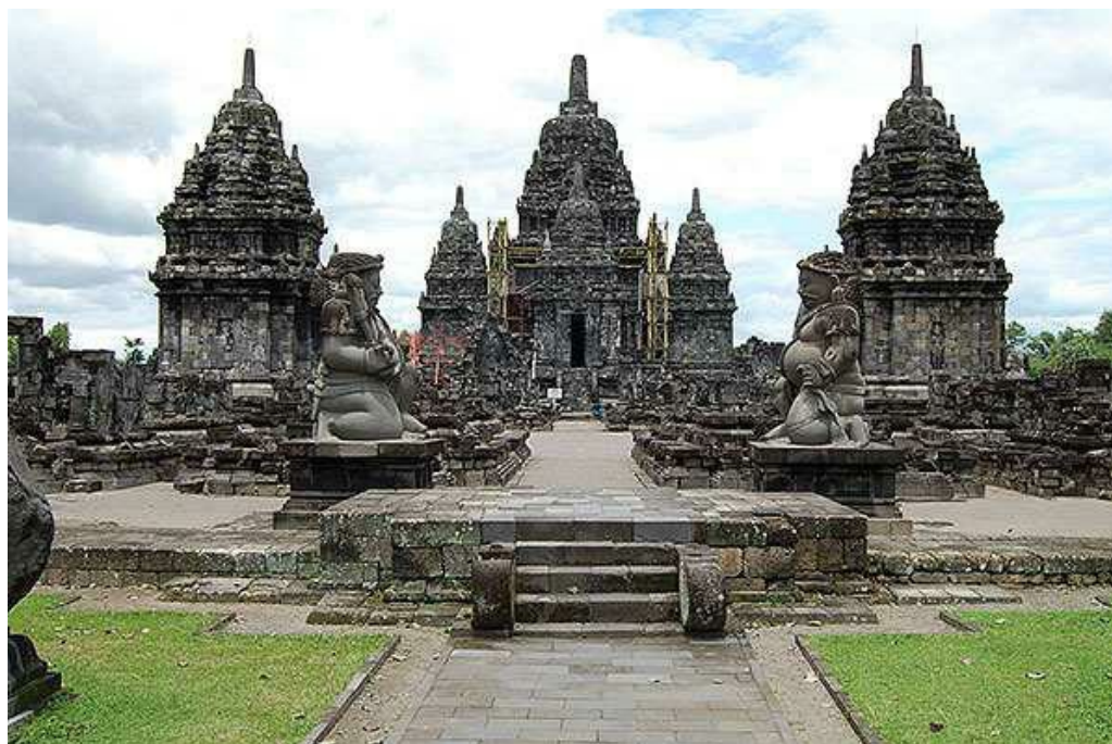
7.13 View of remaining temples c. 792-817 CE Yogyakarta- Indonesia
