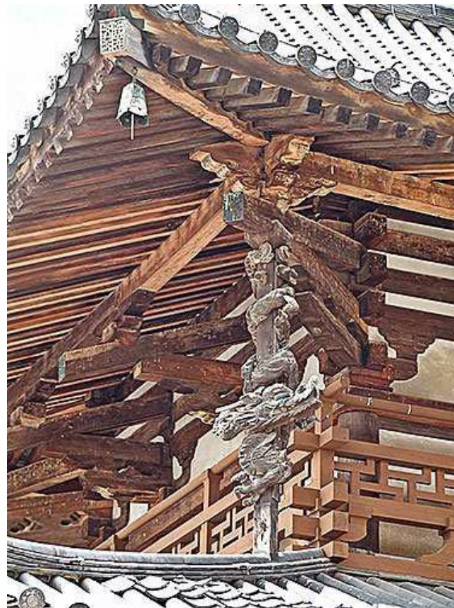
4.7 Eave brackets of Golden Hall 623 CE Nara- Japan
