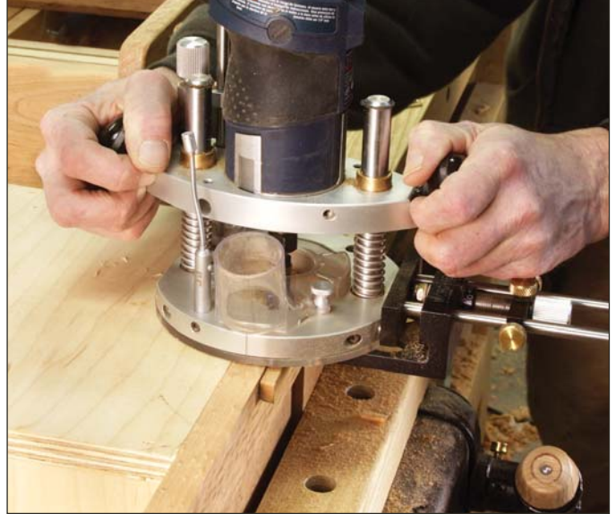
Support group. I clamp the door in my vise with the top edge of the door even with the top of a wood block. The fence on the router sets the distance for the hinge mortise, and the base of the router can't tip.
