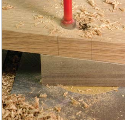
On the up and up. A wedge below the arm provides the proper tilt to keep the holes vertical.
