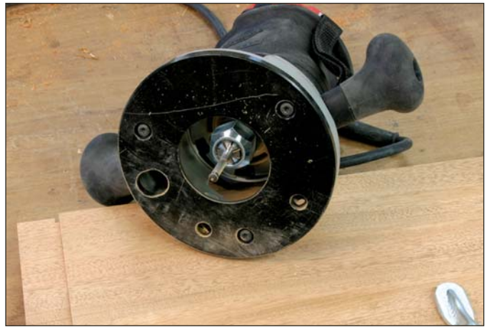
A small-diameter flush-cutting bit follows the template and shapes all of the cloud lifts accurately and identically leaving only minimal sanding to be done.
