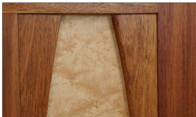
The difference in thickness between the corbel and the adjacent stile and rail adds visual interest.
