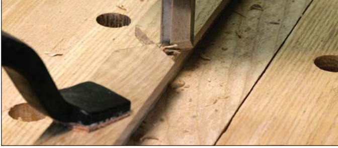
Cutting corners. The router will leave material in the corner, which can be removed with a chisel. The finished edges of the joint have been established with the knife and saw.
