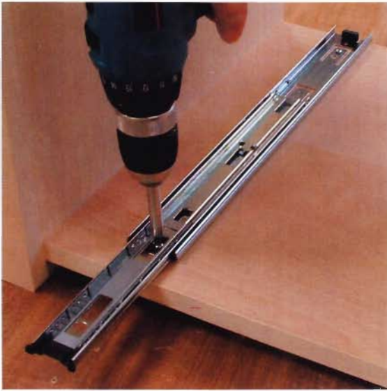
9 Install the drawer glide hardware in the center of the drawer side and locate the cabinet part of the glide on the cabinet side, accordingly.
