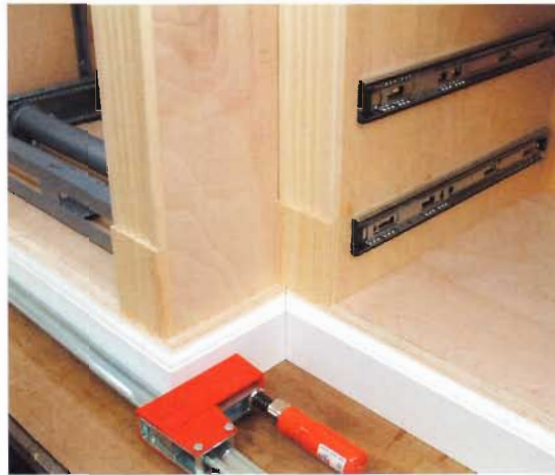
22 Assemble the bookcases. Install the lift in the center cabinet. Attach the side base cabinets to the center cabinet with screws. Screw the tops and the bookcases to each of the side cabinets. Then, cut and glue the two base trim returns to the center cabinet.
