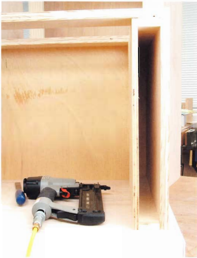
13 Glue the base trim on the front and side of the two small base cabinets. Be sure to make left and right cabinets. Glue the side spacers at the top and bottom of these base cabinets. Then nail the inner sides to the spacers.
