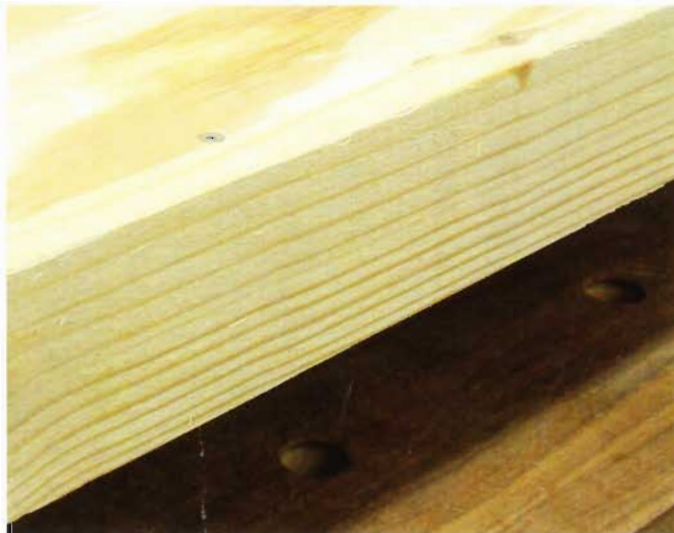
11 Cut the plywood bottom to size and install it so it rests on the cleats inside the cabinet. Attach it with screws inserted into the cleats.
