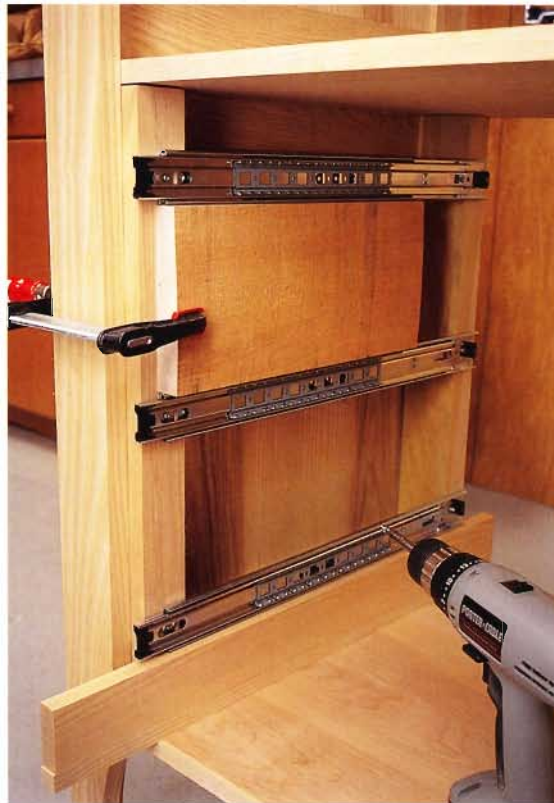
18 Lay out where the hardware will be mounted on the drawers and transfer this to the cabinet sides. Use temporary spacers to hold the hardware parallel to the cabinet bottom. The spacers also ensure the hardware will be located at the same height on both sides of the cabinet.
