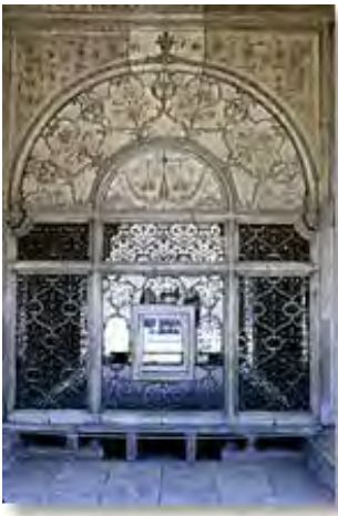
Jali work, Khas Mahal, Red Fort, Delhi
