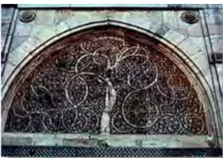
Jali Work, Sidi Sayyid Mosque,
