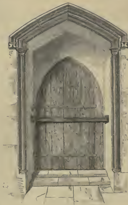
FELMARSHAM CHURCH, BEDFORDSHIRE.
