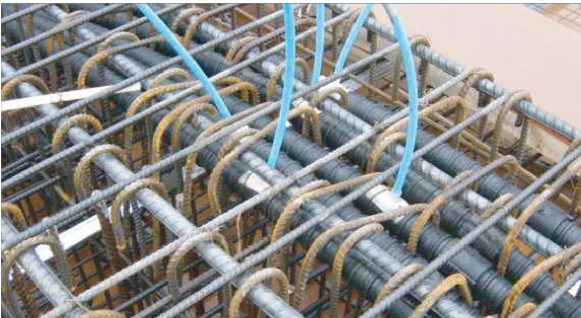
Figure 7.40 Typical ducts in transfer beams (courtesy of Sir Robert McAlpine Ltd)
