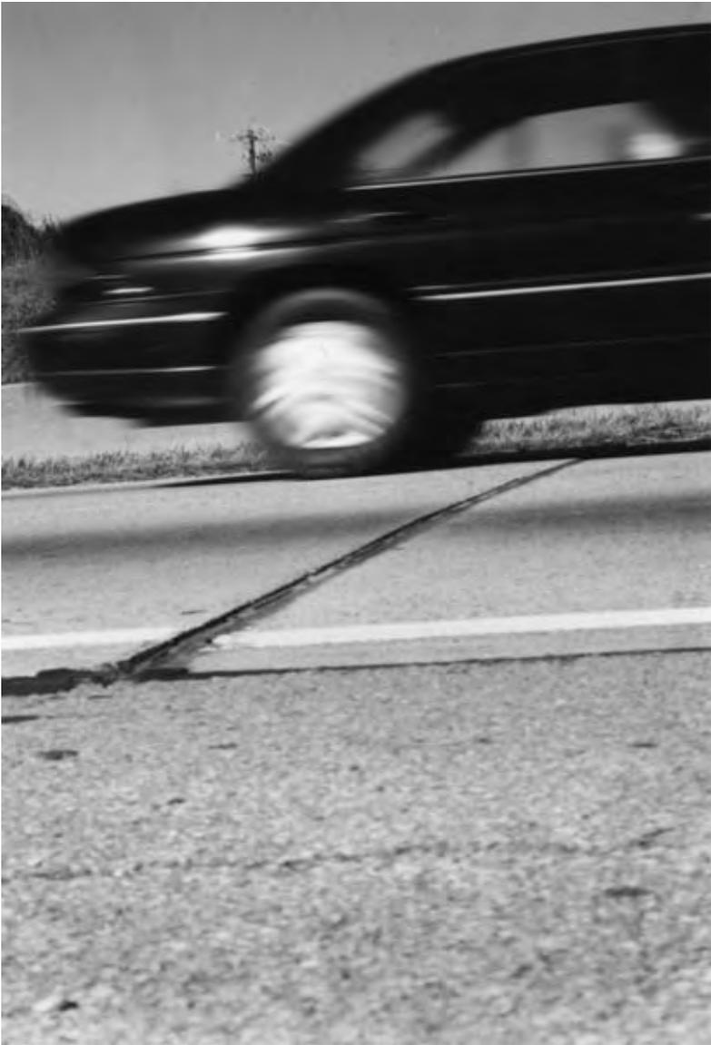
*Figure 3.10* Faulted transverse joint (photo by author).
