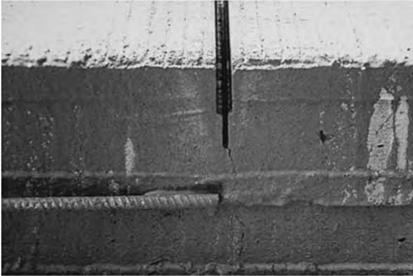
Figure 15.3 Transverse joint initial and widening cut (ACPA 1996a: VII-11).
