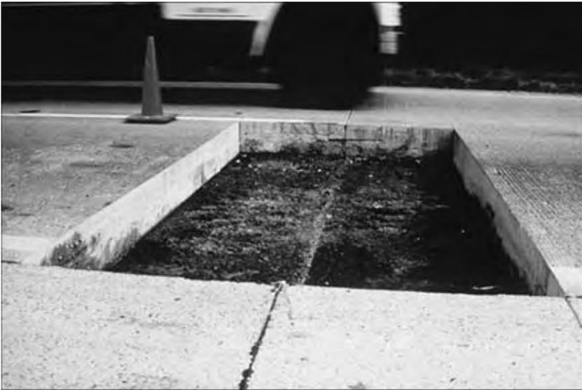
Figure 17.1 Hole prepared for a full depth repair at a joint (ACPA 1996a: VIII-28).
