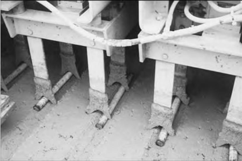
Figure 14.7 Dowel bar inserters (ACPA 1996a: VI-32).
