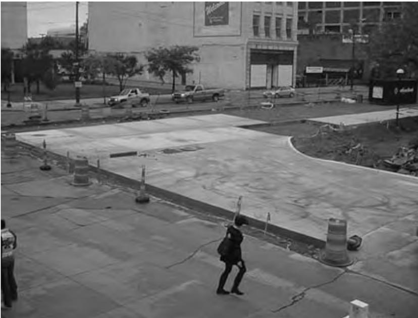
Figure 9.9 Quadrant construction at an urban intersection in Cleveland, Ohio (photo by the author).
