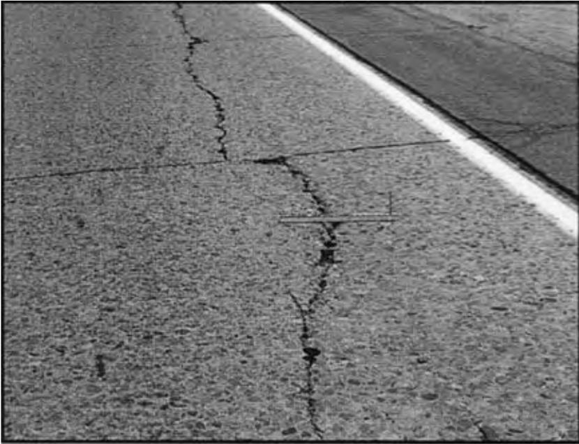
Figure 3.3 High severity longitudinal crack (Miller and Bellinger 2003: 39).
