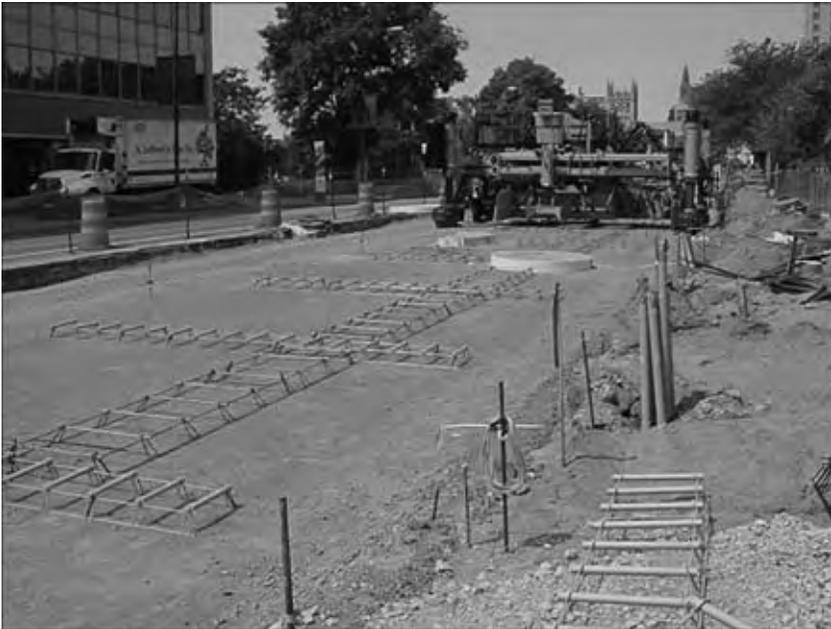
*Figure 2.6* Tie bar basket assemblies with corrosion resistant epoxy-coated tie bars – dowel baskets are also shown (photo by author).
