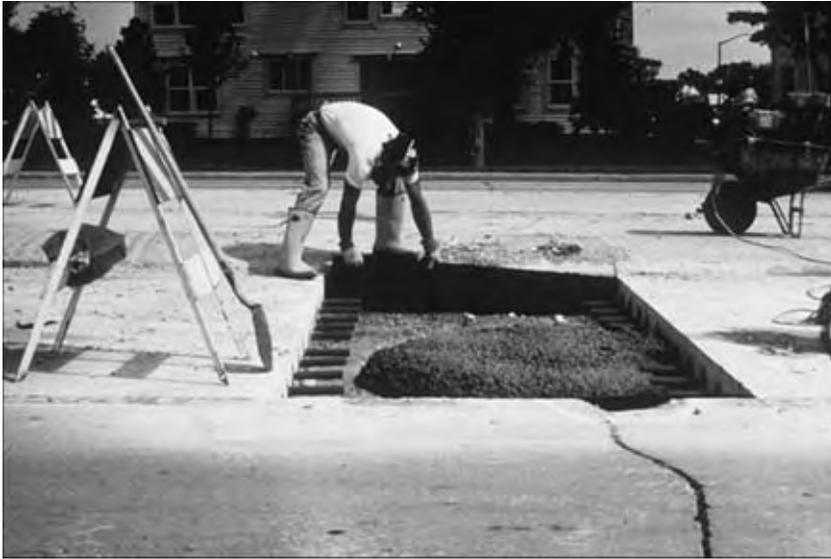
Figure 17.3 Full depth repair with dowels and fiberboard for isolation (ACPA 1996a: VIII-41).
