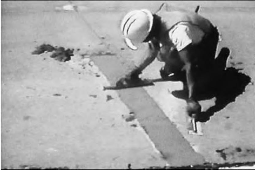
Figure 17.2 Partial depth repair (ACPA 1996a: VIII-57).
