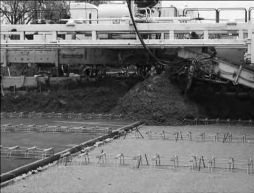
Figure 18.3 Unbonded overlay on two lanes with a third lane paved at the same time (photo courtesy: Dale Crowl).
