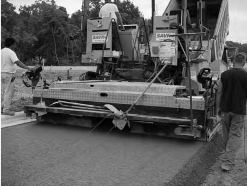
Figure 2.10 RCC pavement construction – Columbus, Ohio (photo by author).
