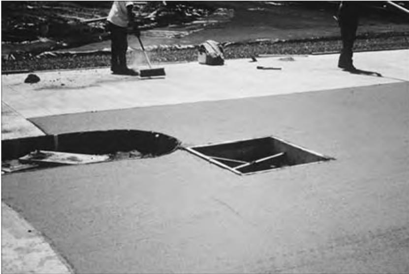
Figure 14.11 Blockouts for utility, drainage, and similar structures (ACPA 1996a: VI-91).
