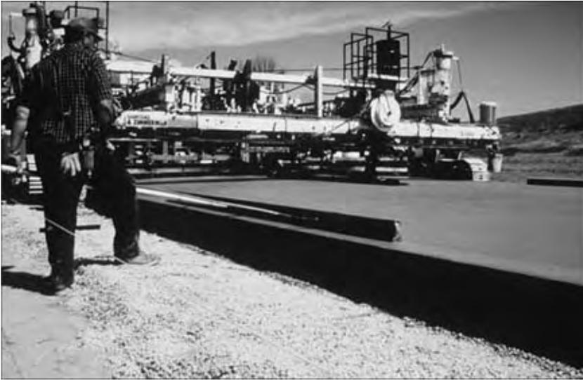
Figure 14.2 Concrete pavement produced by slipforming (ACPA 1996a: VI-6).
