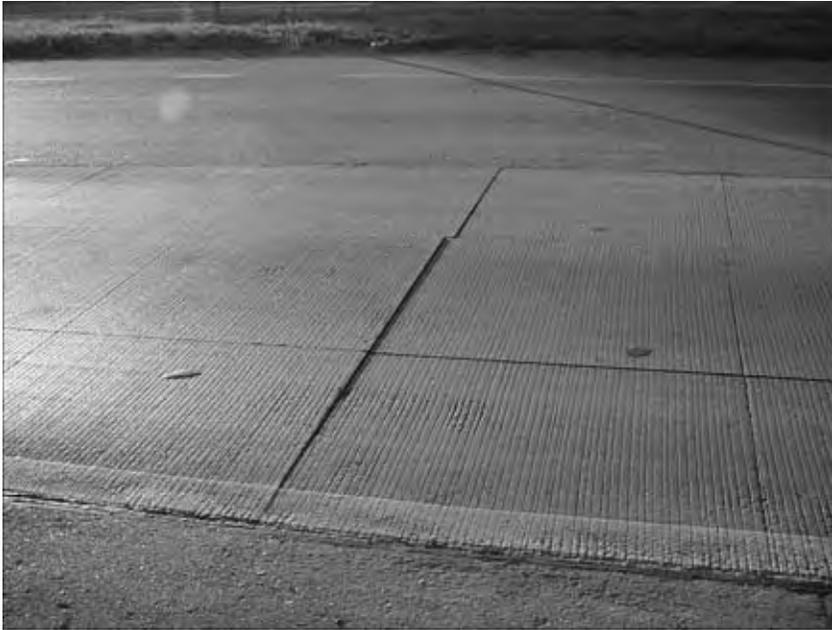
Figure 18.9 Failure of UTW by panel sliding (photo by the author).
