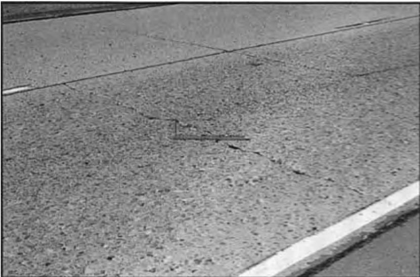
Figure 3.4 High severity transverse crack in JRCP (Miller and Bellinger 2003: 41).
