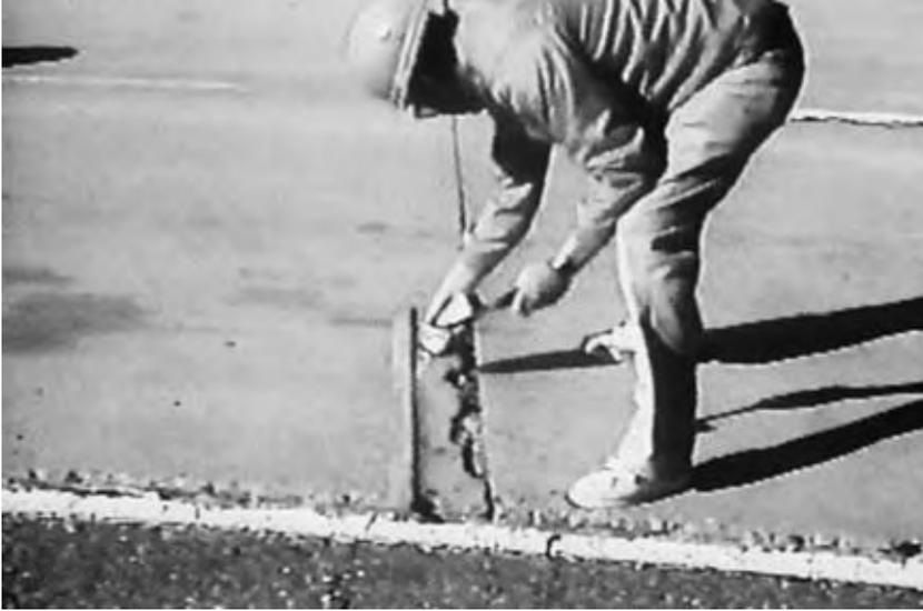
Figure 3.5 High severity transverse joint spalling (ACPA 1996a: VIII-47).
