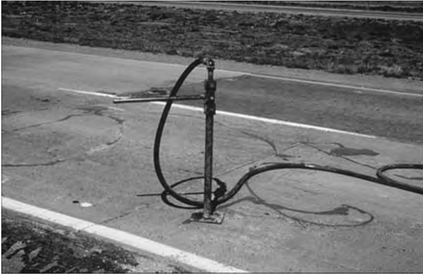
Figure 17.6 Grout injection for slab stabilization (ACPA 1996a: VIII-23).
