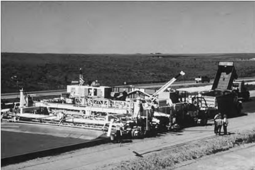
Figure 14.1 Slipform paving train (ACPA 1996a: VI-6).
