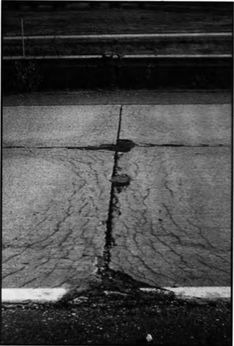
*Figure 3.2 High severity D-cracking (Miller and Bellinger 2003: 37).*
