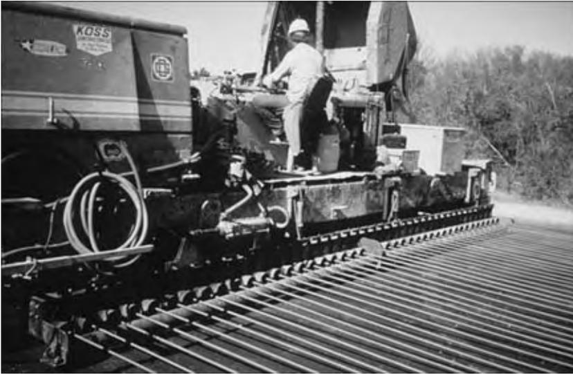
Figure 14.8 CRCP steel installation with tube feeders (ACPA 1996a: VI-37).
