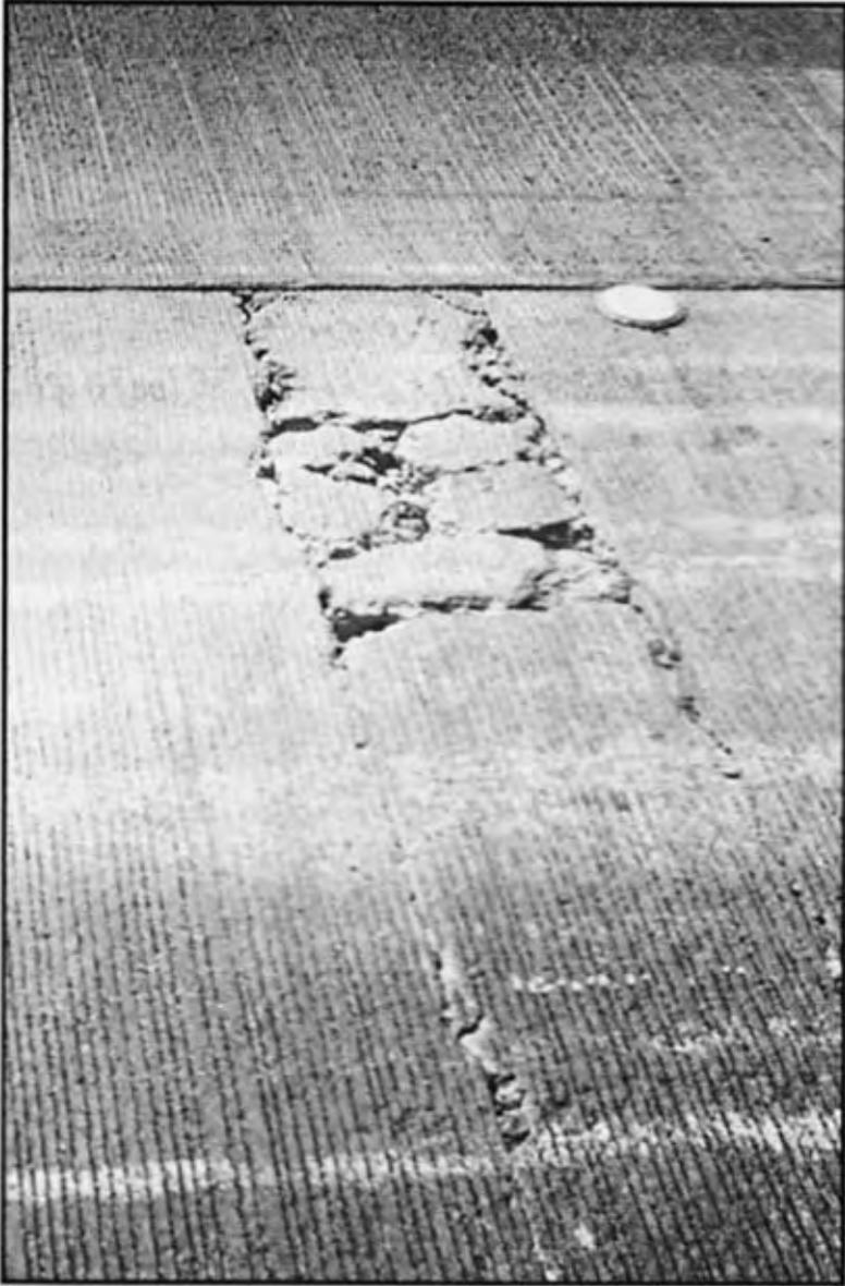
*Figure 3.12* High severity punchout (Miller and Bellinger 2003: 79).
