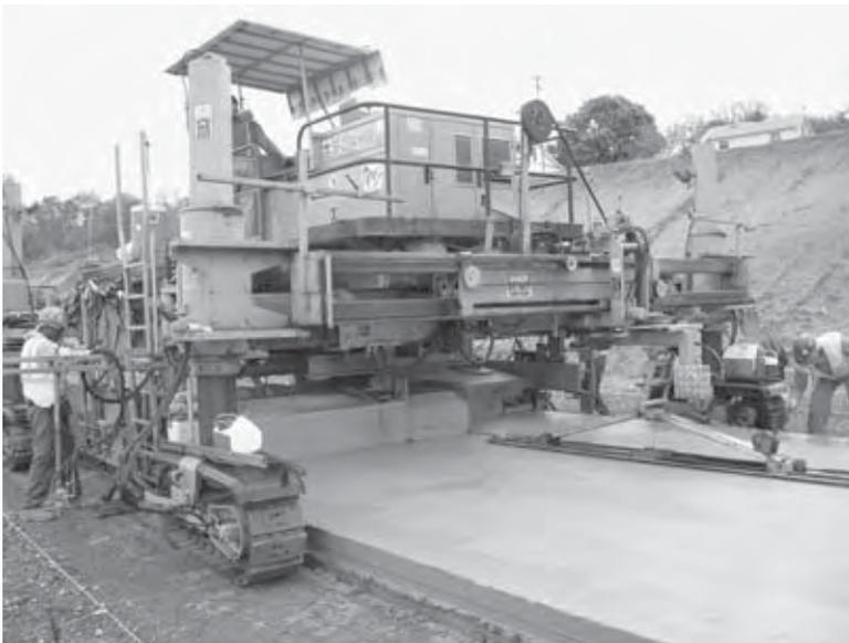
Figure 1.2 (a) and (b) Slipform pavers (photo courtesy of The Great Lakes Construction Company, Hinckley, Ohio).
