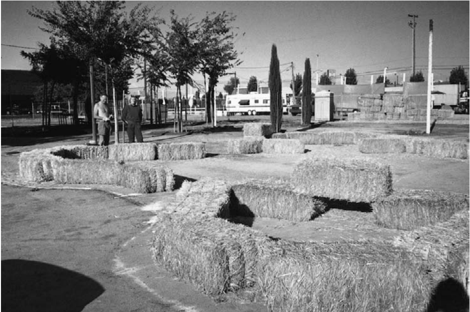
Marking out a (straw-bale) building with straw bales. Such full-size modelling enables better space fine-tuning than does any drawing. It's also easier for non-professionals to understand and simulate using. And lots of hands can build – and adjust – it!
