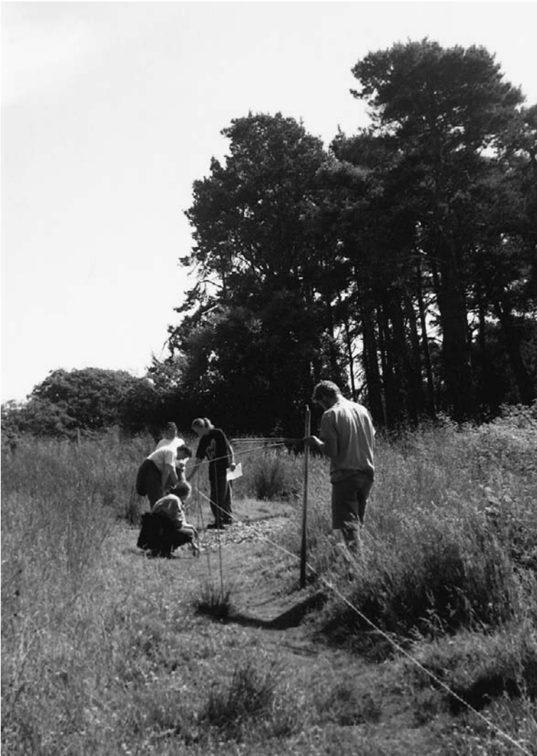
Marking-out a building on site. Is it right here? Or should the plans be adjusted?
