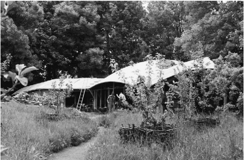
The first building takes shape.
