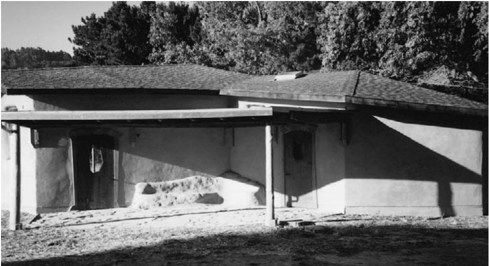
The first of the new (straw-bale) buildings. Design: East Bay Waldorf School, Greg van Mechleren, Bob Davidson, Christopher Day and Vital Systems (the part professional, part volunteer, building group).
