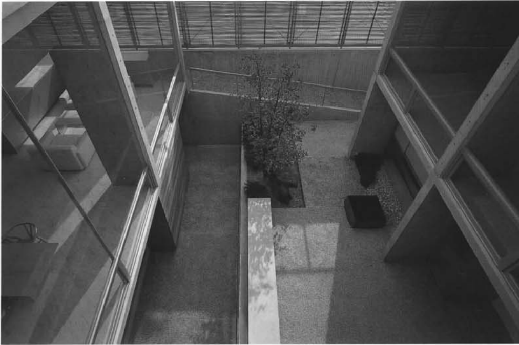
(above) Downward view of the courtyard. (below) The living-dining room opens up to the town through the louvers. (p.119) View of the courtyard.
