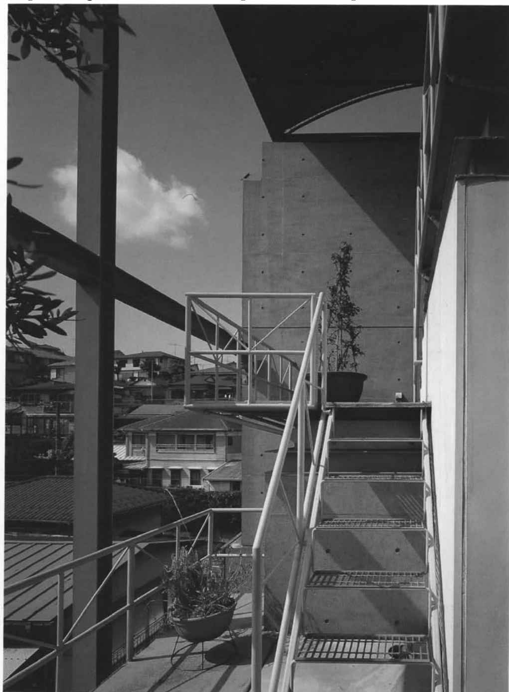
right) View of the exterior stairs, on the southwest corner.
