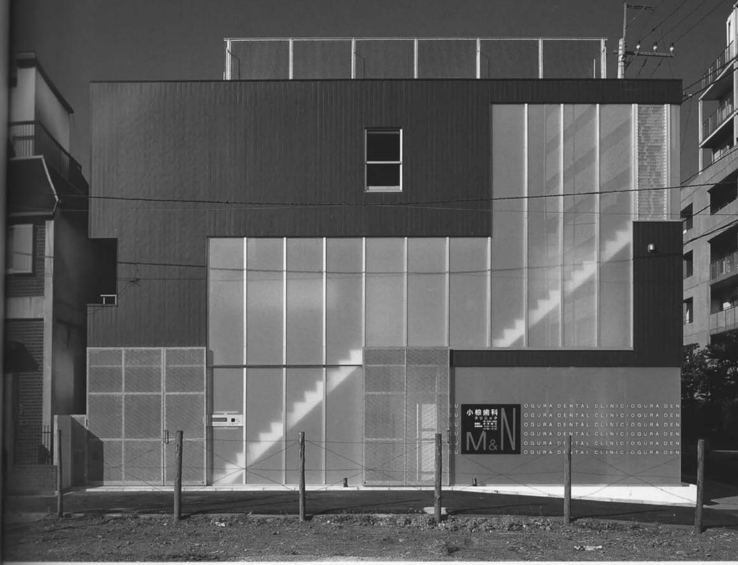
(above) Exterior view from the east. The expanded-metal sliding door on the left is the entrance to the residence and parking area. The sliding door on the right is the entrance to the dental clinic.
