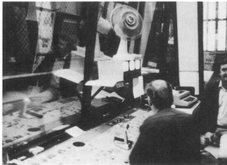
Reflective glass in the control center can inhibit officer view when light levels are too high in the control space.
