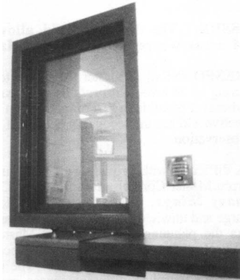
View from lobby of Master Control CCTV monitor and into the jail.
