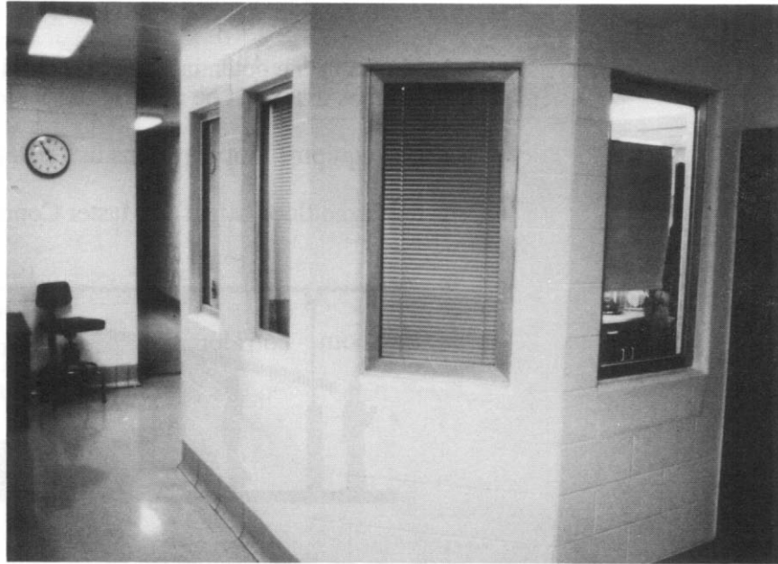
Blinds used by Master Control staff block view of staff by inmates, but defeat location and design of the space.
