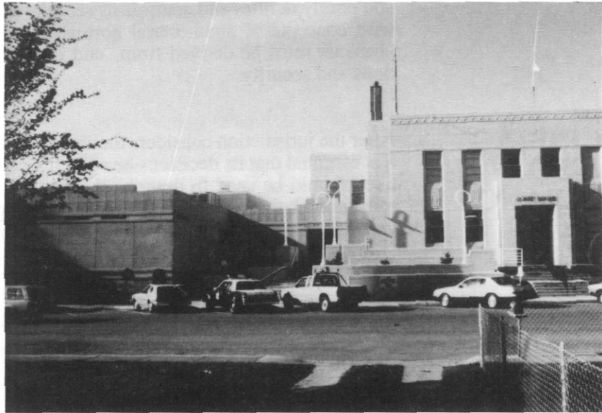
Jail (on the left) using materials, detailing, and scale to complement the appearance of an existing courthouse.
