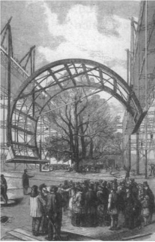
The Crystal Palace, designed by the botanist Joseph Paxton, was constructed in six months from modular cast- and wrought-iron structural elements bolted together to receive thousands of pieces of glass. Etching courtesy of Phaidon Press.
