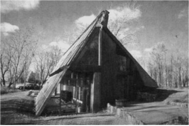
Orobolous, a research project of the University of Minnesota, was designed to be heated with solar energy and electrified by a windmill. A clivus multrum processed human waste into the soil.
