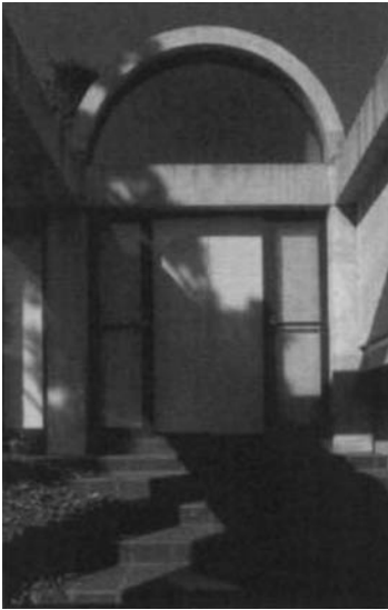
Wall House courtyard. Photograph courtesy of Tadao Ando.
