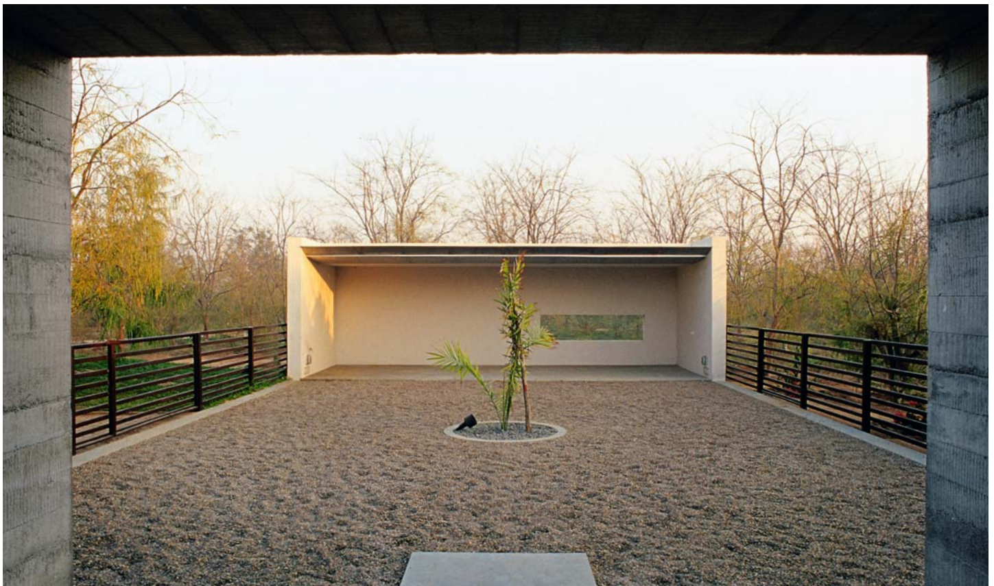
Roof terrace and pavilion — Roof terrace
