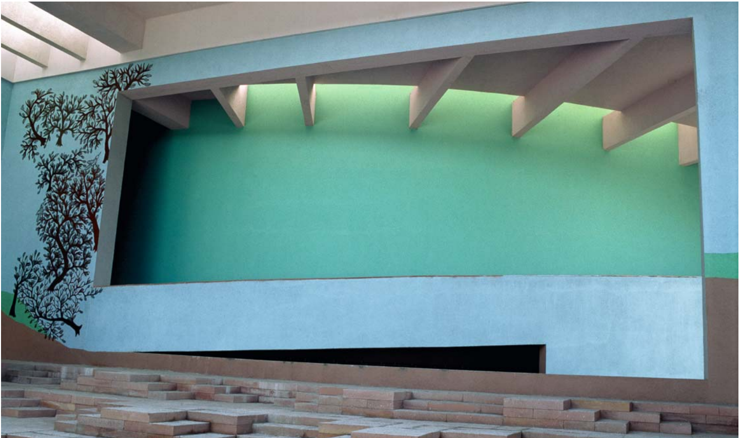
Main entrance for the public and wall of the multi-purpose room — In the public waiting area
