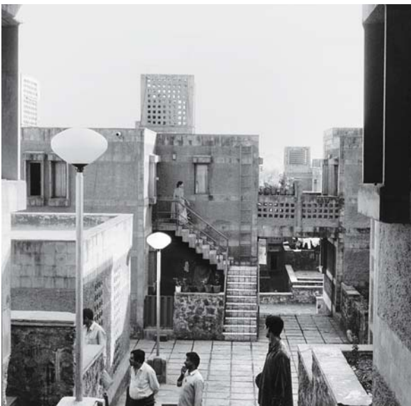
Courtyards and terraces
