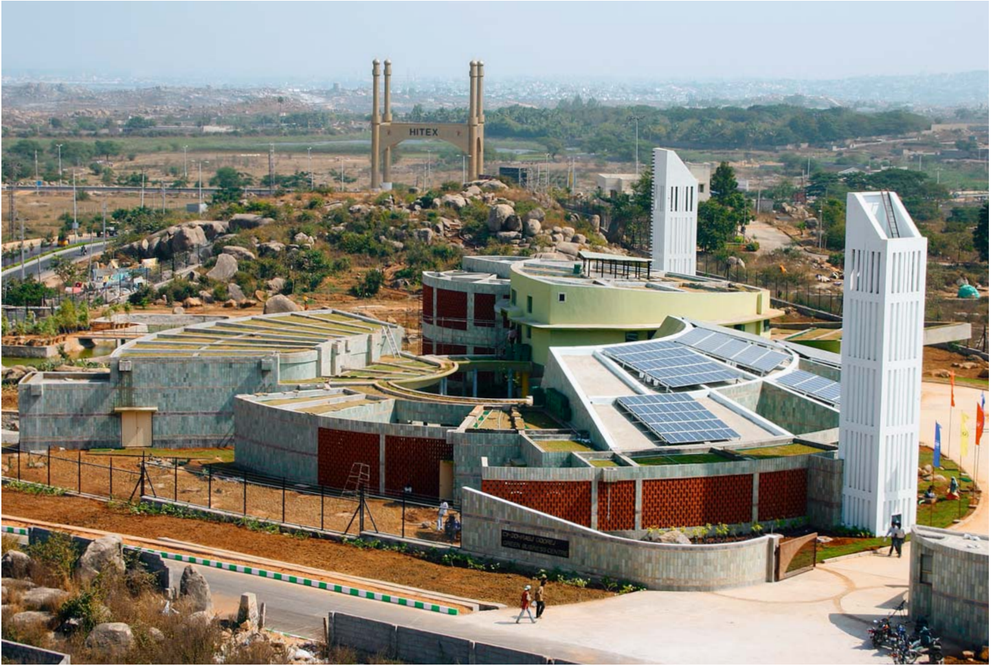
Full view of the complex
