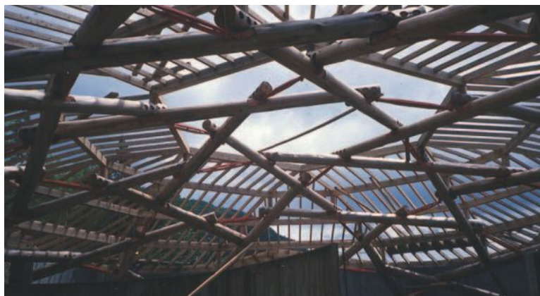
▲ 9.12 The roof under construction – internal view. (Photo: Keikaku-Inc.)
