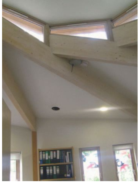
▲ 10.30 Office building – internal view.
