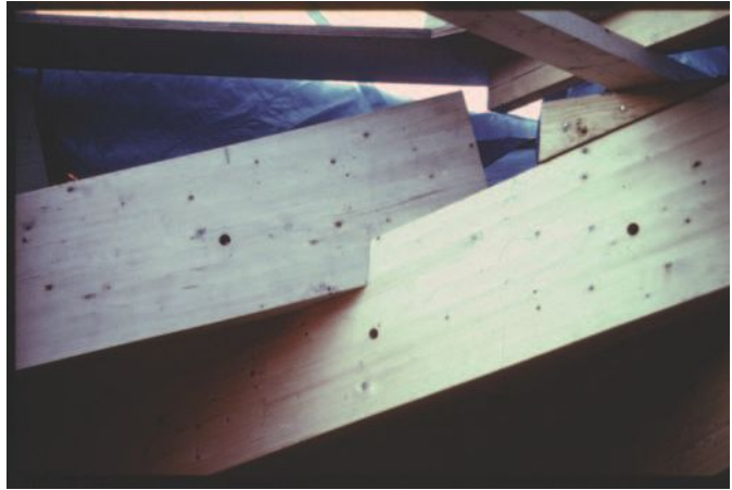
▲ 5.4 Notched connection – Graham Brown’s RF building under construction.
