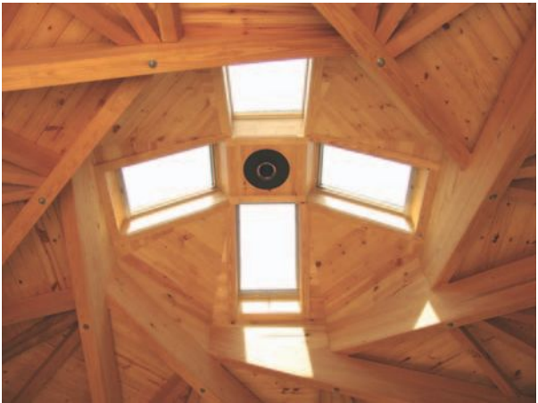
▲ 11.11 The roof light – internal view. (Photo: Fred Oesch.)
