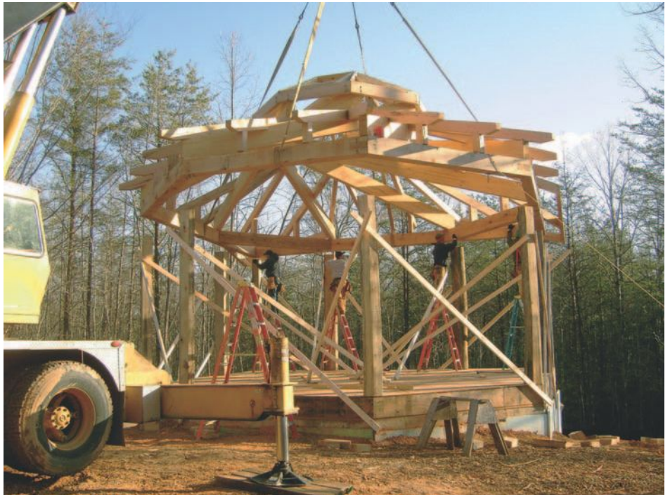
▲ 11.9 The finished skeleton. (Photo: Fred Oesch.)
