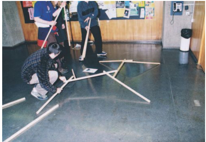
▲ 3.10 Sheffield architecture students constructing a multiple RF grid dome – 1.
