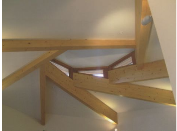
▲ 10.25 Internal view towards the roof light.
