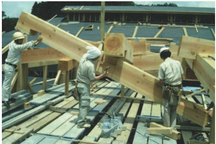
▲ 7.52 Assembling the timber beams' pre-cut beams. (Photo: Kazuhiro Ishii.)
