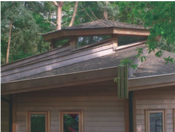
▲ 10.31 Office building – roof close-up.
