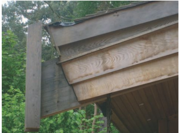
▲ 10.18 Eaves detail – side view.
