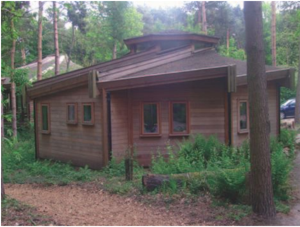
▲ 10.29 Office building – close-up.
