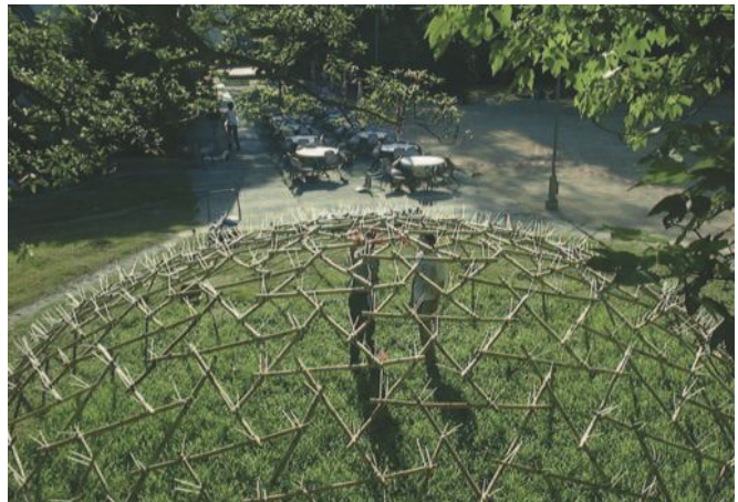
▲ 3.32 Bertin’s 10-metre bamboo multiple RF grid dome. (Photo: Vito Bertin.)
