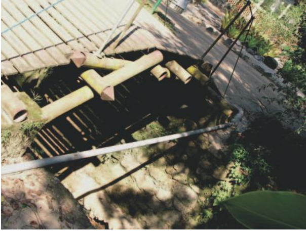
▲ 2.12 Pedestrian RF bridge. (Photo: Andy Tyas.)
