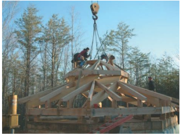
▲ 11.8 Fitting the roof light. (Photo: Fred Oesch.)
