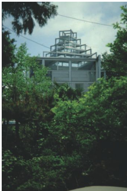
▲ 7.10 Spinning house – external view. (Photo: Kazuhiro Ishii.)
