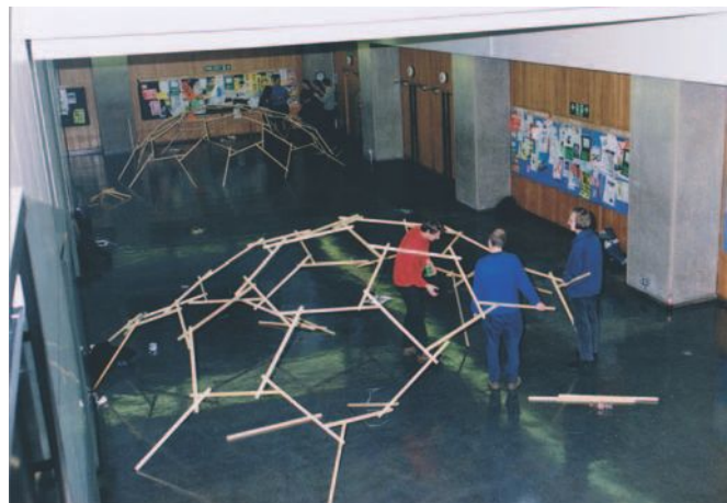
▲ 3.13 Constructing a multiple RF grid dome - 4.
