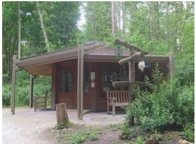
▲ 10.34 A small shelter RF building.
