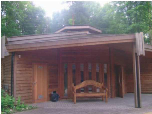
▲ 10.23 Gathering building – elevation facing the internal courtyard.
