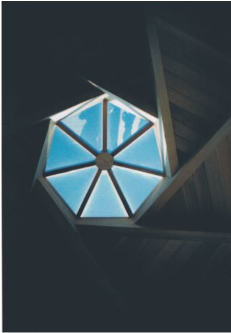
▲ 10.3 Gazebo – internal view.
