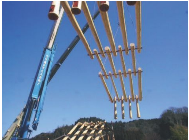
▲ 7.59 The pinned timber structure folds and is locked into its final position. (Photo: Kazuhiro Ishii.)
