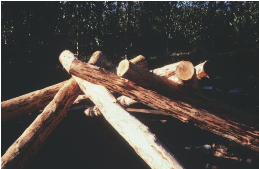
▲ 10.12 Findhorn Earth sanctuary. Wooden poles were used for the RF roof.
