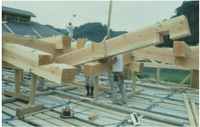
▲ 7.51 Construction of the auditorium roof chopstick structure. (Photo: Kazuhiro Ishii.)
