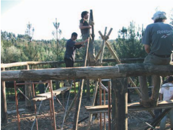
▲ 11.3 Constructing the house – view showing the temporary support. (Photo: Tony Wrench.)
