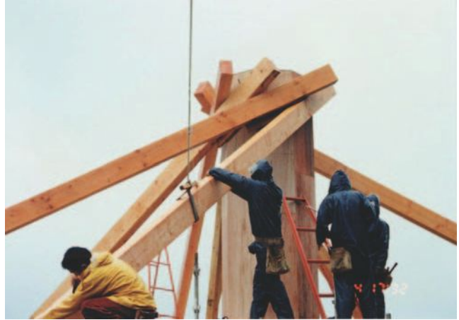
▲ 5.6 Friction connection – the New Farmhouse RF building by Yoichi Kan under construction. (Photo: Yoichi Kan.)
