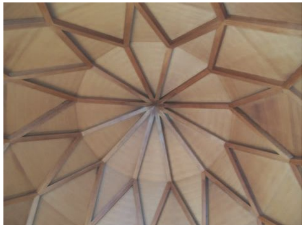
▲ 7.29 The geodesic dome forms the roof enclosure - internal view.
