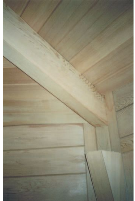
▲ 10.4 Gazebo – internal finishes.
