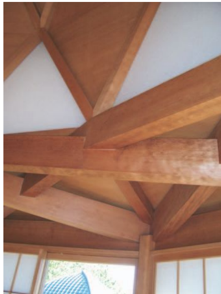
▲ 7.30 Complex notched timber connections.
