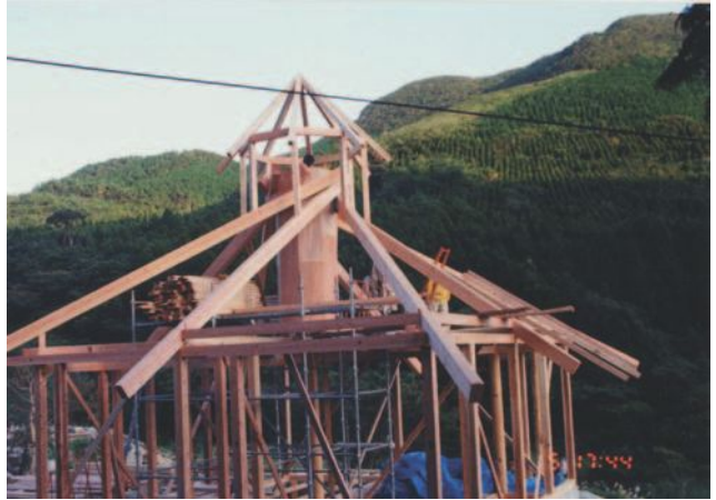
▲ 8.20 The RF structure becomes stable when all the beams are installed. (Photo: Yoichi Kan.)
