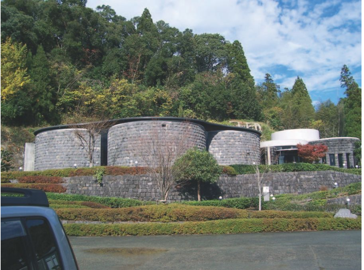
▲ 9.6 The Stonemason Museum in context. The full height narrow windows bring in a slit of light.
