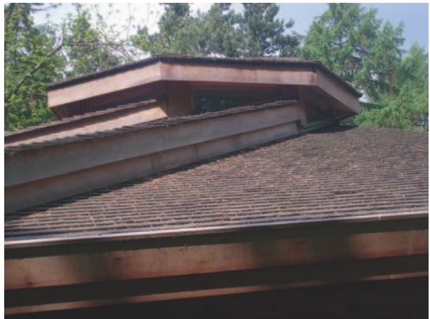
▲ 10.26 RF roof – close-up.
