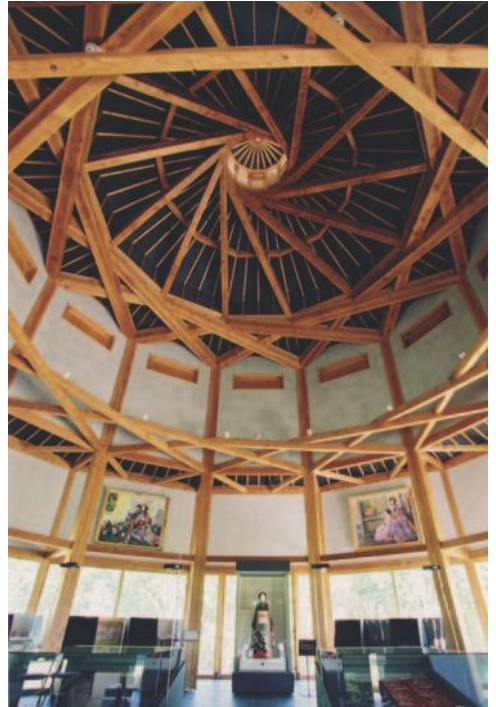
▲ 7.34 The double height space of the exhibition hall makes the space feel bigger than it really is. (Photo: Kazuhiro Ishii.)
