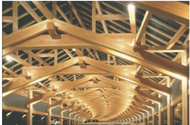
▲ 7.54 The roof structure of the shop and café building is a type of RF structure – internal view. (Photo: Kazuhiro Ishii.)
