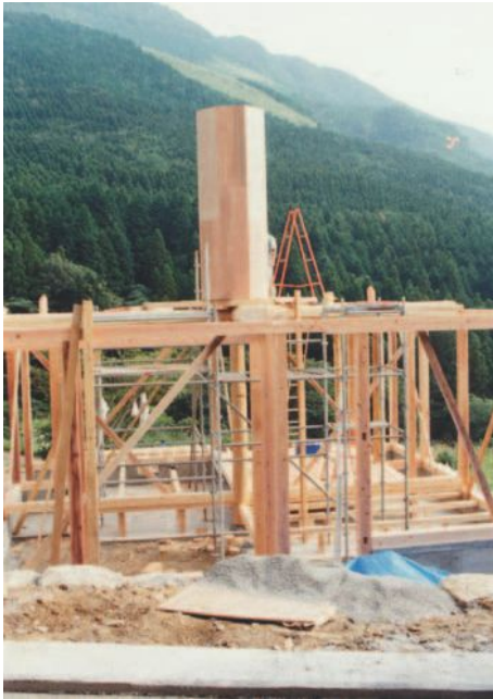
▲ 8.17 Construction of the RF is done using a temporary prop.
