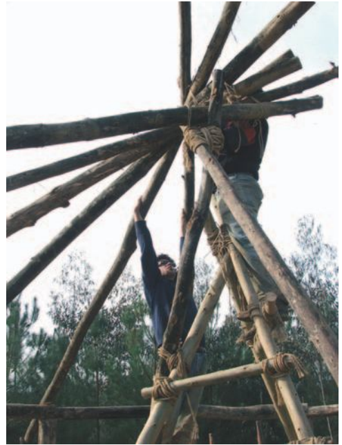
▲ 11.4 Constructing the roof. (Photo: Tony Wrench.)
