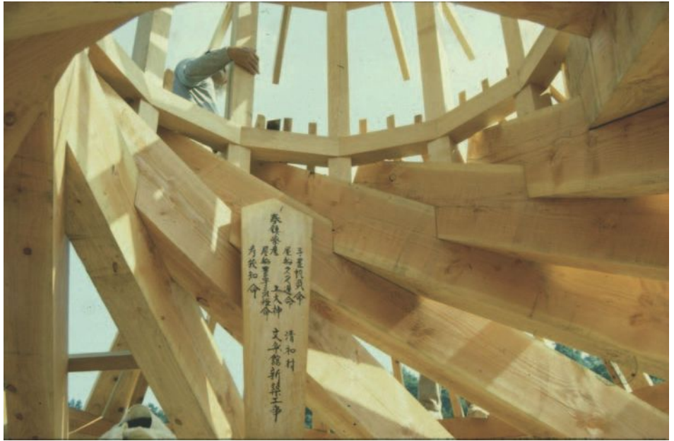
▲ 7.43 Internal view of the RF roof structure. (Photo: Kazuhiro Ishii.)
