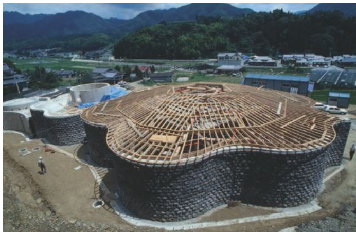
▲ 9.11 The roof under construction – external view. (Photo: Keikaku-Inc.)
