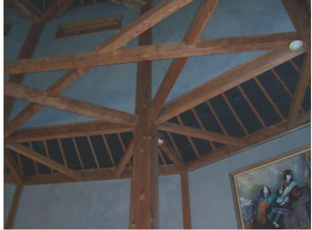
▲ 7.37 The RF-like ring beam reduces buckling.
