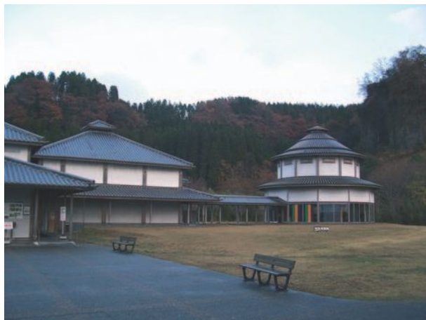
▲ 7.47 The auditorium building is connected to the exhibition hall via a covered walkway.
