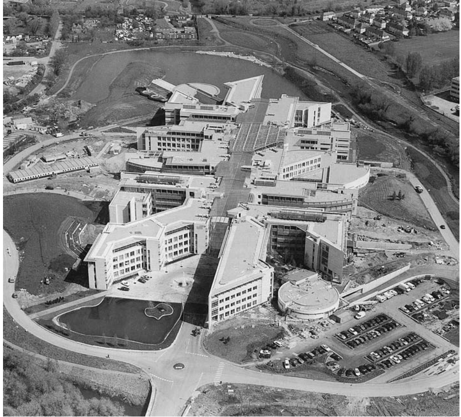
▲ 13.3 British Airways headquarters – Waterside, Heathrow
