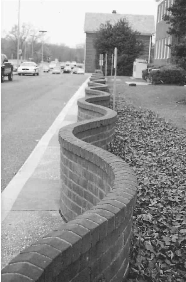
Figure 4.65 Photograph of serpentine brick wall.
