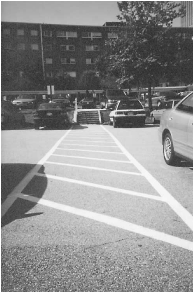
Figure 5.41 Photograph of markings in parking lots.
