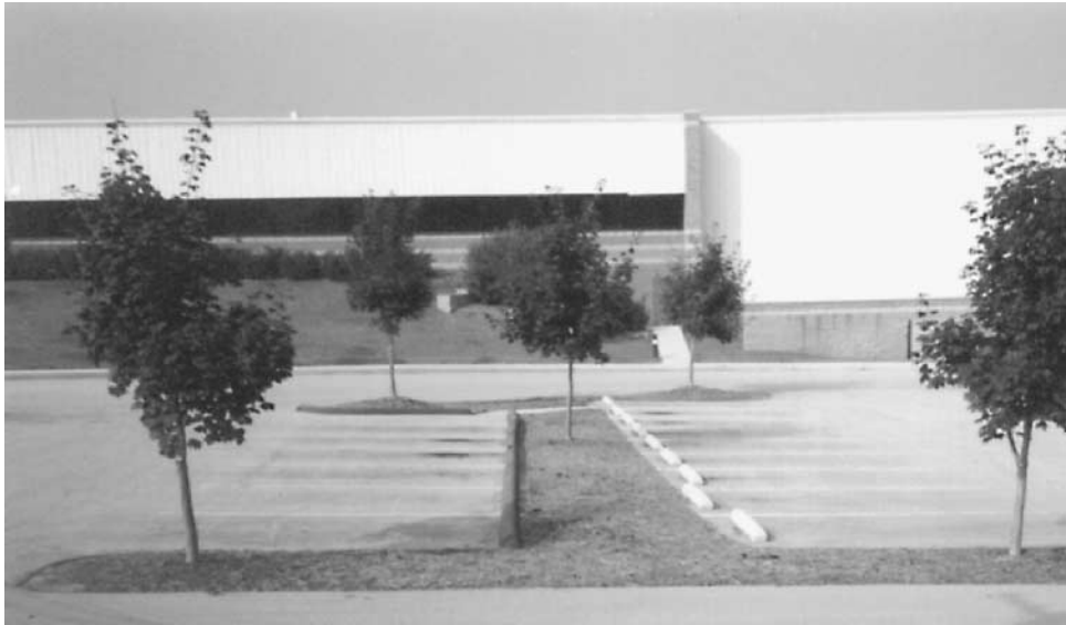
Figure 6.7 Photograph of parking lot island infiltrator.
