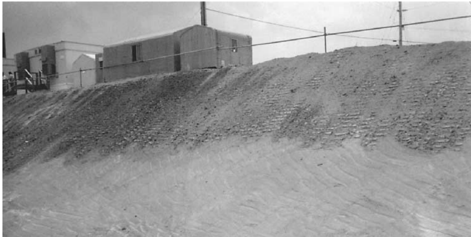
Figure 3.4 Photograph of roughened surface.
