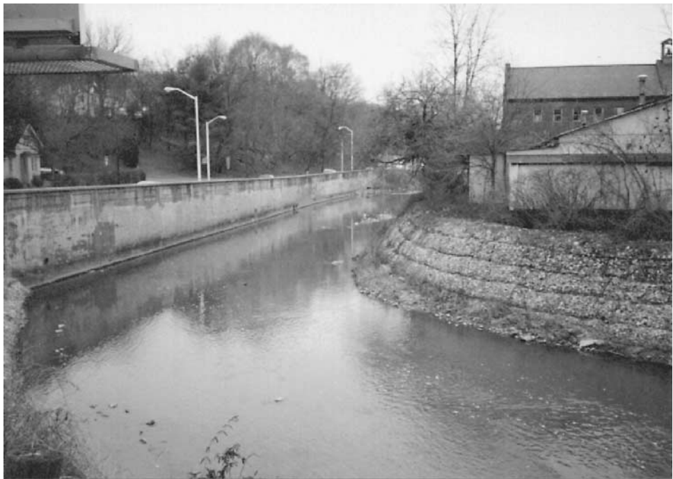
Figure 3.22 Photograph of gabion wall.
