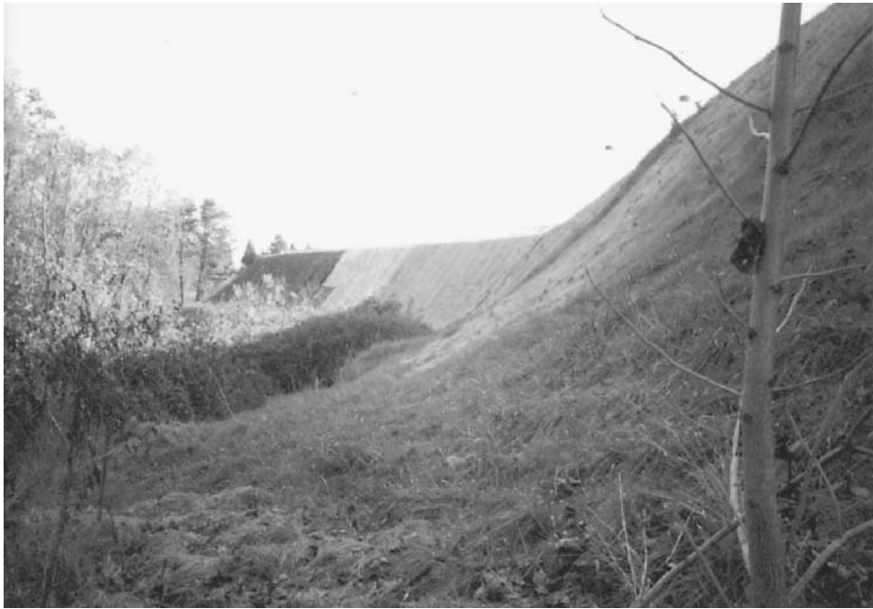
Figure 3.24 Photograph of stabilized slope.
