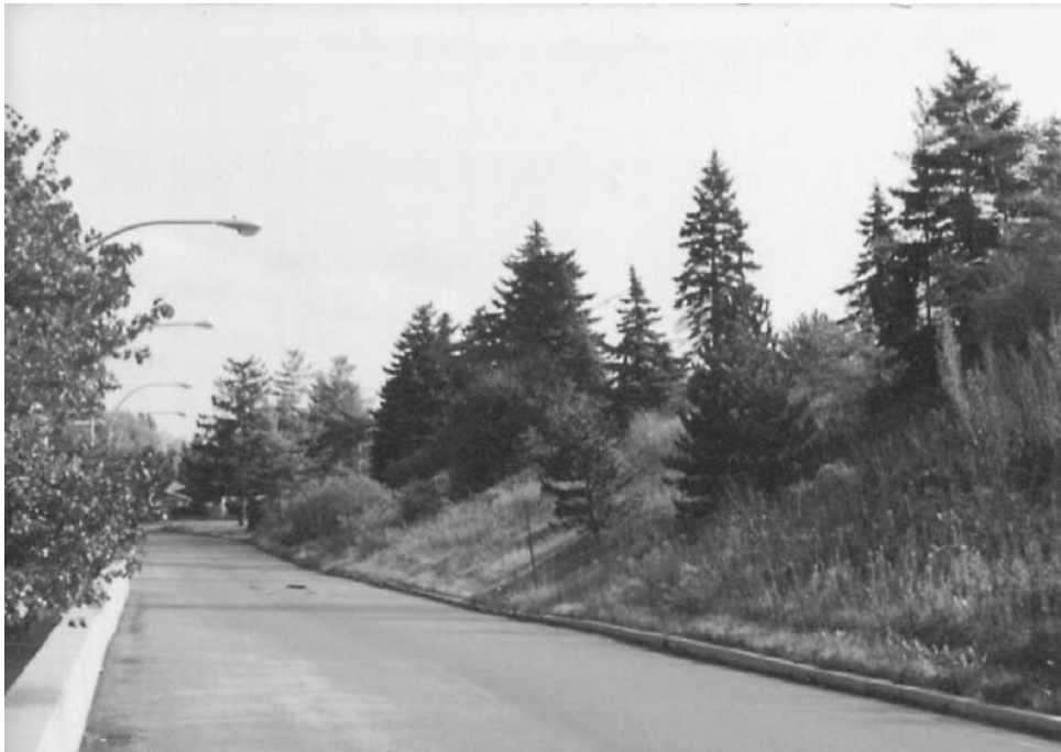
Figure 7.3 Photograph of trees planted on a slope as part of a stabilization plan.
