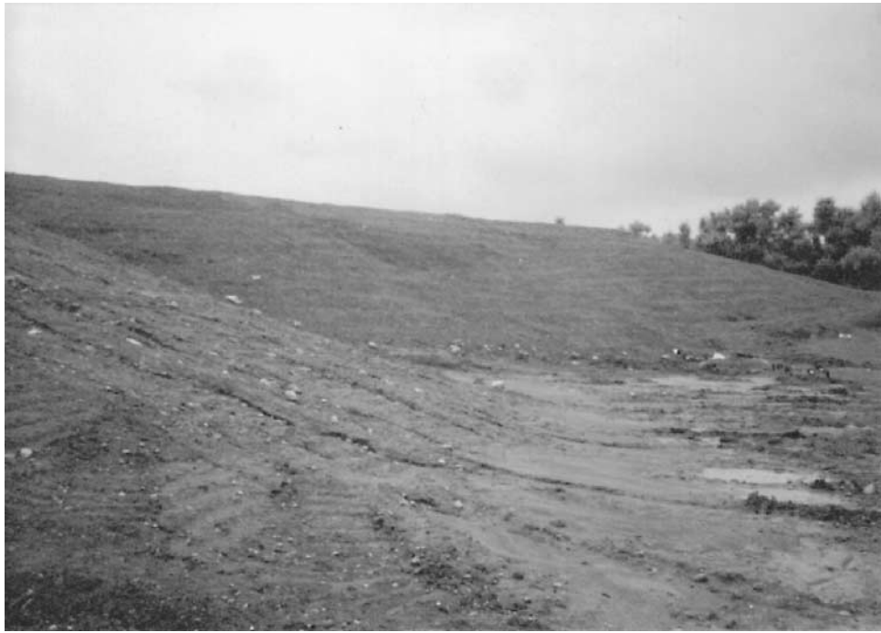
Figure 7.2 Photograph of tracking on a slope.
