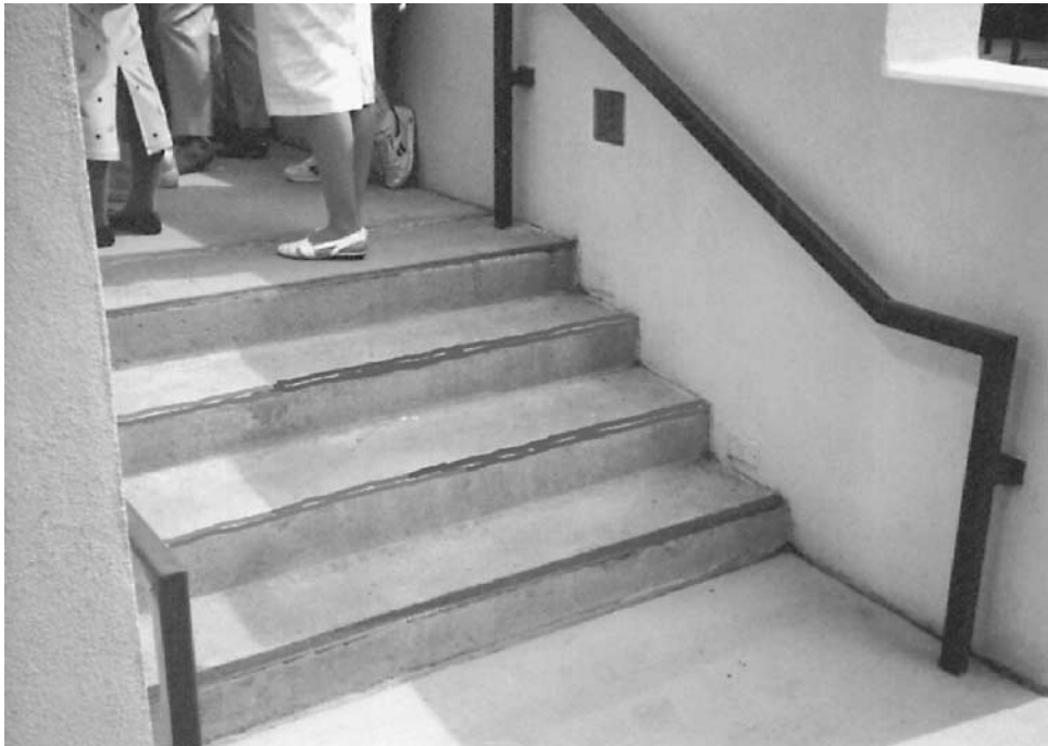
Figure 4.6 Photograph of stair treads with painted nosing.
