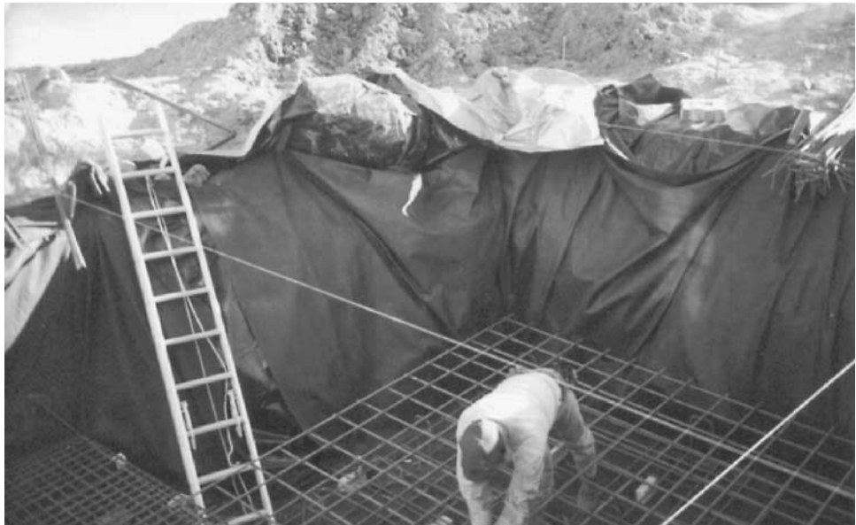
Figure 7.31 Photograph of lined foundation excavation.
