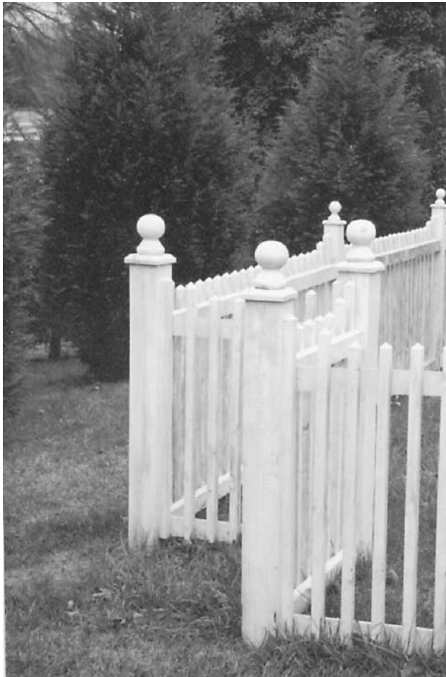
Figure 4.53 Photograph of picket fence corner detail.
