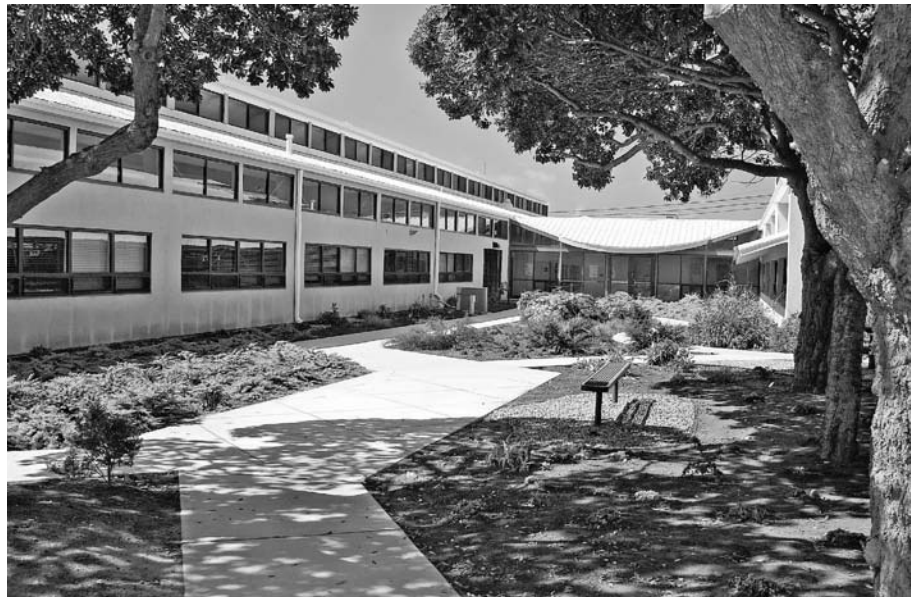
Home to the Naval Base Ventura County Public Works Department, consisting of 10,000 square feet of renovated space and 7,000 square feet of new construction.
