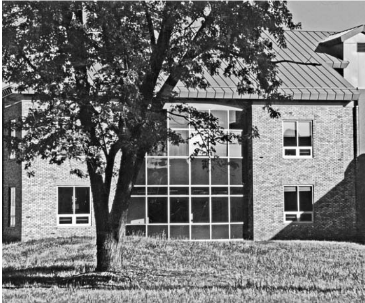
Sustainable-design elements on the 3.4-acre inner-city brownfield site redevelopment of The Green Institute's Phillips Eco-Enterprise Center include geo-exchange heating and cooling, sun-tracking daylighting, air-to-air energy recovery, salvaged steel joists, wood, and brick.
