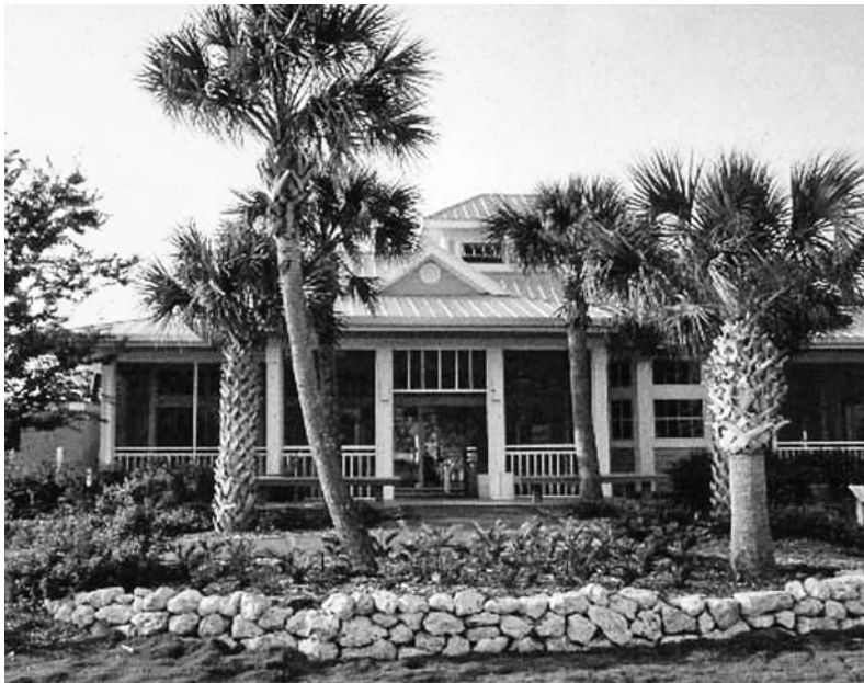
Florida House Learning Center is unique as a public and private partnership for a sustainable model home and yard for the public to visit.
