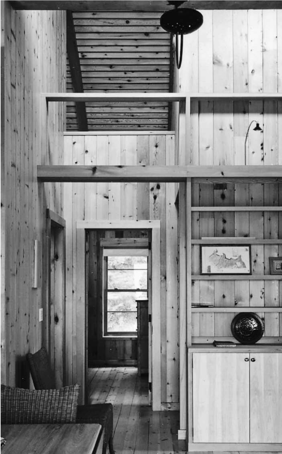
Natural stack ventilation through low and high windows cools the cabin. An air-to-air heat exchanger provides ventilation.
