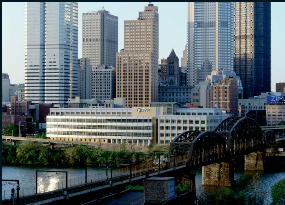
PNC Firstside Center. Energy costs at PNC Firstside are 50 percent lower than the conventional building's and employee retention has improved 60 percent. Photography by Ed Massery.
