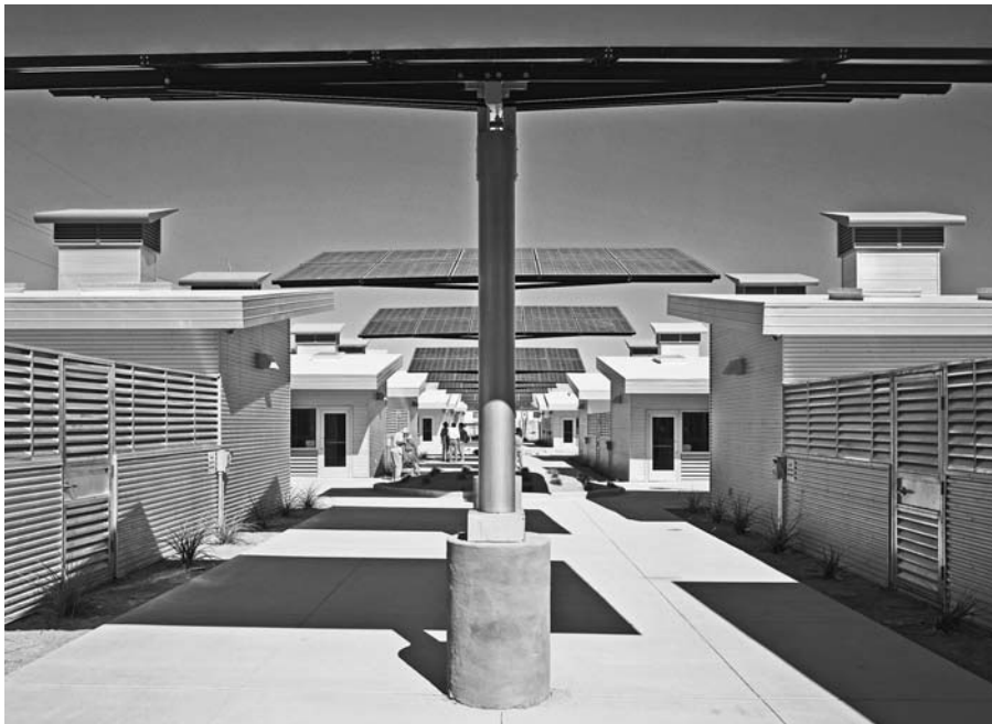
The space between kennels at the Animal Foundation Dog Adoption Park is shaded by canopies of photovoltaic panels.
