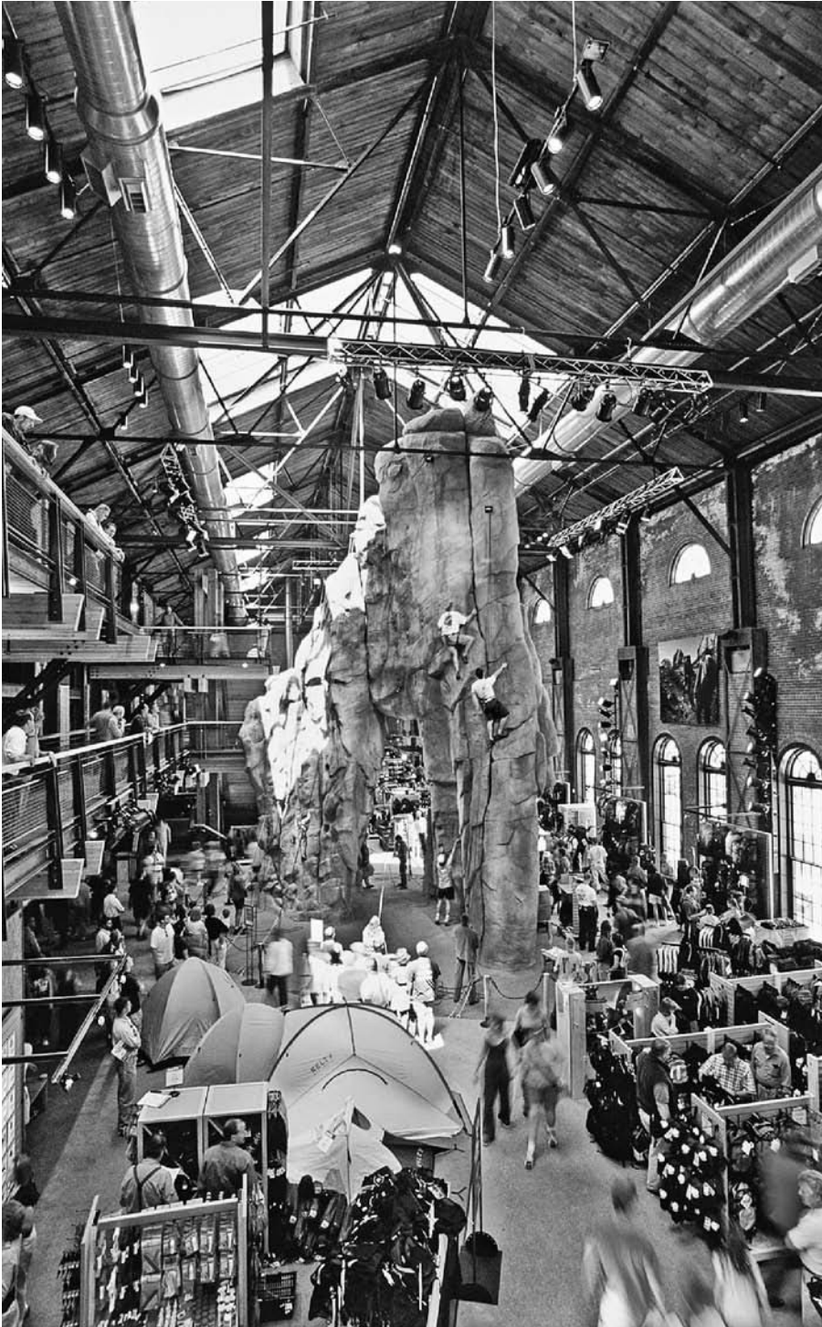
At REI Denver, reclaimed wood timbers, salvaged from an abandoned mine, were used for stair supports, and reclaimed wood decking was used for a new second-floor structure.
