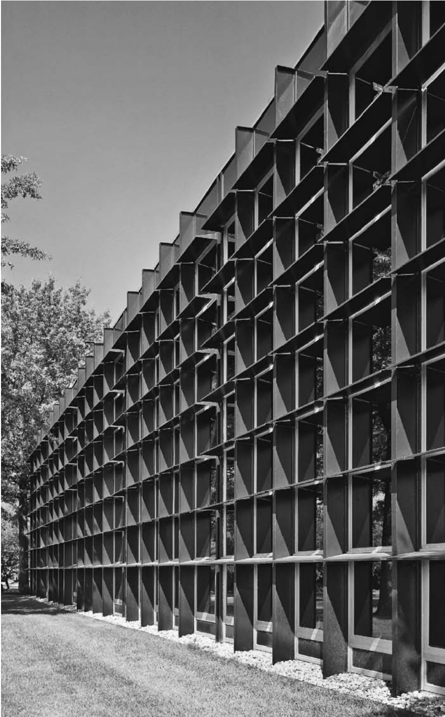
Herman Miller Building C1 is an example of smart reuse of a building, which is one of the most sustainable strategies available.
