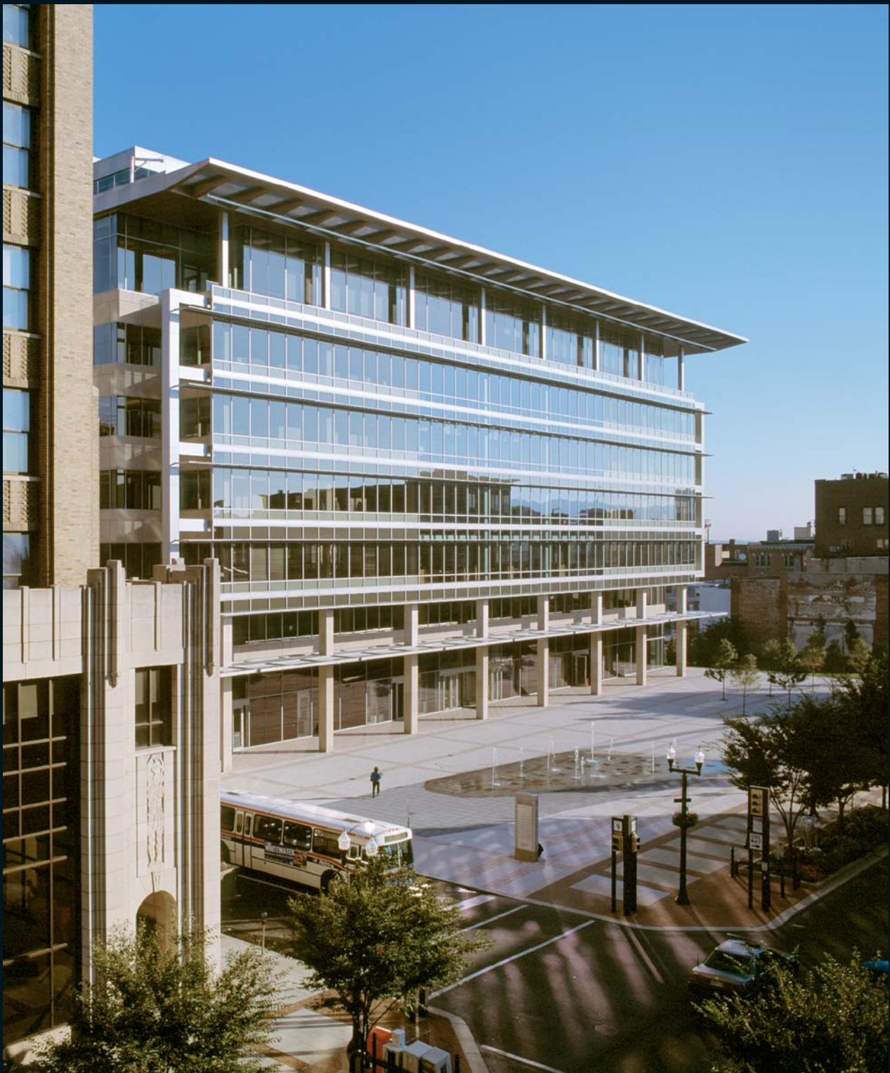
The Plaza at PPL Center. An eight-story glass atrium brings natural light deep into the core of the building, while extensive perimeter glazing provides panoramic views and abundant daylight, filtered through brises-soleil, directly to all building spaces. Copyright Peter Aaron/Esto.
