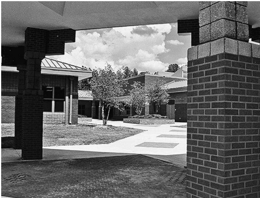
Durant Road Middle School is the first school in the county to comply with ASHRAE's 15 cubic feet per minute (cfm) per-person guideline.
