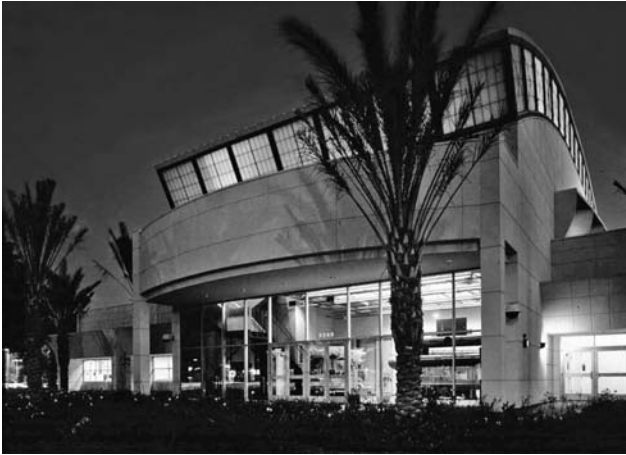
The Energy Resource Center by WLC Architects acts as a showcase building, integrating not only top-quality energy strategies but also environmental material choices and indoor environmental quality elements.
