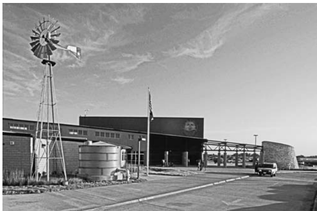
The design of Malvern Elementary School by SHW Group, Inc. illustrates multiple elements for a pilot sustainable school.
