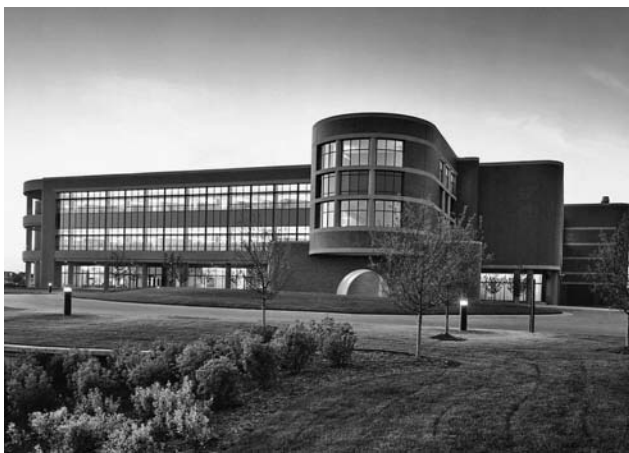
The SC Johnson Wax Commercial Products building designed by Zimmerman Design Group and Hellmuth Obata + Kassabaum (HOK) serves as a benchmark for environmentally responsible design and construction.
