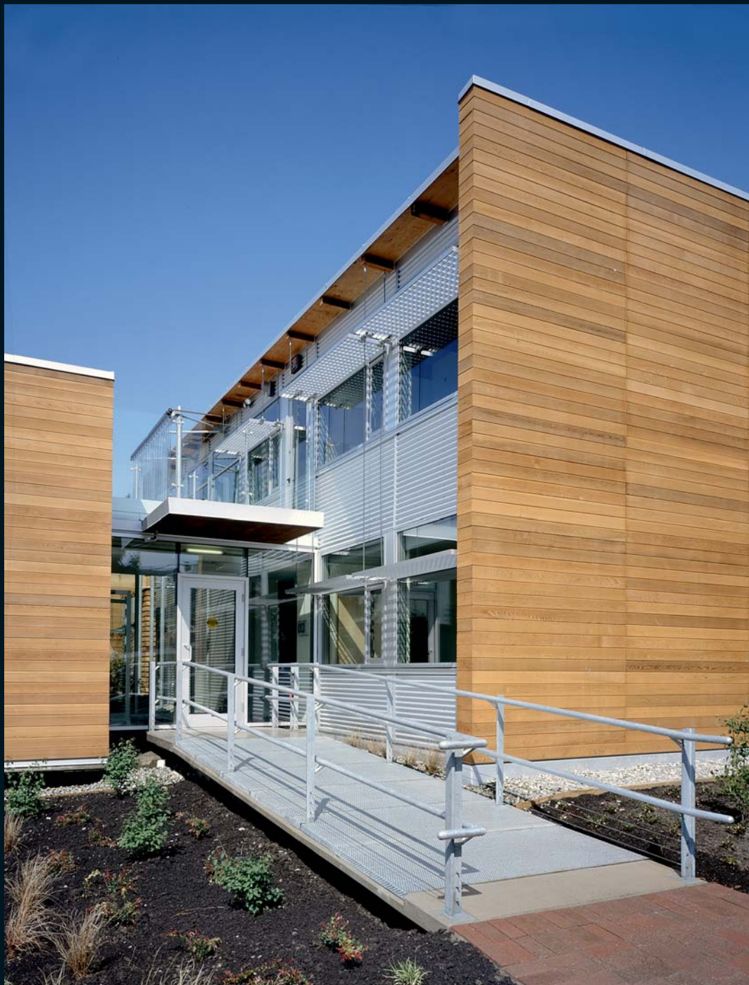
City of White Rock Operations Building. Daylight light shelves provide balanced daylight and reduce electric lighting needs. A green-sod roof reduces runoff from impermeable surfaces, while a pervious parking lot allows infiltration of water into the ground. The facility also uses stormwater rather than potable water to wash city vehicles and for toilets, and waterless urinals and low-flow faucets throughout the facility further reduce water consumption. Extensive use of materials produced within a 500-mile radius of the site also reduced transportation effects on the environment. Photo by Colin Jewell.
