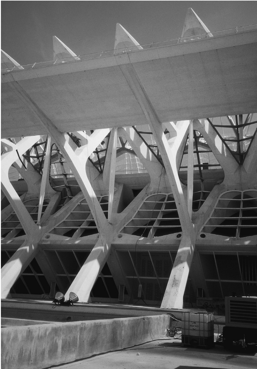
Figs. 2.6–7 City of Arts and Sciences, Valencia, Santiago Calatrava: skeletal structure.
