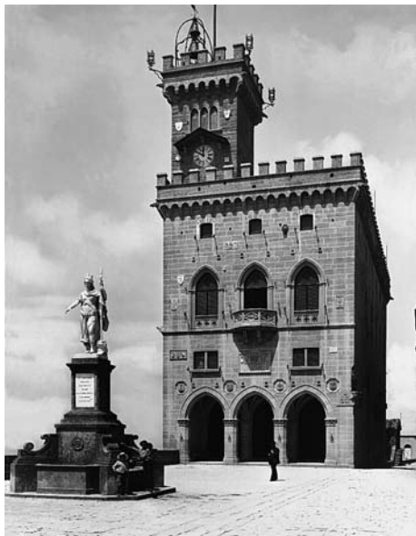
4.17 Alfonso Rubbiani, Via del Santo Stefano houses restoration project, Bologna, 1904. Ink drawing on a photograph by Pietro Poppi 4.18 Francesco Azzurri, Palazzo Pubblico, San Marino, 1884–94
