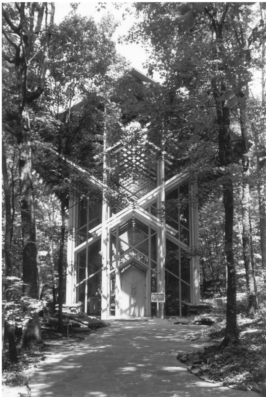
FIGURE 12. Thorncrowne Chapel, Eureka Springs, Arkansas, exterior. Photograph courtesy of The Arkansas Historic Preservation Program.
