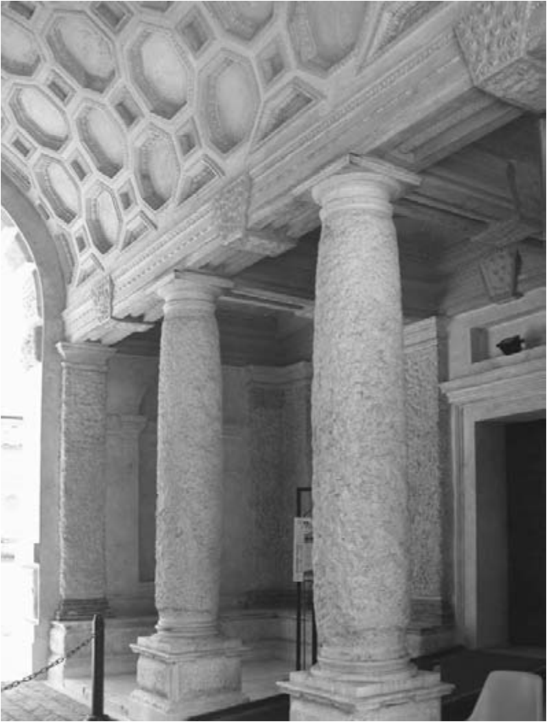
Palazzo del Te, a grotto-like entrance passageway with roughened columns and rugged coffering.
