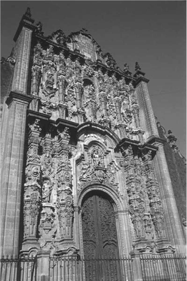
Lorenzo Rodriguez, Sagrario, Mexico City, 1740–68, the parish church attached to the cathedral, view of side facade; though based on classical elements like columns, each unit is multiplied or subdivided until no longer recognizable.
