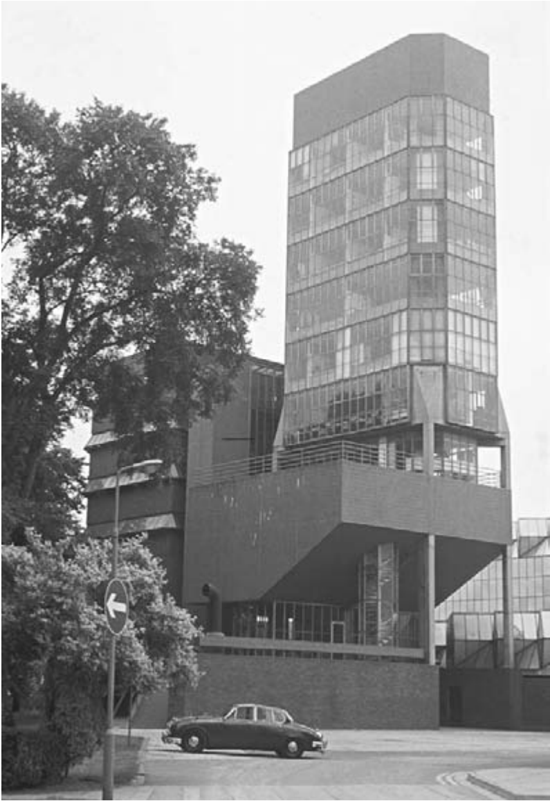
James Stirling and James Gowan, Engineering Faculty, University of Leicester, 1959–63, Constructivist ideas of form and materials surface 45 years later in different political circumstances.
