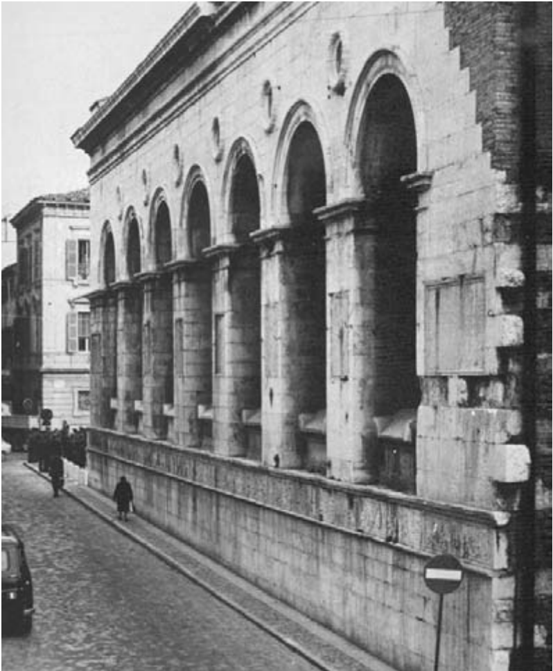
Leon Battista Alberti's Tempio Malatestiano, Rimini, where he modernized an existing building by referring to antique precedent: side wall furnished with sarcophagi, echoing pagan shrines, from 1450.
