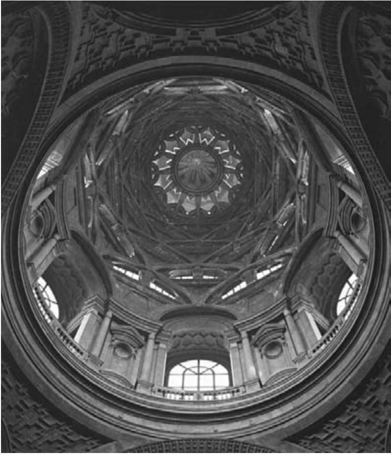
Guarini, Chapel of the Holy Shroud, attached to the Cathedral, Turin, 1667–90, a further development of the dome broken into segments and lit in many increments to create effects of baffling complexity.
