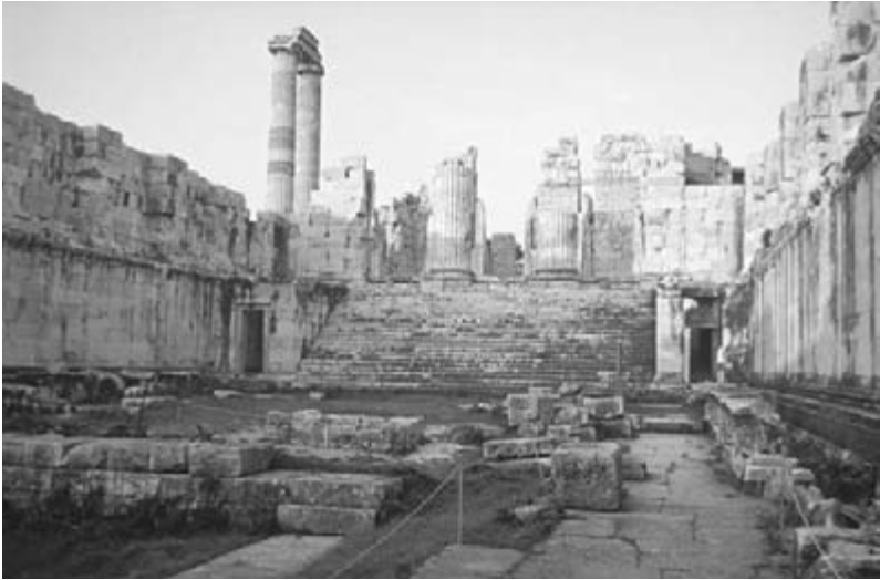
Didyma, Temple of Apollo, 3rd century BC and later, interior, which was always unroofed, looking back toward the platform of the oracle and two symmetrical entrance passages.
