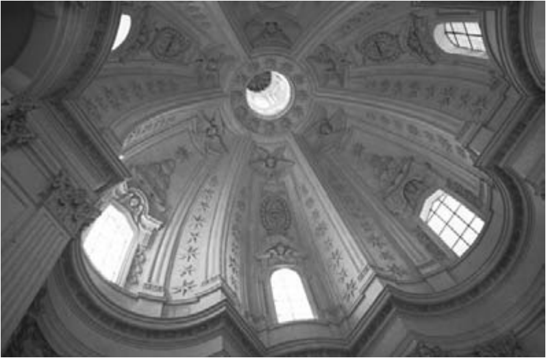
Borromini, Sant' Ivo della Sapienza, view into the dome showing the two geometries of the plan in their clearest manifestation.
