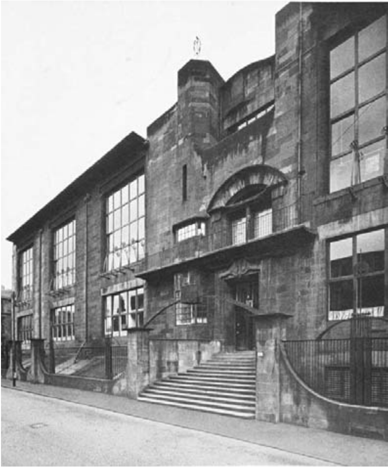
C. R. Mackintosh, Glasgow School of Art, 1897–9, 1907–9, north-facing studio windows along the street facade; a Scottish castle vernacular tending toward Art Nouveau incorporates the British functional tradition of iron and glass.
