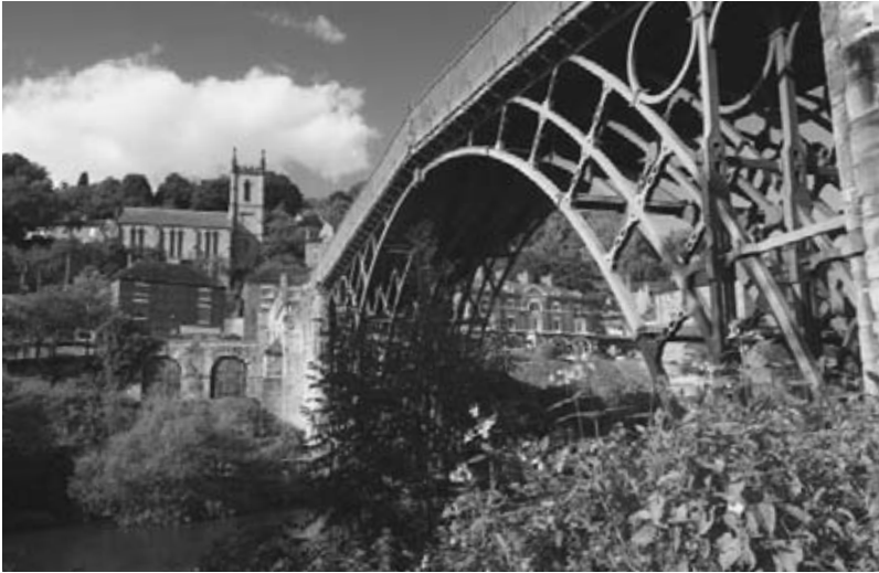
Ironbridge near Coalbrookdale, Shropshire, 1777–80, an early example of iron construction, lighter and cheaper than masonry, engineering edging out architecture.
