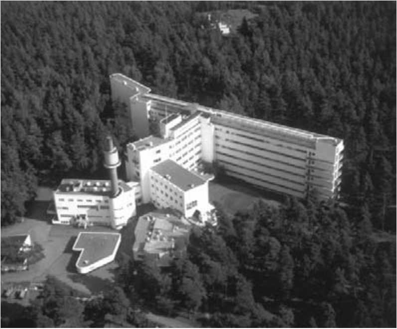
Alvar Aalto, Paimio sanatorium, Finland, 1928–32, with clearly distinguished functions and elements dictated by methods of treating tuberculosis, like the long south-facing flank.
