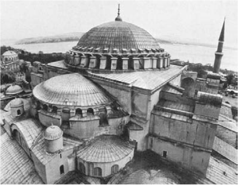
Hagia Sophia, Istanbul, 532–7, view of roofs from a minaret.
