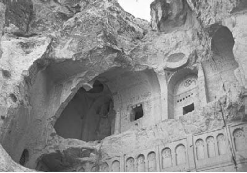
12th-century rock-cut church in Cappadocia, from which roof, floor and a whole side wall have fallen away, revealing the fictitious nature of the structure more clearly.
