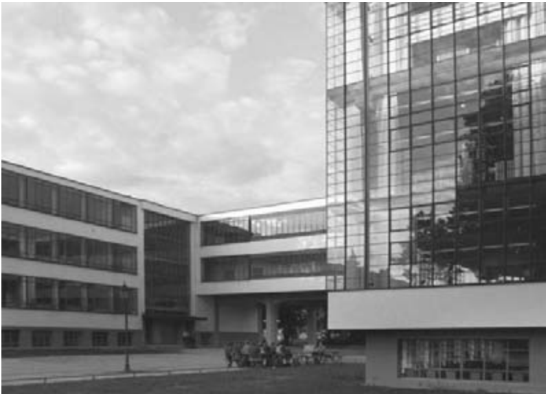
Walter Gropius and Hannes Meyer, Bauhaus, Dessau, 1925–6; glazed corners (walls detached from the system of support) in the workshop wing of this radical art school.
