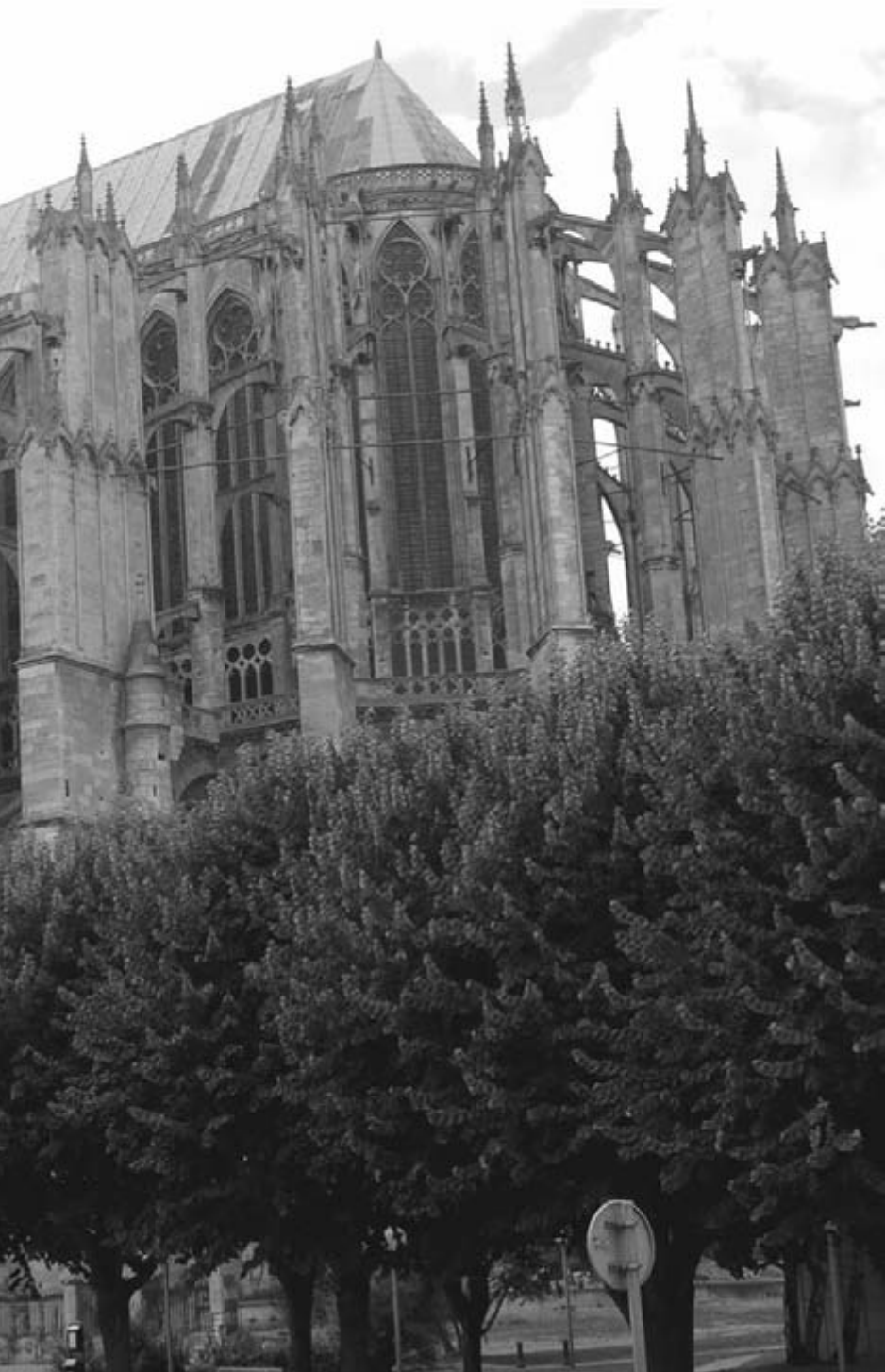
Beauvais Cathedral from the south-east showing the exo-skeleton of flying buttresses that makes the high walls of glass possible, choir rebuilt 1284–1338.
