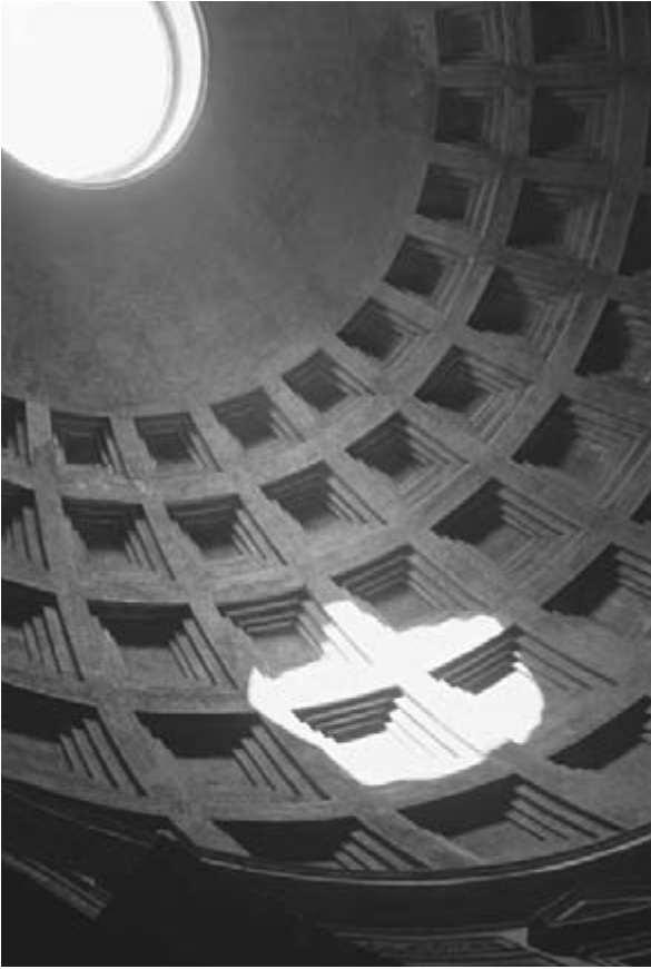
Pantheon, Rome, c. AD 118–28, curve of dome overhead, on which the path of the sun is traced by a circle of light admitted by the oculus, the only aperture in the great hemispherically domed cylinder.
