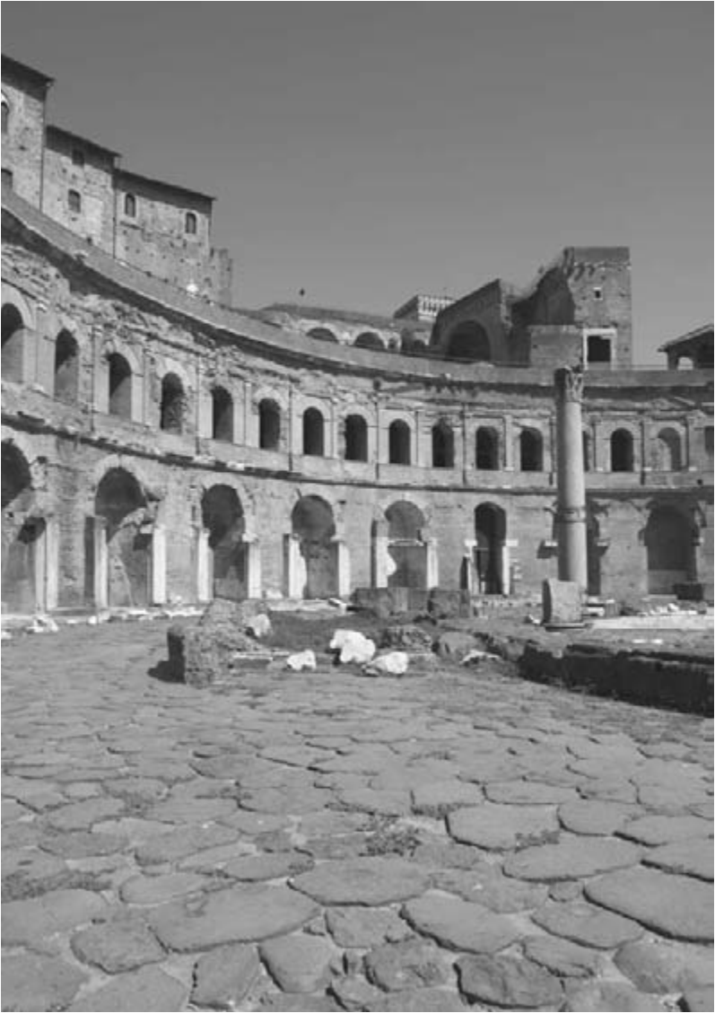
Trajan's Market, Rome, brick-faced concrete trimmed in travertine, c. AD 110–12. This ceremonial front facing Trajan's Forum conceals the varied scales and everyday functions of the complex.
