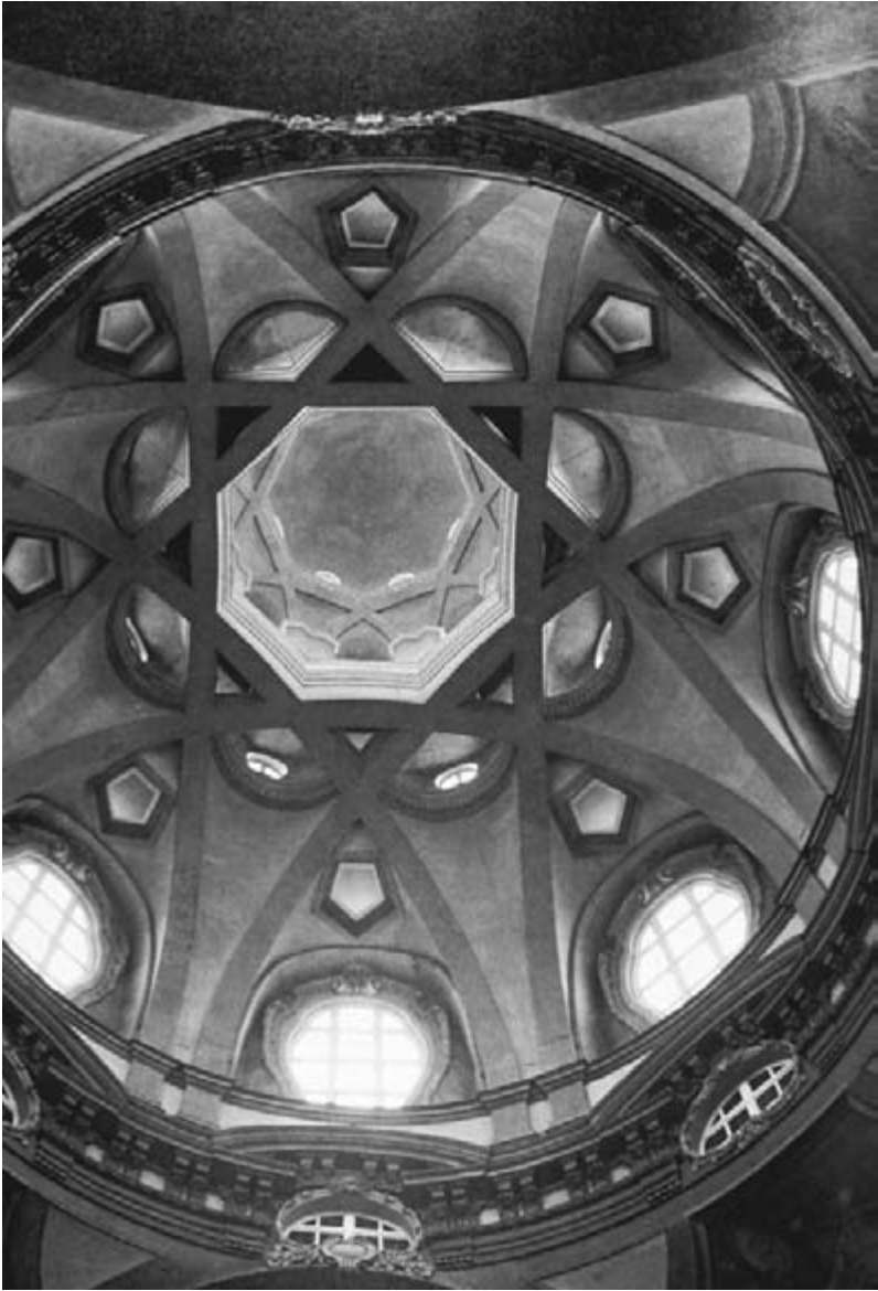
Guarino Guarini, San Lorenzo, Turin, 1668–80, view into a dome that is like a mathematical puzzle which fractures space by allowing bursts and slivers of light to illuminate the fabric in a variety of ways.
