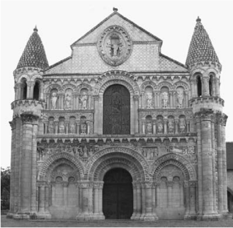
Notre-Dame-la-Grande, Poitiers, facade whose arcades are framed by overscaled derivatives of classical orders and whose surface is carved with a rich jumble of scenes in relief, second quarter of the 12th century.
