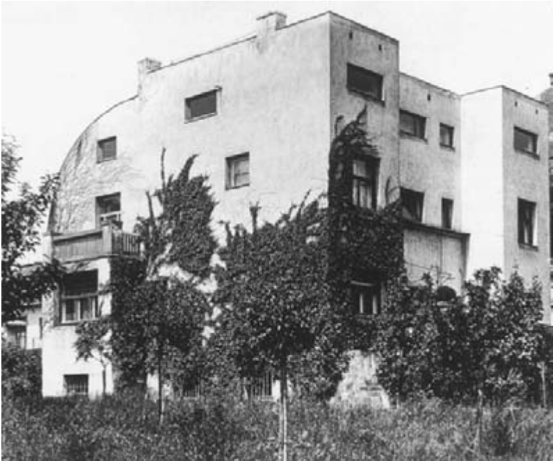
Adolf Loos, Steiner House, Vienna, 1910. An austere exterior of hard-edged rectangular forms.
