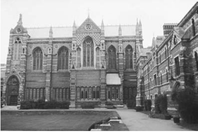
William Butterfield, Keble College, Oxford, 1868–82, view of chapel and buildings along the street front, inexpensive industrial brick used in variegated patterns as an analogue of medieval carved detail.
