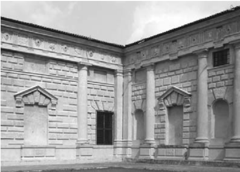
Giulio Romano, Palazzo del Te, Mantua, studious disruptions of classical norms, including dropped triglyphs, blind windows and pseudo rustication, 1527–34.
