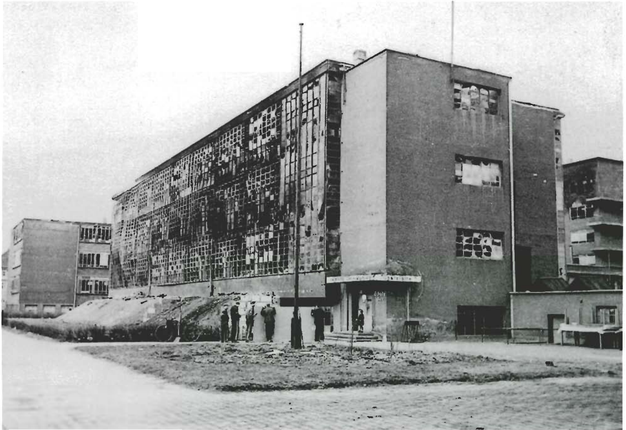
The workshop wing in 1945, with earth rampart and damage after a blaze caused by fire-bombs. Writing above the door: "Gaststätte Seminarplatz" / „Gaststätte“, under that: „Schade-Biere“/ „Schultheiss-Bier(e)“. The north wing after the air-raid in March 1945.
