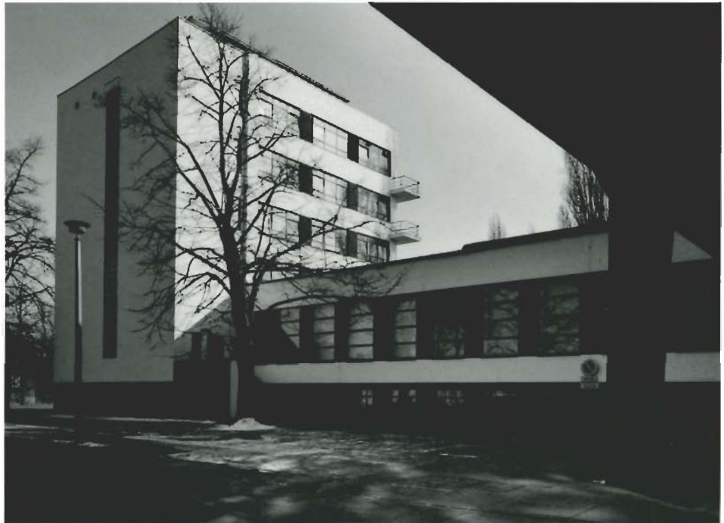
View from the bridge of the studio building and the intermediate section with refectory and stage, and east view, photographs by Dieter Rausch, 1993.
