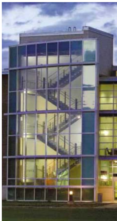
Sun control curtain wall, concealed vents and storefront at the Massachusetts Maritime Academy. Courtesy VistaWall.
