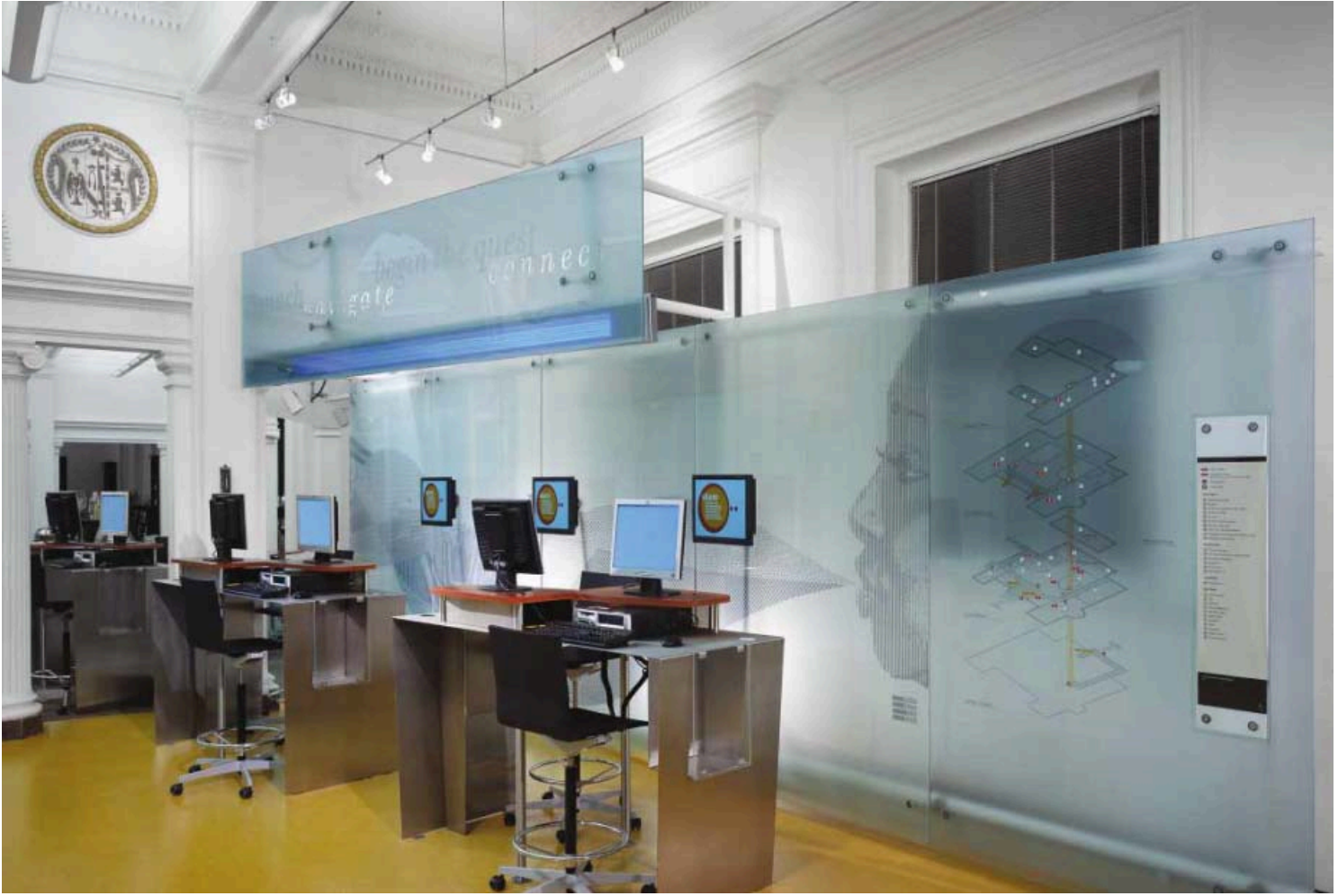
The display system consists of single and double layers of 3/4-inch-thick glass panels supported by a steel framework (above and detail, left). In some cases, panels measuring 5 by 12 feet cantilever 5 to 7 feet.
