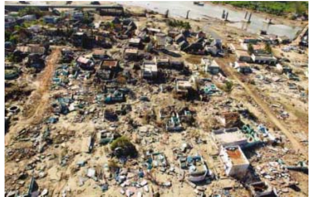
A village destroyed in India represents the rebuilding challenge.
