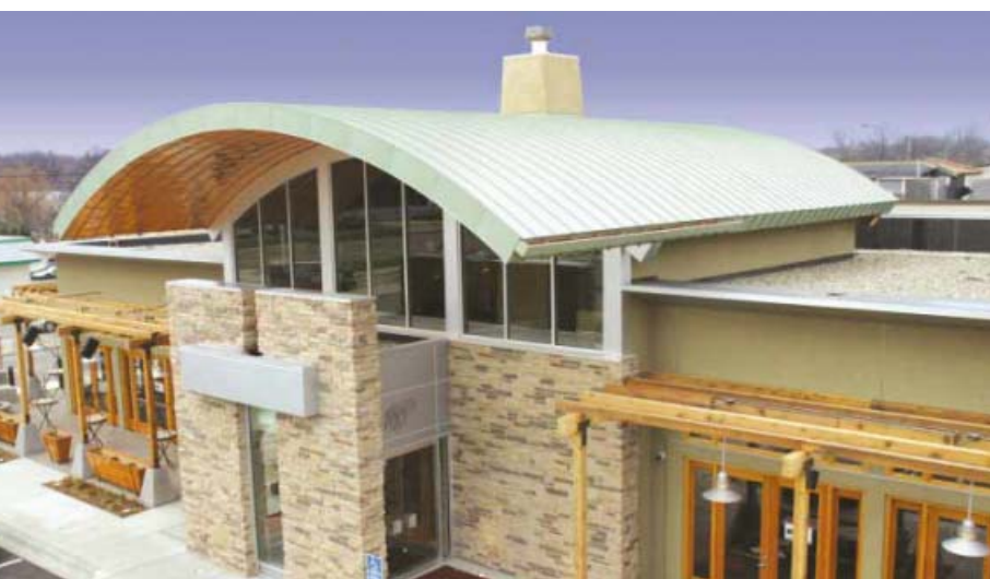
Copper roofing at Tryg’s Restaurant in Minneapolis, MN. Courtesy Revere Copper Products.
