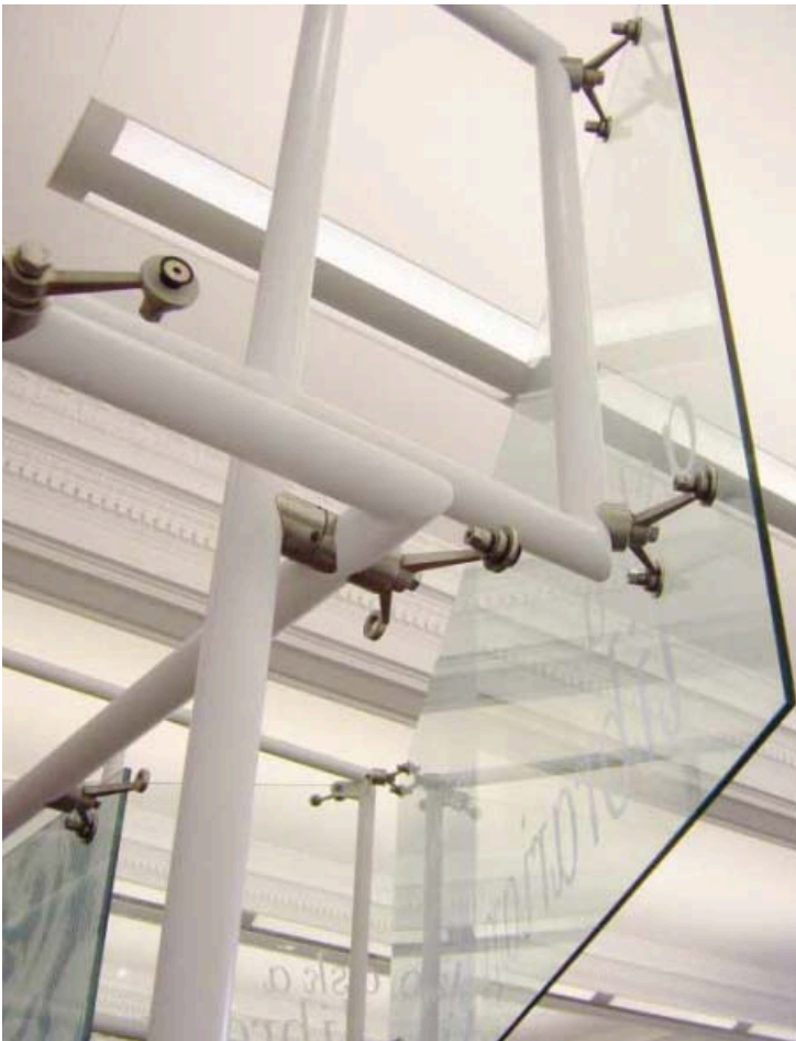
The display system consists of single and double layers of 3/4-inch-thick glass panels supported by a steel framework (above and detail, left). In some cases, panels measuring 5 by 12 feet cantilever 5 to 7 feet.
