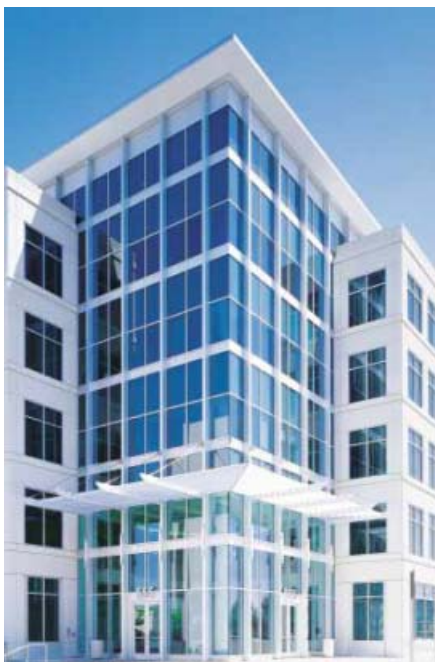
Sun control curtain wall. Courtesy VistaWall.
