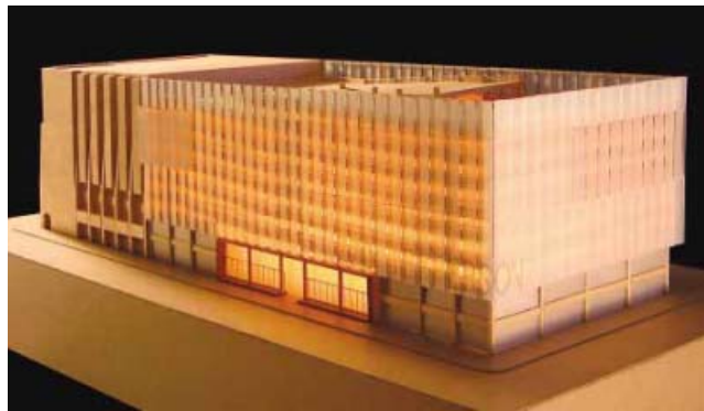
Downtown Garage, Milwaukee Currently in schematic design, this project's translucent panels will wrap around the seven-story ramp of a preexisting parking garage. During the day, the panels' appearance will change with the sun's intensity and angle; at night, the facade will be illuminated by a lighting system.
