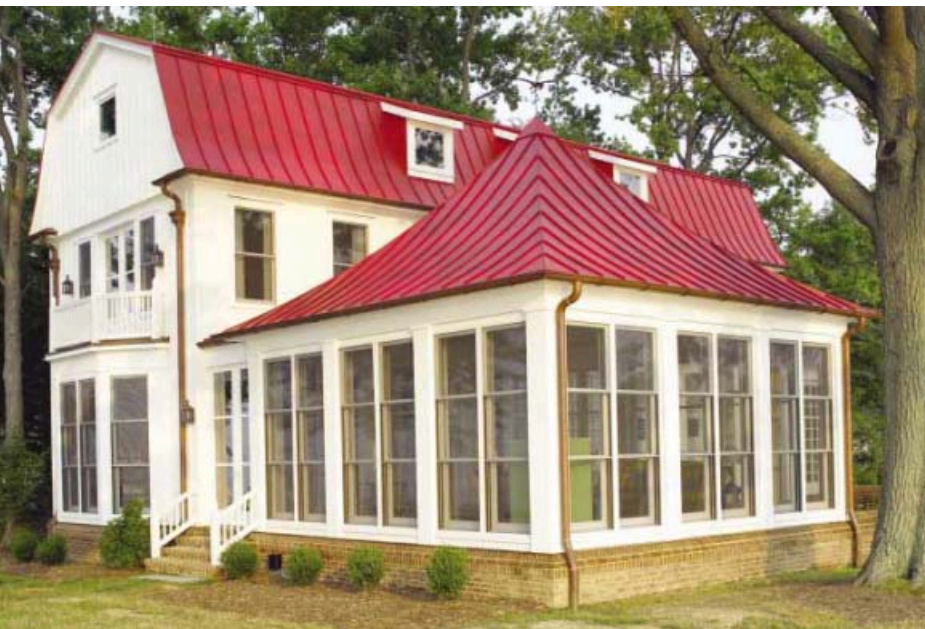
Zinc/tin roof, painted with solar reflective coatings. Courtesy Follansbee.
