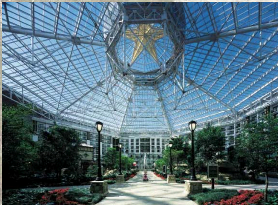
Atrium Skylight at the Gaylord Texan Resort & Convention Center. Courtesy VistaWall.
