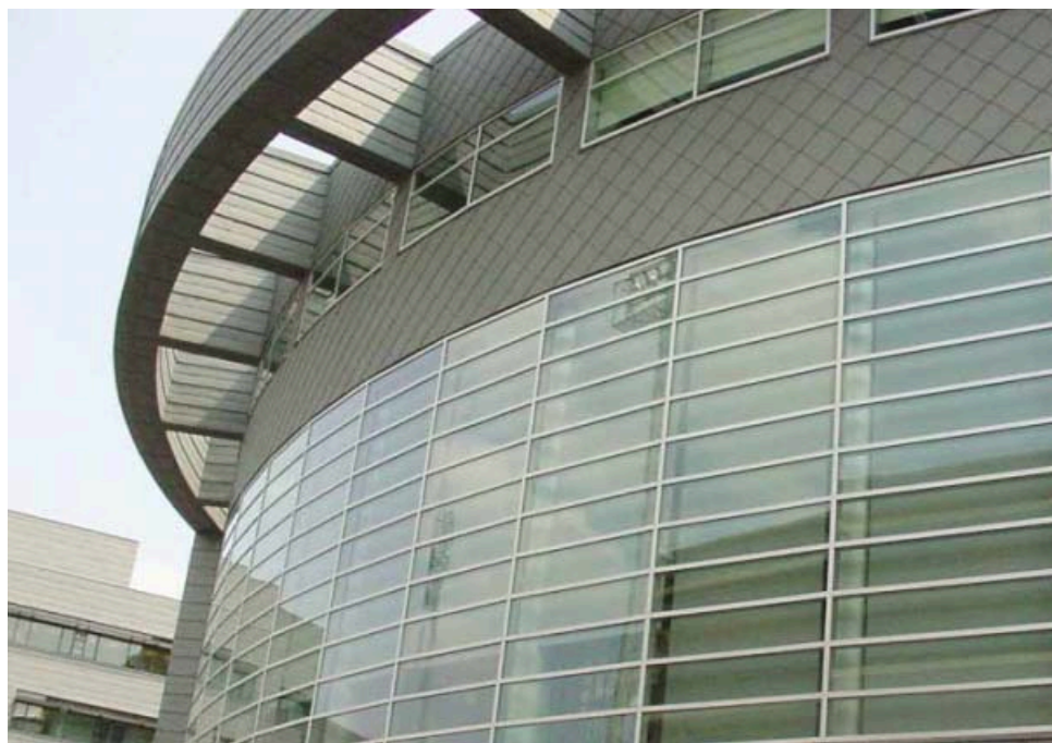
Zinc sunshade at the University of Cincinnati. Gwathmey Siegel Architects/GBBN Architects. Courtesy Umicore.
