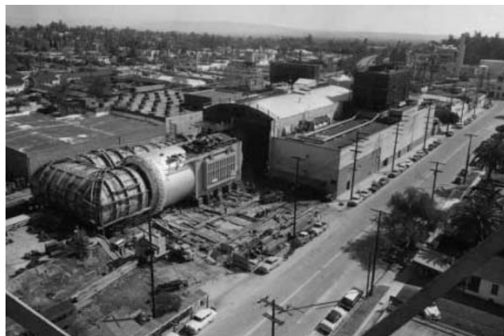
As documented in this historic photograph, the turbine was removed from the wind-tunnel building for a rare cleaning.
