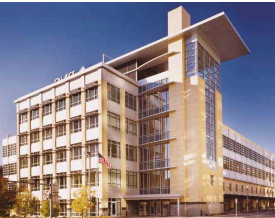
PNC Firstside Center. Courtesy PPG Glass.
