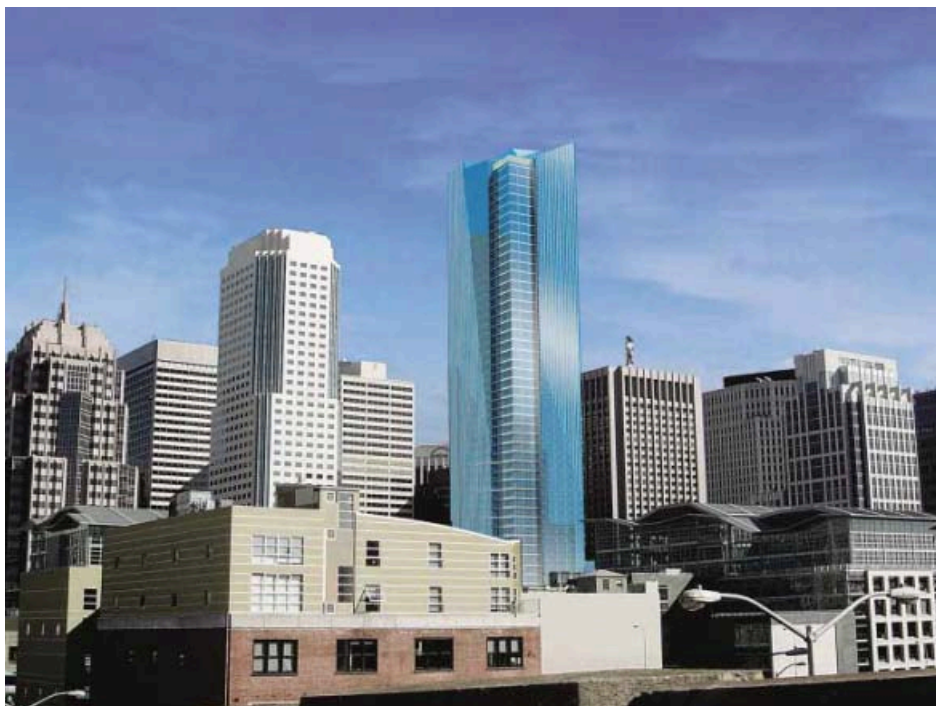
Noise levels were measured at ground level and at 120 feet above ground at the site of this 58-story multiuse tower in San Francisco, designed by Handel Architects.
