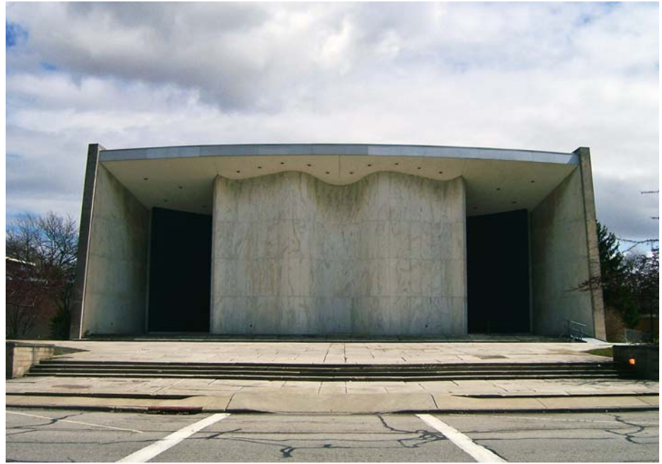
The top portion of the undulating stone façade has marks from a soffit that does not drip water away from the façade. Hall Auditorium at Oberlin College.
