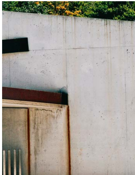
above and right Botanical Gardens in Barcelona, designed by Carlos Ferrater and completed in 1999. Elements of the park are constructed with Cor-Ten steel. The staining that occurs at the entrance almost looks deliberate.
