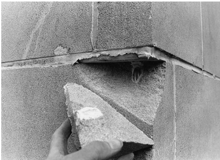
below Metro Dade Center. Corner cracks in stone.
