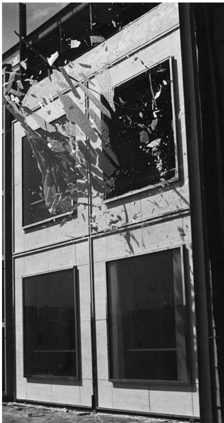
Glass failure at 4.3 MPa (90psf) pressure test on windows in façade mock-up.
