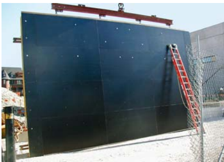
Fabrication of wood forms at Pulitzer Foundation, St. Louis.
