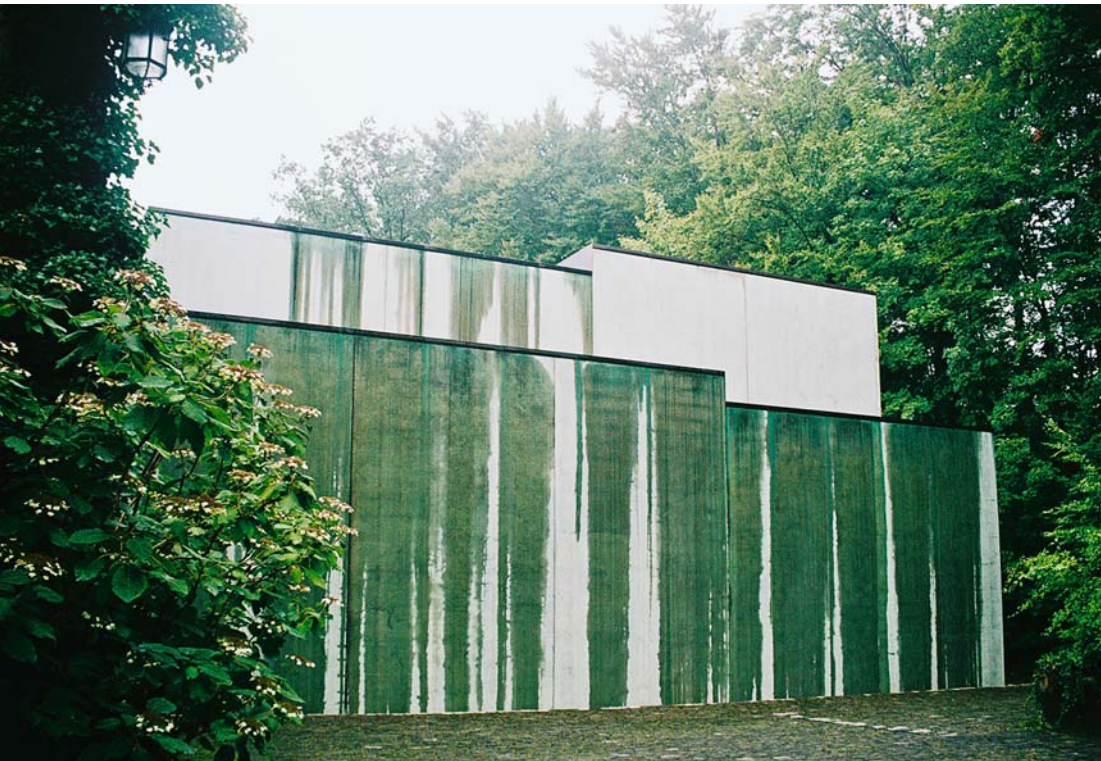
above Jurassic limestone and copper were added to the concrete panel mix to provide a green patina to the wall. Oskar Reinhart Collection, Winterthur, Switzerland, 1998.
