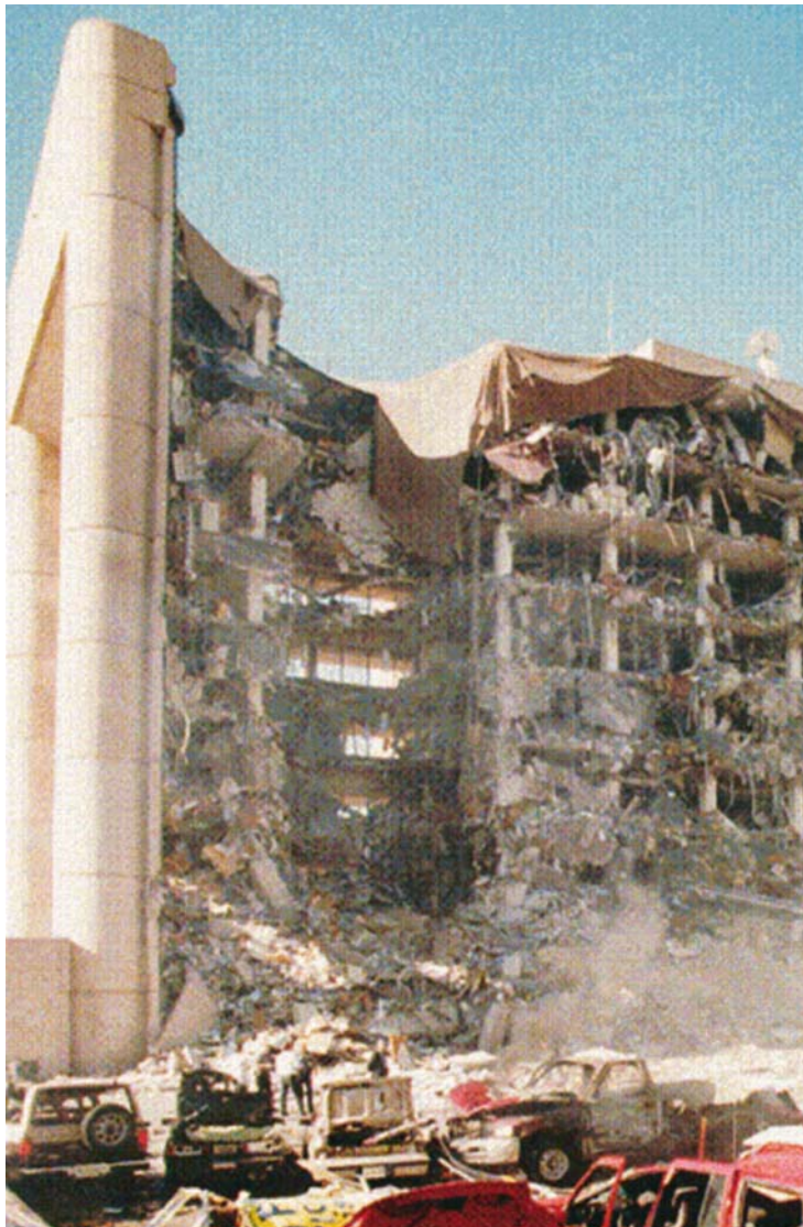
right and below Murrah Building, Oklahoma City. Façade destruction due to impact.
