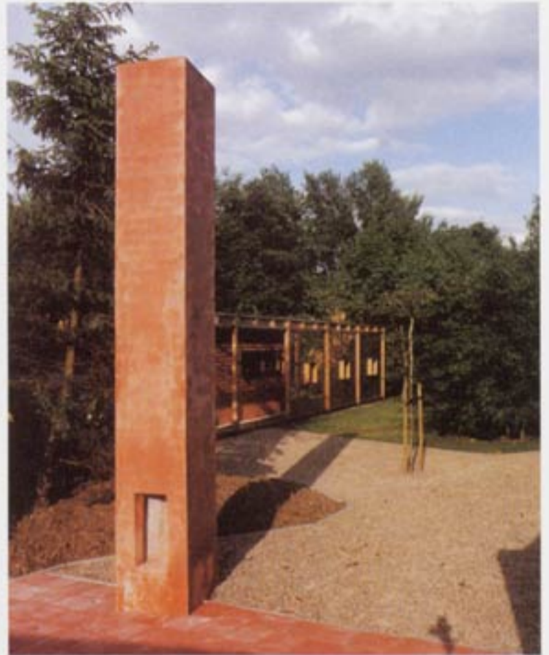
Vista de la terraza y chimenea Chimney and terrace view
