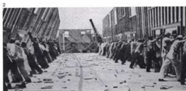
1. Casa Trubek & Wislocki/Trubek & Wislocki Houses, Nantucket Island, Massachusetts. Venturi, Scott Brown & Associates, 1970 2. Estructura de madera en entramado balloon frame/Timber frame of balloon frame structure 3. Casa y estudio Coxé-Hayden/Coxé-Hayden house and studio, Rhode Island. Venturi, Scott Brown & Associates, 1979 4. Splitting/Splitting, Matta-Cark, 1974
