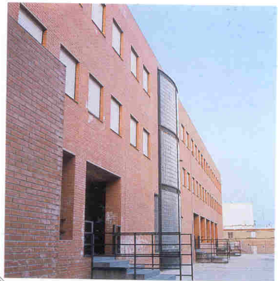
The south elevation, and axonometric showing the brick wall and the steel and glass cylinder.
