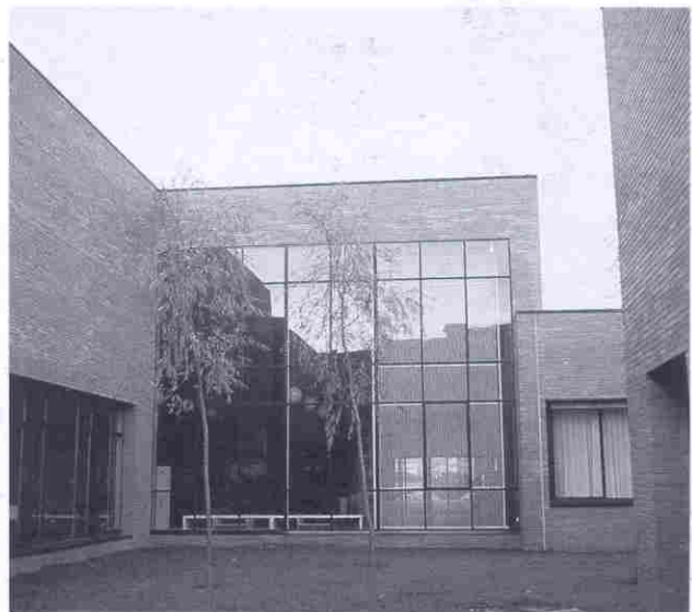
General view of school complex, plans of first and ground floors, and an internal courtyard.
