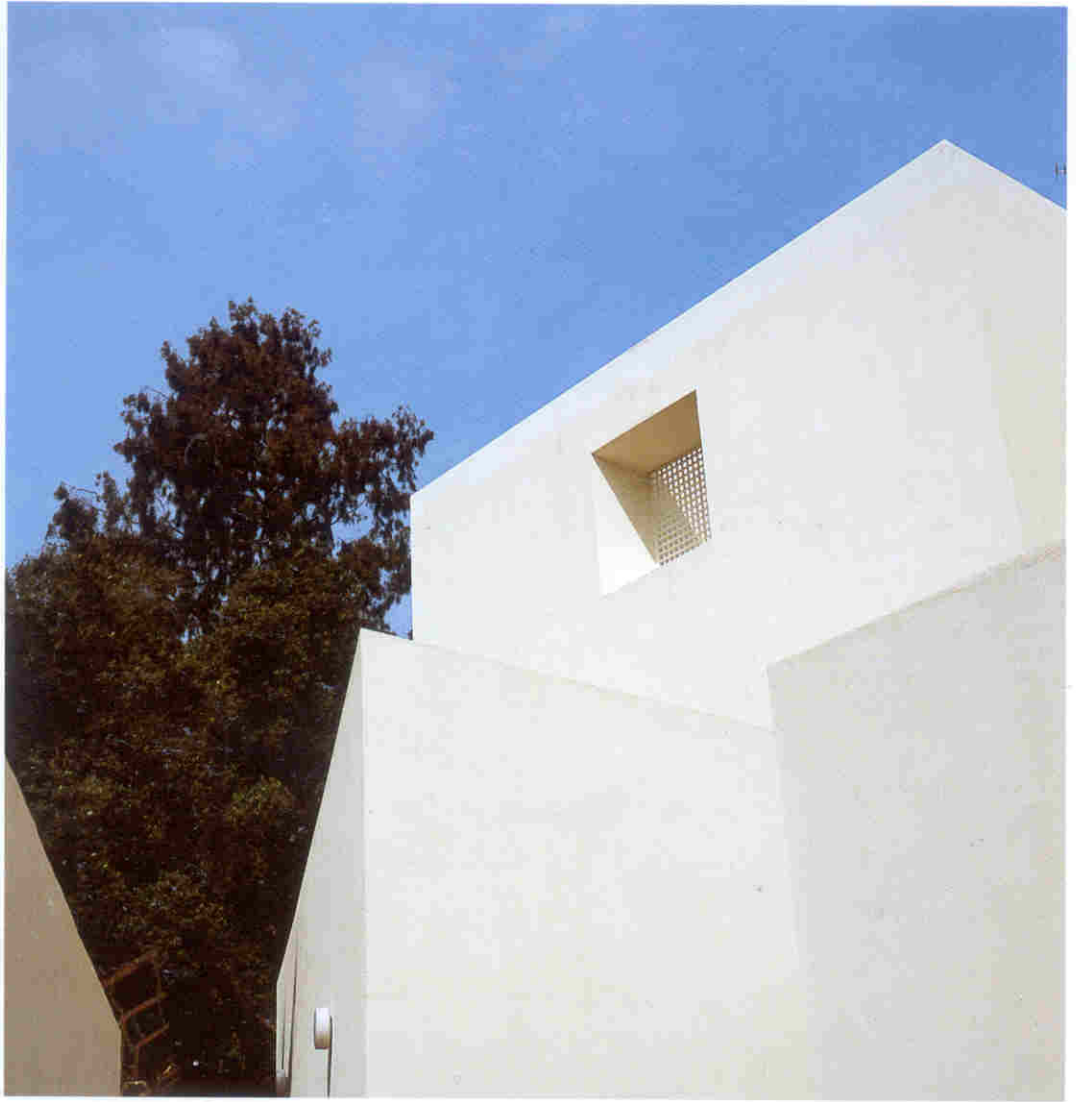
The interlocking volumes of one of the houses, and interior views.
