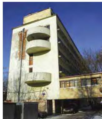
Largely ruined, Narkomfin is often the first stop that many visiting architects make in Moscow.
