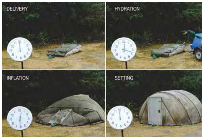
Concrete Canvas: Add water, use a battery-powered fan to inflate, and wait 12 hours.
