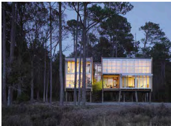
Mostly opaque on the three sides facing the woods (opposite), the house opens to the west (left) with views of the Chesapeake Bay.
