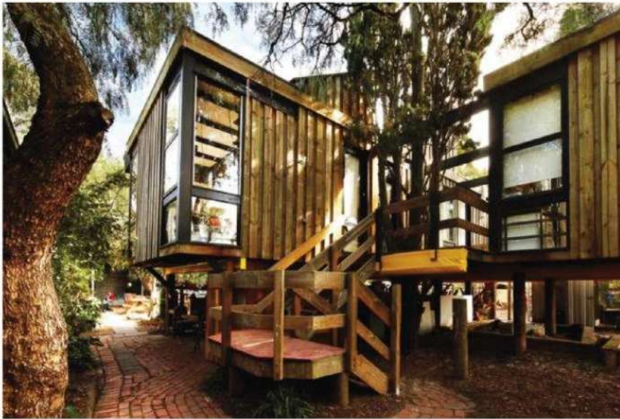
The 'tree house', constructed in 1965 – two elevated classrooms separated by a timber deck and an Italian Cypress.
