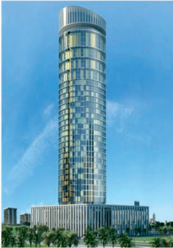
a new tower that stores solar power, which is used to rotate the building
