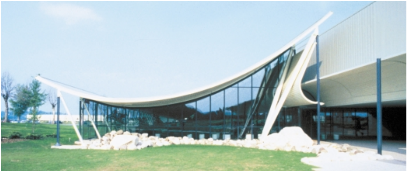
Lowara Company Offices, Vicenza, Italy — 1985
