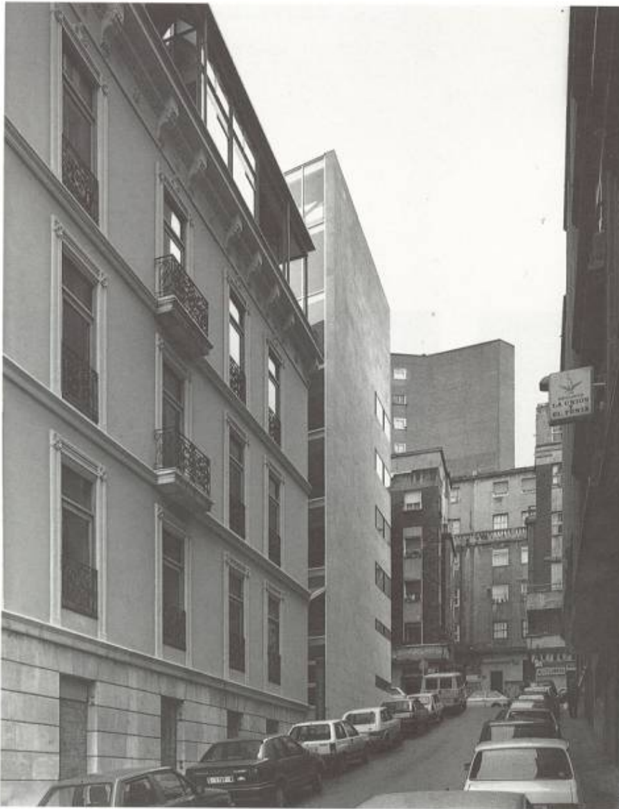
Vistas de los dos testeros desde la avenida principal Two views of both side elevations from the main street
