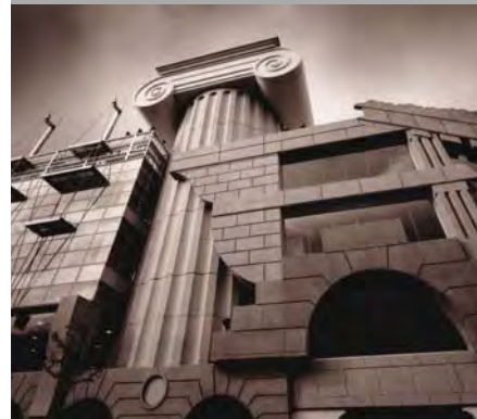
FIG. 11. M2 BUILDING, KENGO KUMA, TOKYO, 1991
