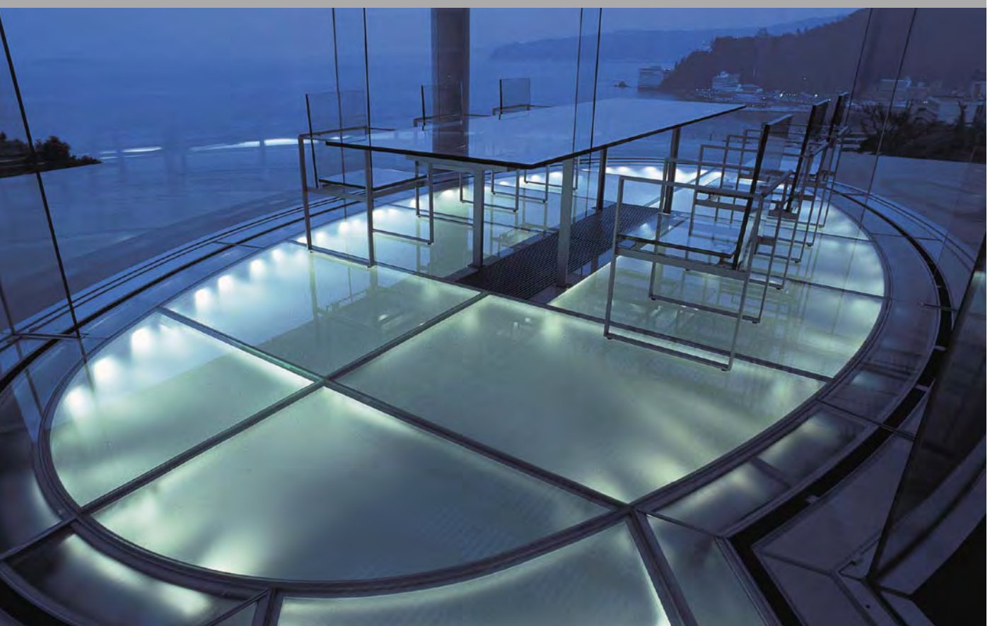
TOP / ROOF OF GLASS LOUNGE
