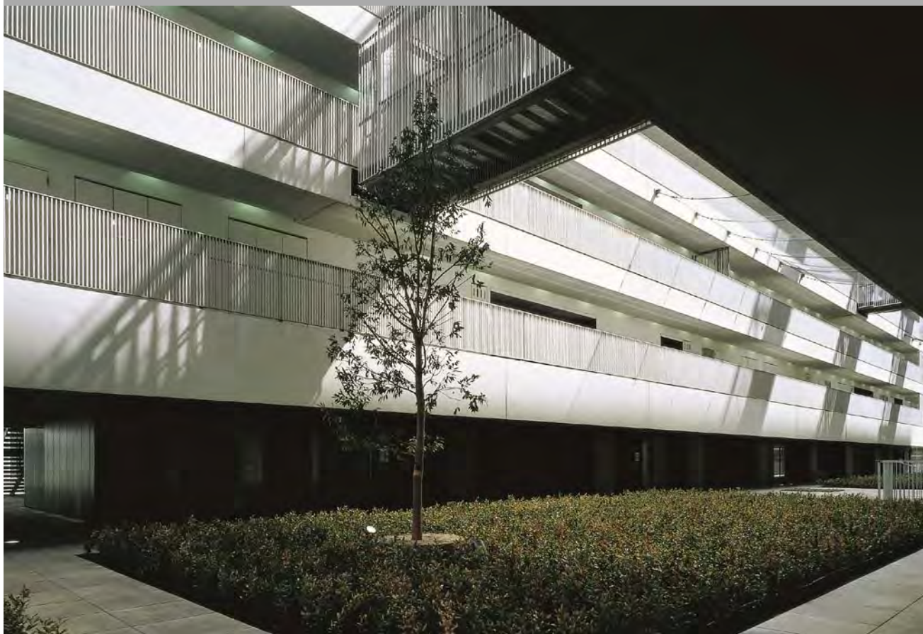
TOP / UPWARD VIEW OF INNER COURTYARD WITH CONNECTING BRIDGES BOTTOM / DETAIL OF PLANTED FLOOR OF COURTYARD
