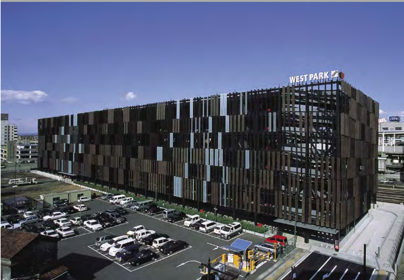
OPPOSITE / ELEVATION DETAIL TOP / AERIAL VIEW FROM THE SOUTH BOTTOM / VIEW OF FRONT FACADE
