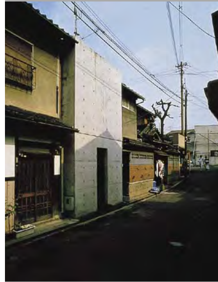
FIG 3. ROW HOUSE IN SUMIYOSHI (AZUMA RESIDENCE), TADAO ANDO, OSAKA, 1976
