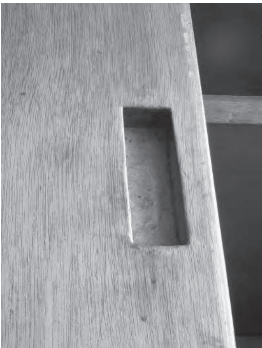
Figure 5.6 Cupboard door handles, studio of penthouse, 24 Rue Nungesser et Coli (1934)
