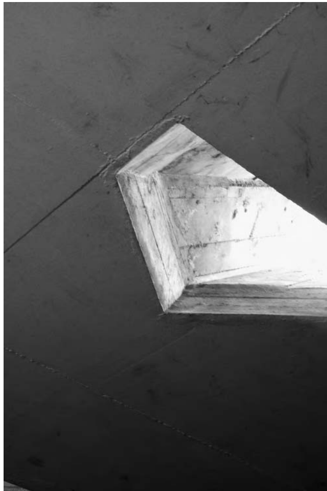
Figure 3.9 'Mitraillette' rooflights over the sacristy La Tourette (1959)
