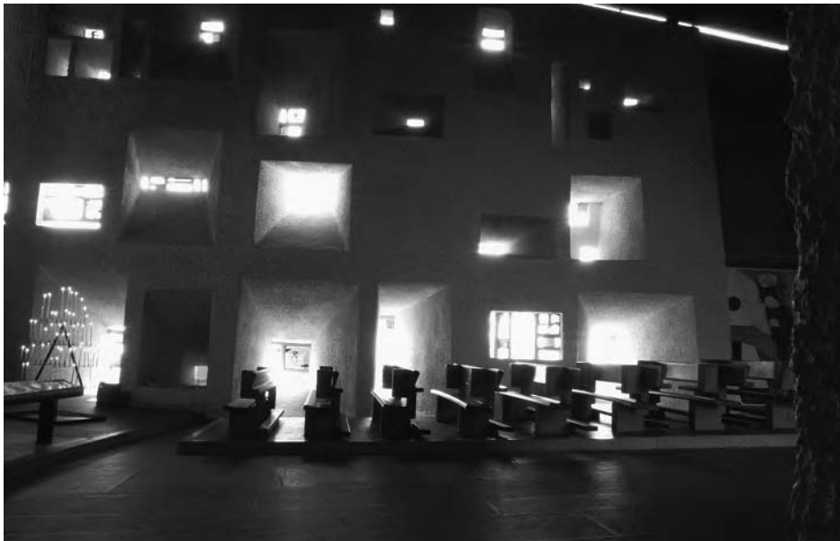
Figure 4.17 Chamfered windows south wall of Notre-Dame du Haut, Ronchamp (1955)
