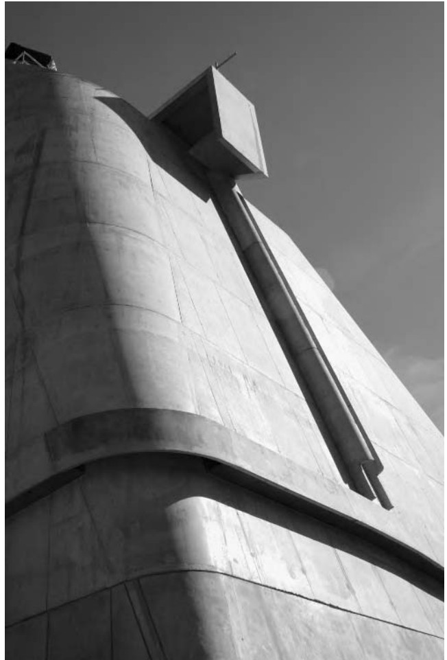
Figure 6.19 Detail of gutter, St- Pierre, Firminy-Vert (started 1960, completed 2006)
