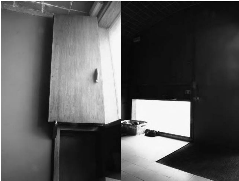
Figure 4.4 Shutters in Maison Jaoul B (1955)
