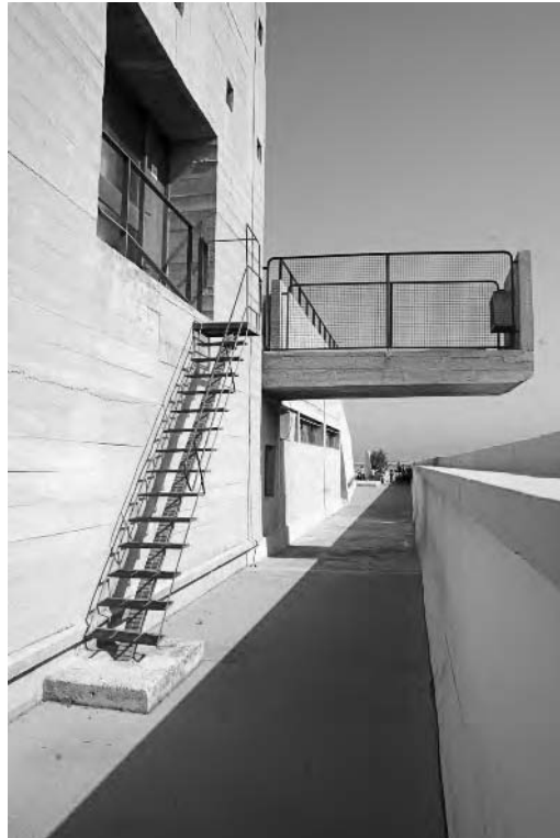
Figure 5.34 Stair up lift shaft on roof of Unité, Marseilles Michelet (1952)
