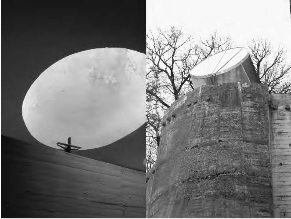
Figure 3.11 Rooflights over the Chapel of the Holy Sacrament, La Tourette (1959)
