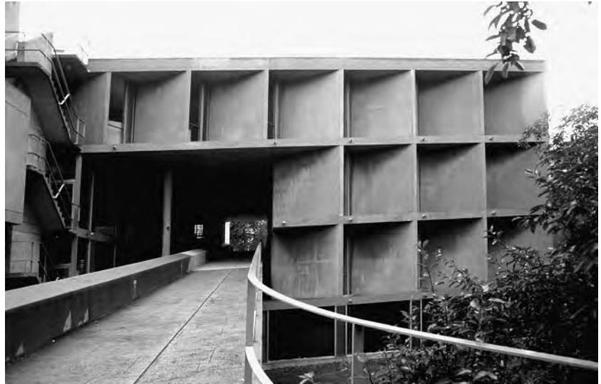
Figure 3.5 Brise soleil, Carpenter Centre, Boston, USA (1963)
