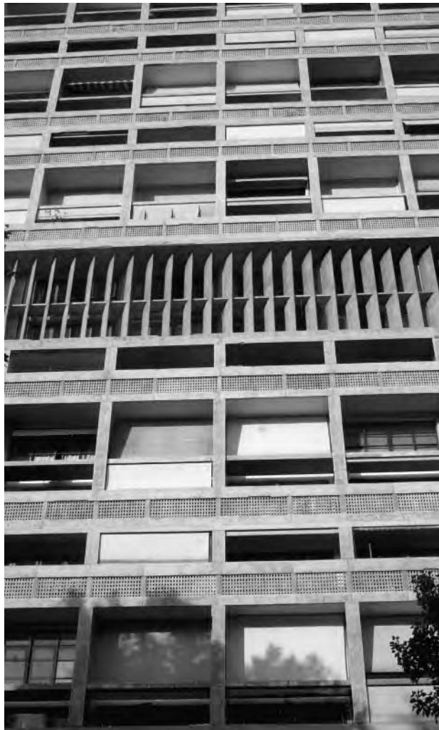
Figure 3.3 Brise soleil, Unité, Marseilles Michelet (1952)
