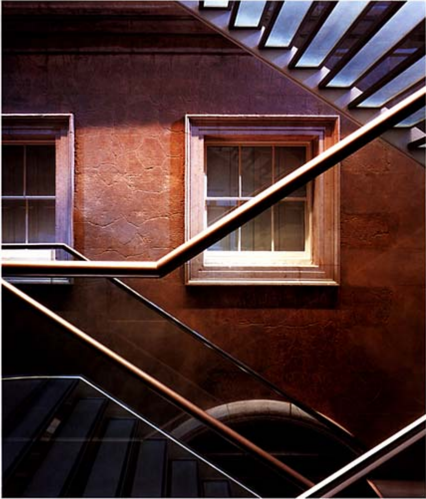
The Sackler Galleries at the Royal Academy of Arts, London, 1985–91: staircase detail
