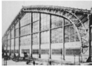
Galerie des Machines, World Fair, Paris, 1889; Contamin and Dutert
