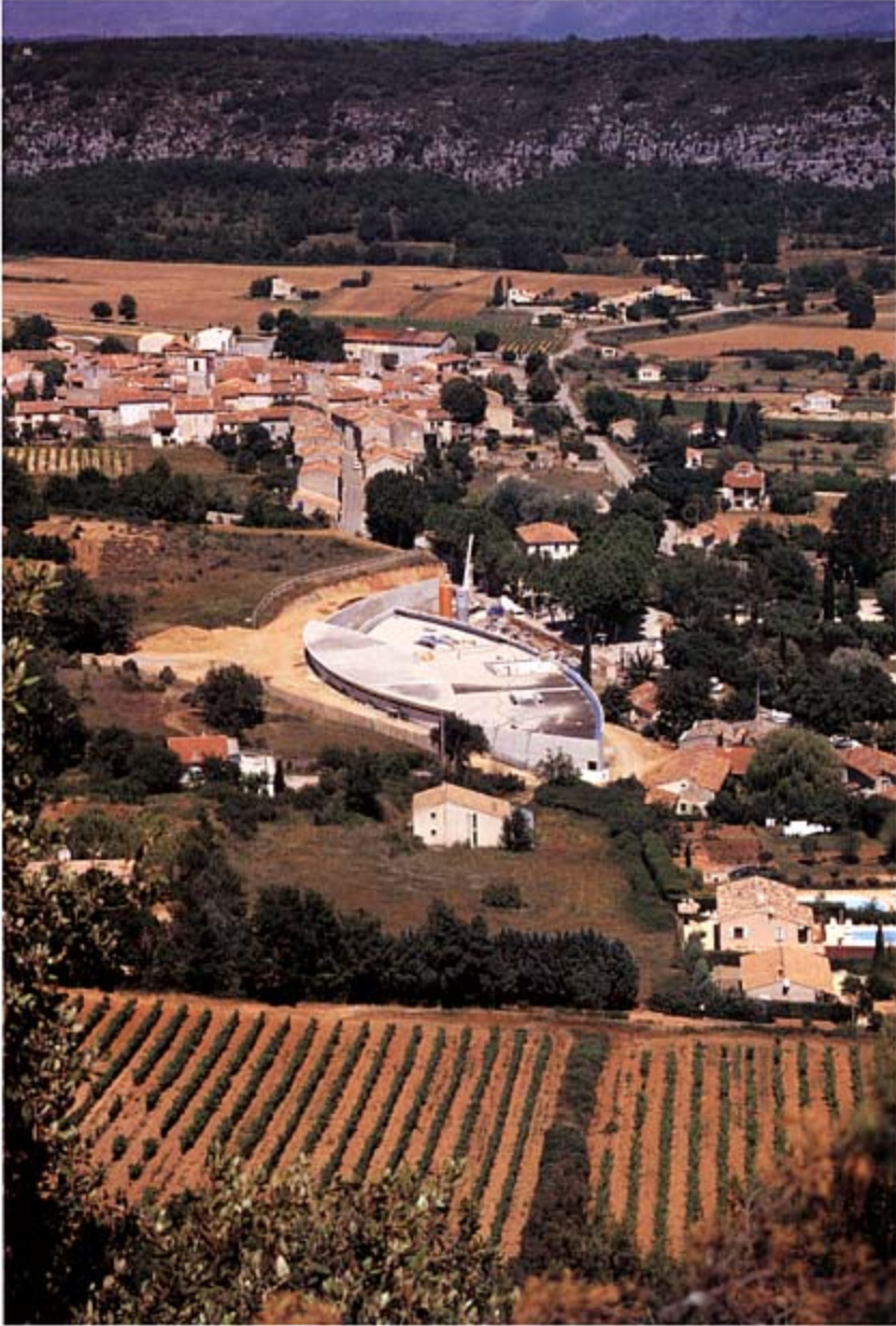
Aerial view of site under construction
