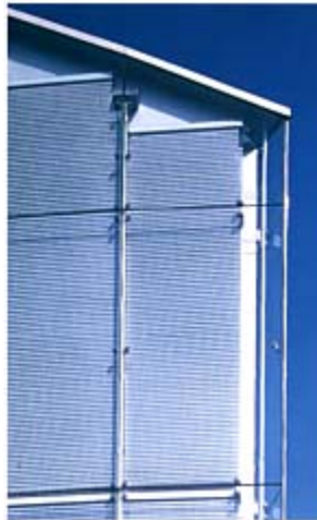
Cladding detail showing the triple-skin wall
