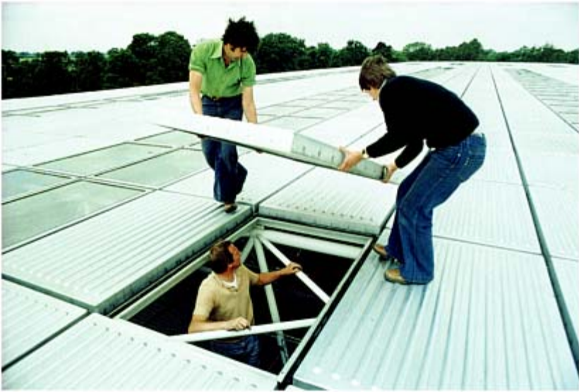
Sainsbury Centre for Visual Arts, UEA, Norwich, 1974–8: interchangeable roof panels
