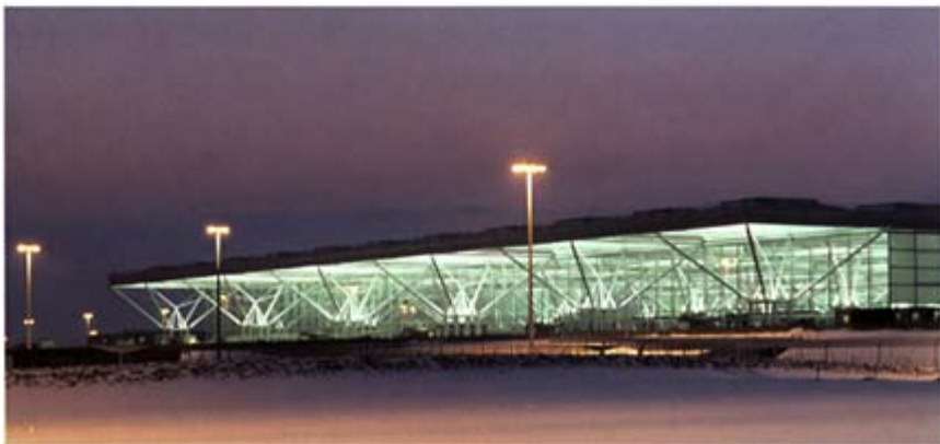
Third London Airport, Stansted, 1981–91: concept sketch by Norman Foster and the terminal at night
