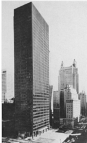
Seagram Building, New York, USA, 1958; Mies van der Rohe and Philip Johnson
