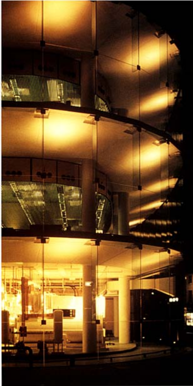
Willis Faber & Dumas Headquarters, 1971–5: night view
