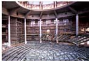
Reichstag, Berlin: the new debating chamber under construction, 1997
