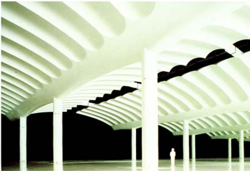
Televisa Headquarters, Mexico City, 1989: pre-cast concrete structure
