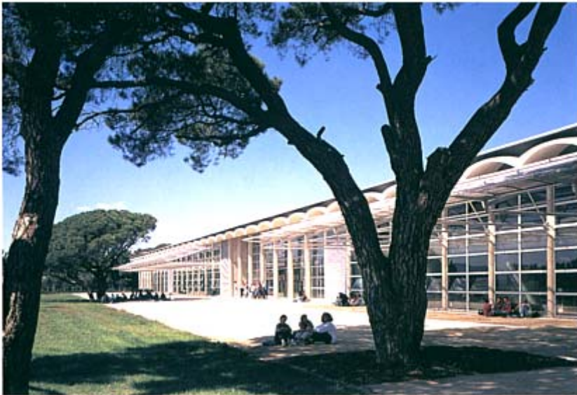
The south-facing facade
