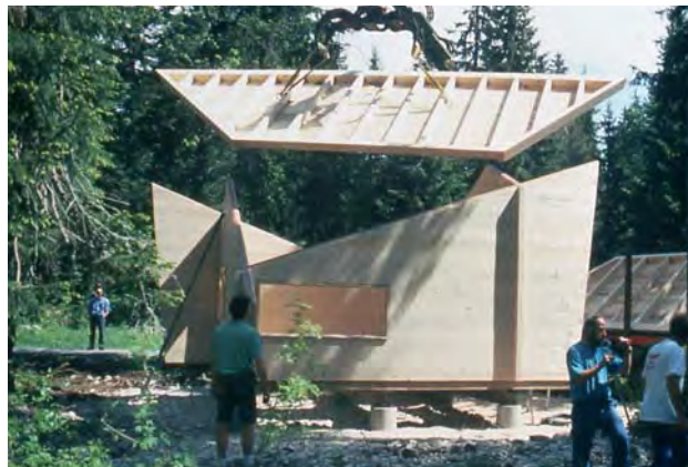
This page, top to bottom: Prototype for a Forest Refuge / diagrams showing how the wall shapes result from their intersection with the pitched roof; views of the assembly process. Opposite: view showing geometry of interior elevation. Following pages: views showing the different geometry of exterior elevations.
