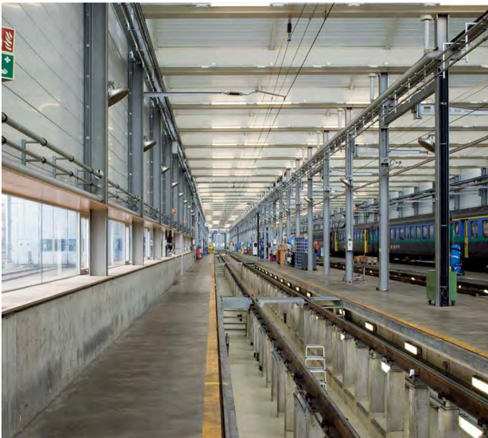
This page: Swiss National Train Maintenance Center / interior views showing maintenance areas beneath the rails. Opposite: interior view and section.
