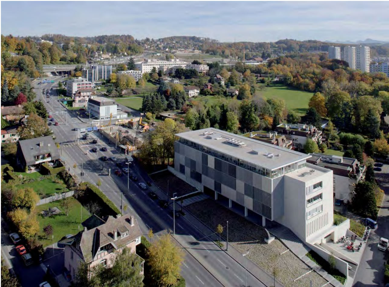
This page: Office Building at Route de Berne 46 / aerial view. Opposite page, top to bottom: plans of attic floor, typical floor, and ground floor. Following pages, clockwise from upper left: entrance portico, main lobby, and view showing how the appearance of the facade varies as occupants adjust the louvered elements to their needs.
