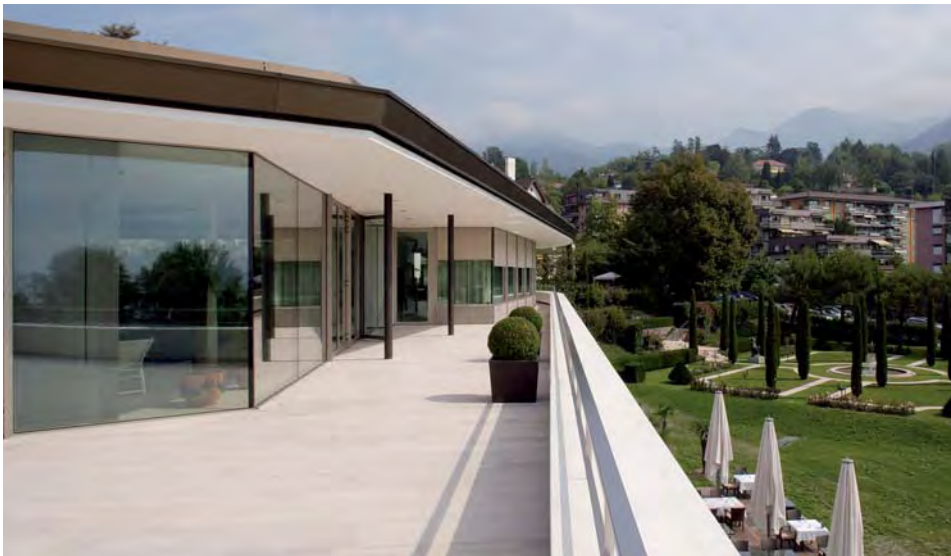
This page: La Prairie Clinic / exterior views. Opposite page, top to bottom: aerial view showing main elevation, and section through swimming pool. Following pages, double spread: general view showing integration of the extension into the terraced site.
