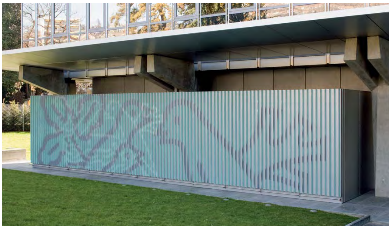
This page: Nestlé Headquarters / view of Company Store facade showing how three different versions of the Nestlé logo shift to produce the optical illusion. Opposite: construction details in plan and section showing how the logo image is broken down and recomposed for this application.
