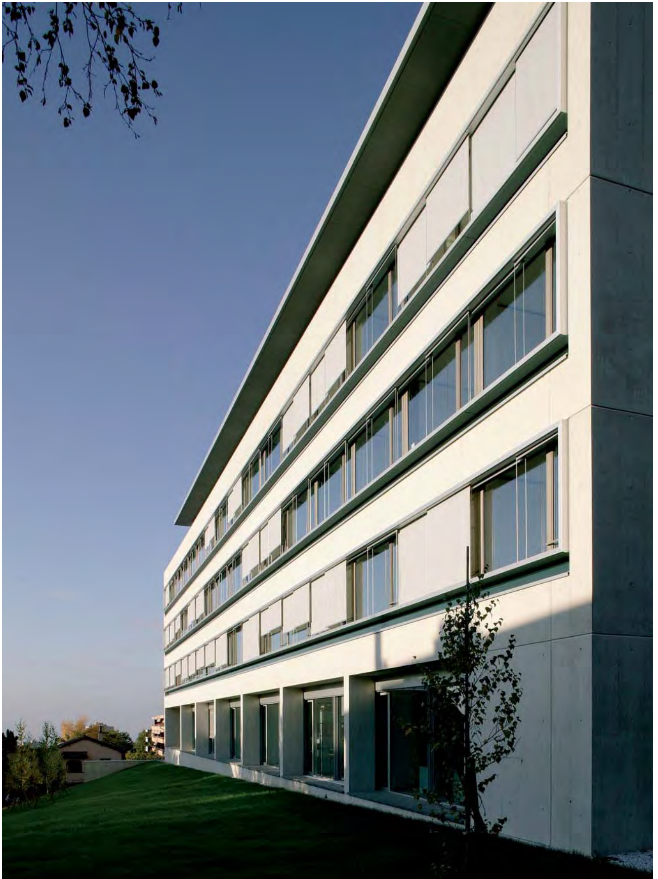
This page: Office Building at Route de Berne 46 / view of concrete facade. Opposite page: construction detail in section and elevation, concrete facade.
