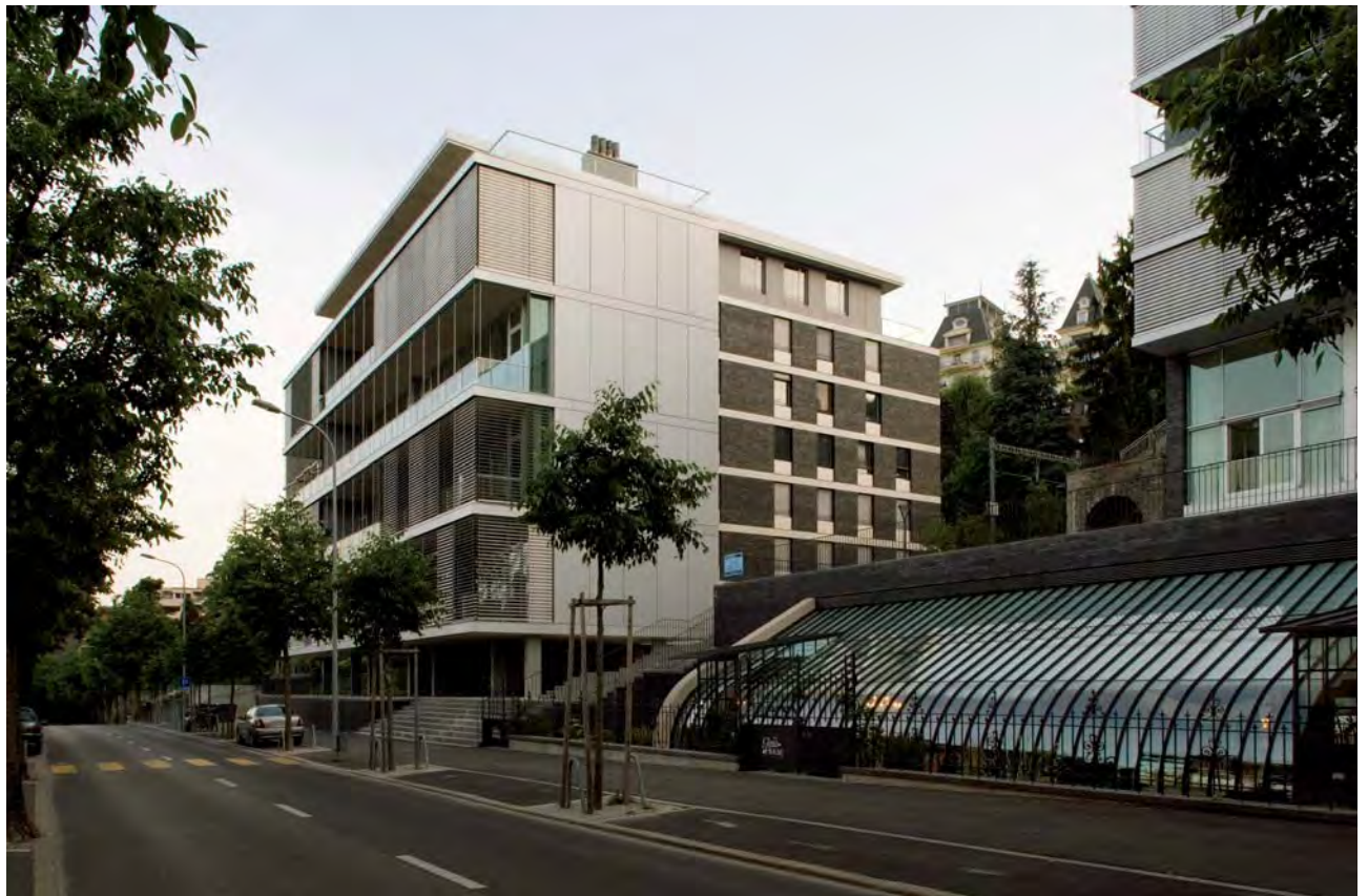
This page, top to bottom: Residential Complex "La Verrière" / construction detail, shade system, and views showing how the facade changes as shades are adjusted to the occupants' needs. Opposite page: detail in section and elevation showing positioning of balcony shade system.
