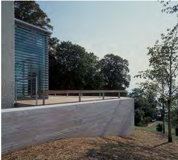
This page, top and bottom: Villa La Falaise / views showing glass-louvered facade. Opposite: construction details in plan and section, glass bays with traditional roll-up solar protection and horizontal glass louvers.
