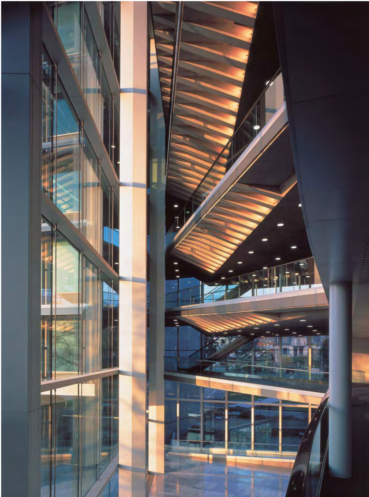
This page: Nestlé Headquarters / Richter & Dahl Rocha's Liaison Space. Opposite, clockwise from upper left: scheme for ramp distribution, plan of sixth floor, and section.
