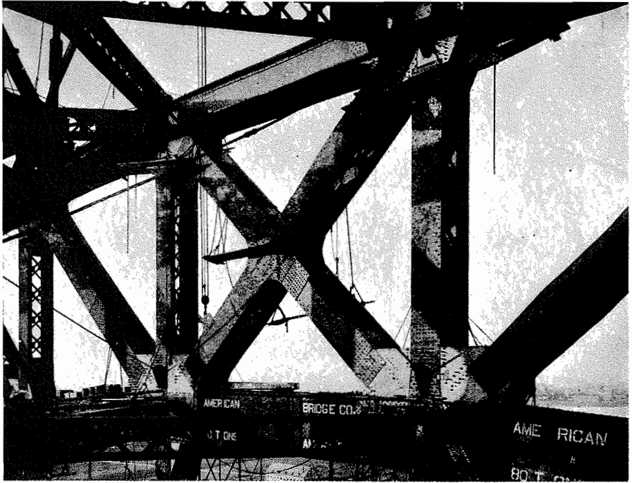
STEEL CONSTRUCTION. THE STEEL CORPORATION
