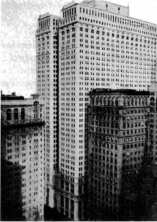
THE EQUITABLE BUILDING, NEW YORK
